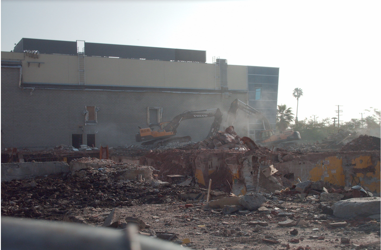
Deluxe Film Laboratories' 3-story film processing facility, shown in January of 2015 being gutted to convert it into an office building.
