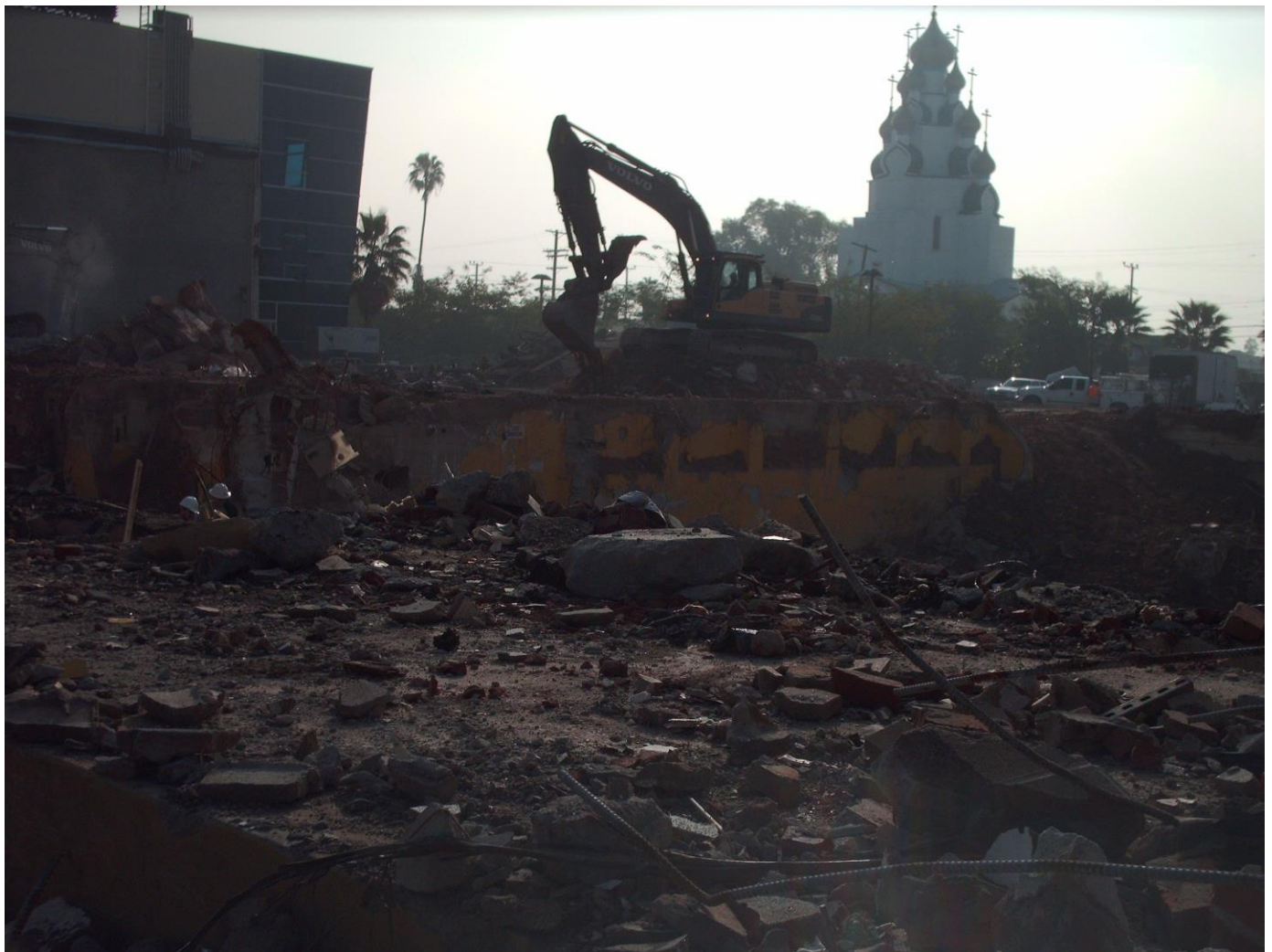
Photo above: Site demolition in 2015. Note gutted film processing building at left.
