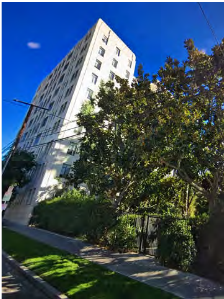
Franklin Ave. front entrance of The Montecito and Landscaped Garden Park with 27 trees. Residents facing west overlook the beautiful gardens and park.
