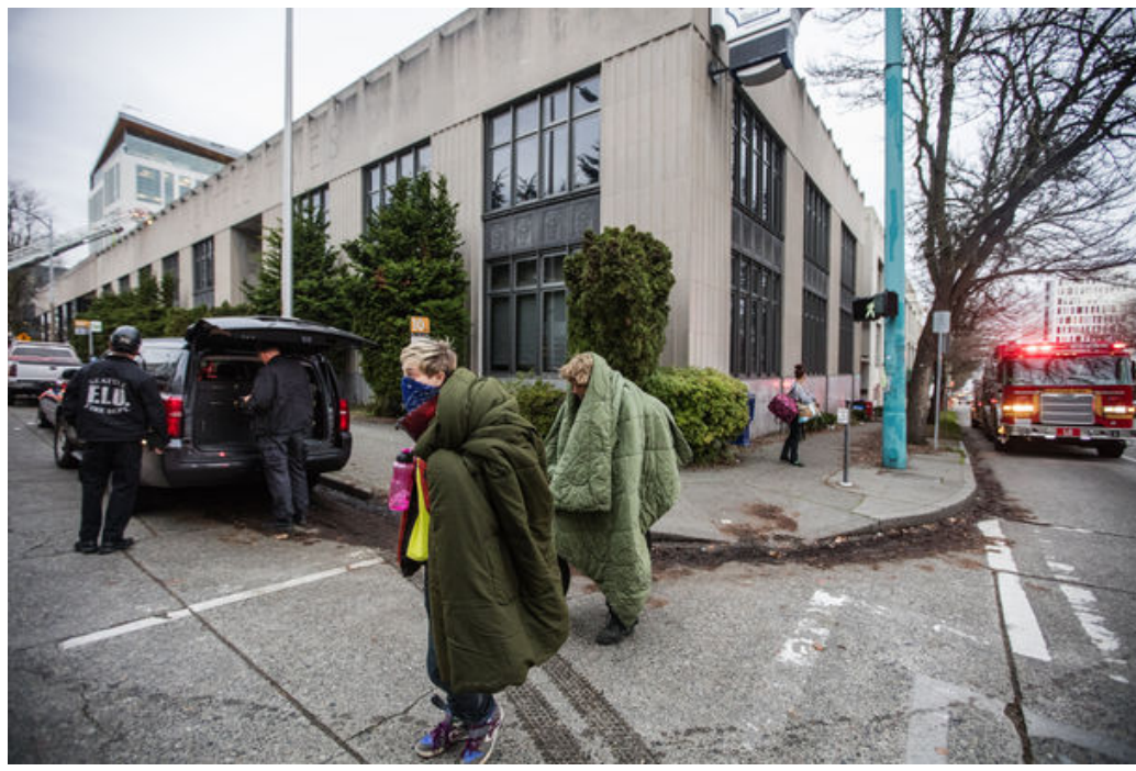
November 2015: "Squatters leave the old Seattle Times building at 1120 John St., after waking up during Thursday's fire" (Steve Ringman / Seattle Times)
