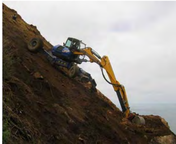
Specialized Hillside Excavator
