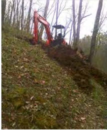
Specialized Hillside Excavator
