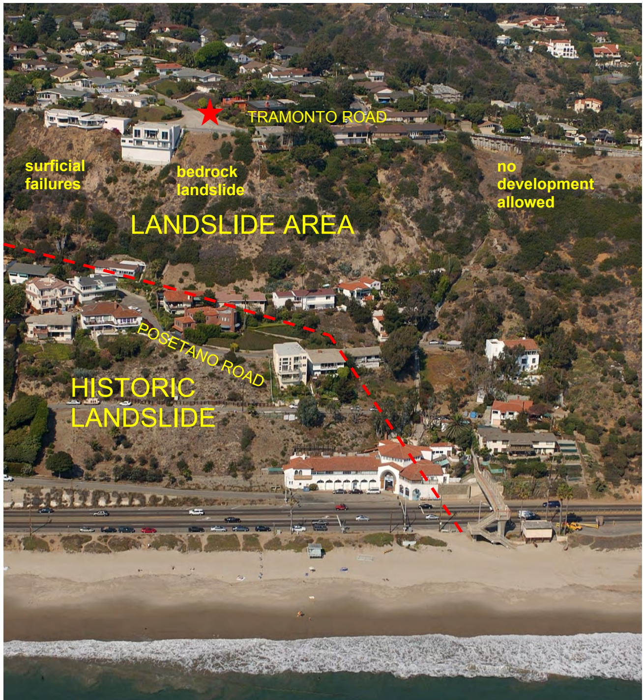
Helicopter view of project area with landslide areas noted
