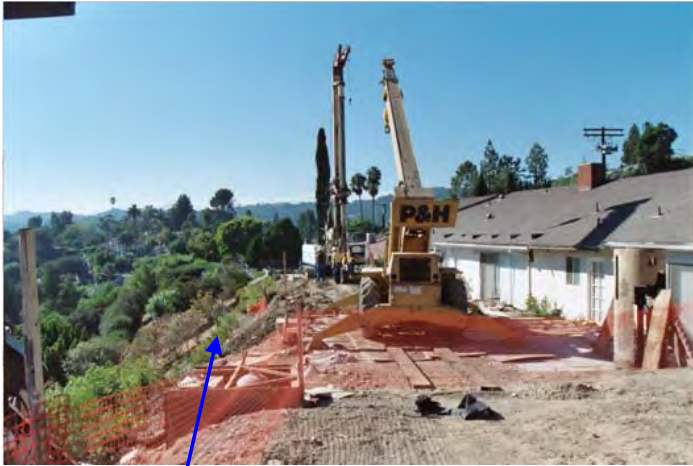
Grading at Top of Slope
