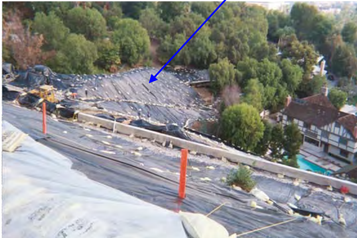
Plastic for Slope Erosion Protection
