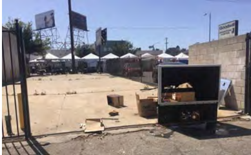
The site in June during South Robertson's SORO Fest due to the owner's failure to repair the fence after a car crash in February 2018.
