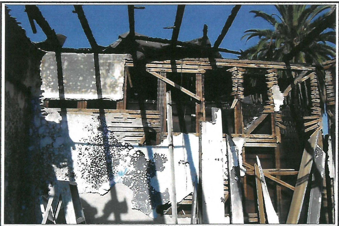
04). VIEW LOOKING NORTH FROM 2 ND STORY NORTHEAST BAY BEDROOM
