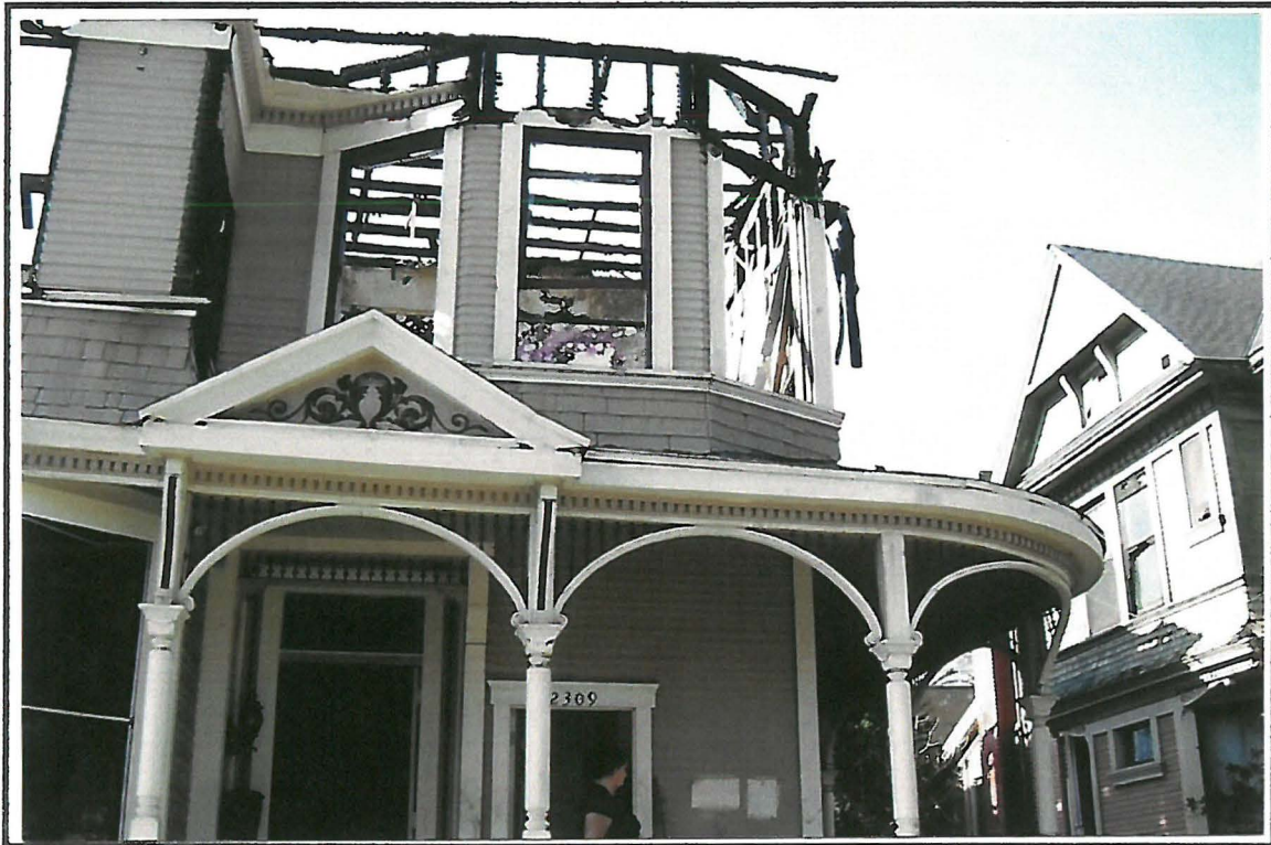
03). VIEW OF 2 ND STORY NORTHEAST BAY
