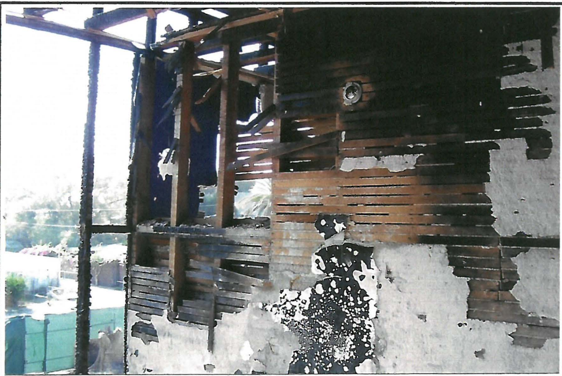
14). VIEW LOOKING SOUTHWEST FROM 2 ND STORY SIDE BEDROOM
