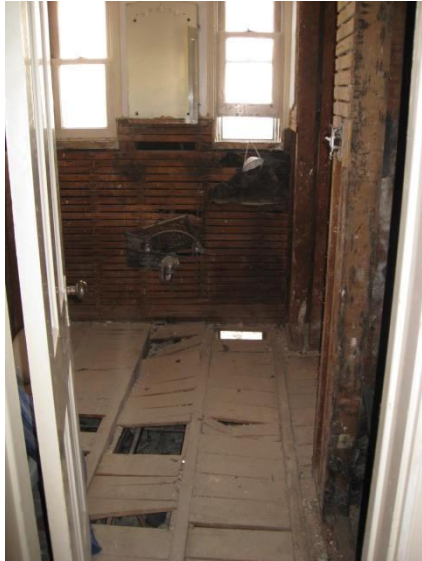
Figure 7. Bathroom renovation, lower front unit (134 ½ Kings Road), 2010.
