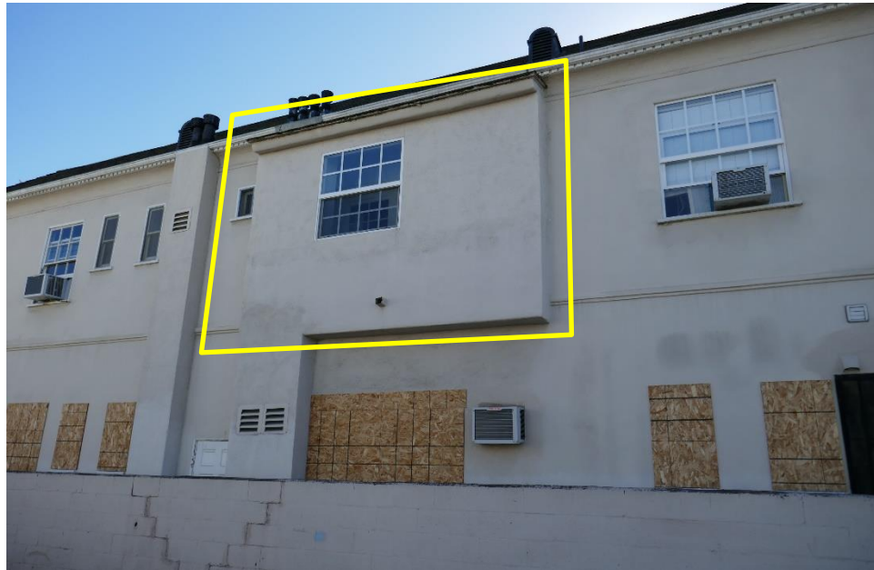
Figure 5. Detail of enclosed balcony on north façade.
