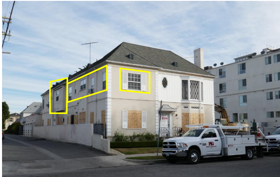
Figure 1. Front (west) façade and north side façade (at left) of 132 N. Kings Road, looking southeast. In yellow are altered areas, like vinyl windows and the enclosed balcony on the north façade (left).
