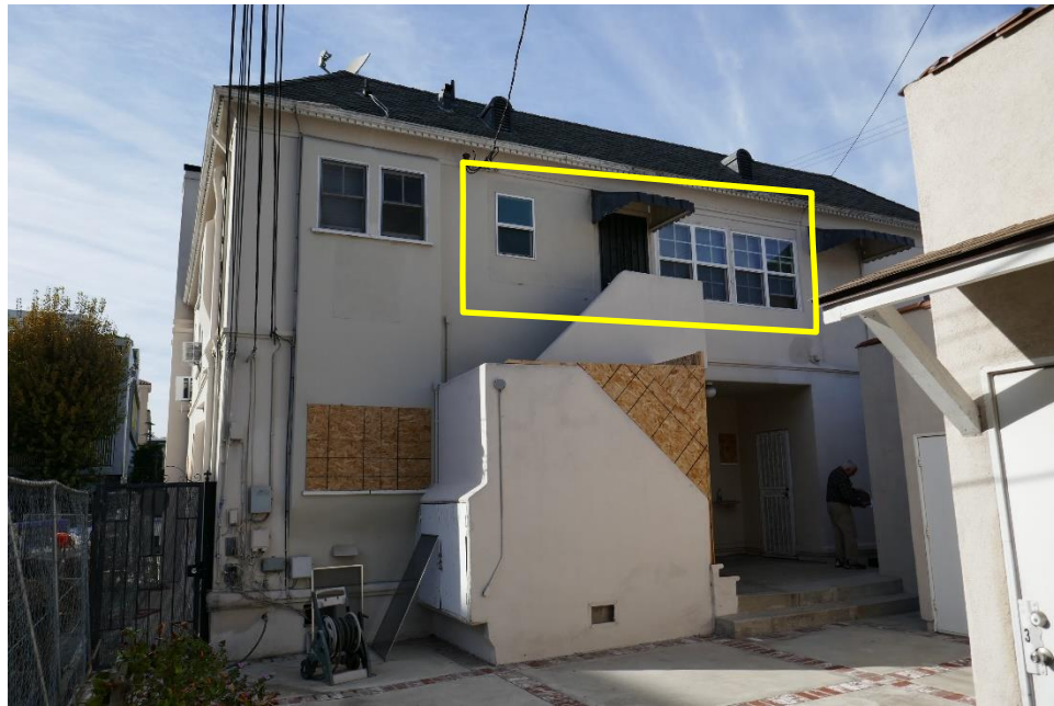
Figure 3. Rear (east) façade with area of previous balcony highlighted, looking west.
