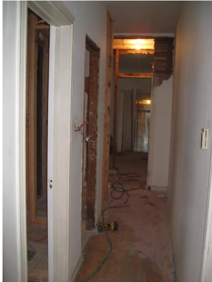
Figure 11. Hallway in lower front unit, with new bathroom door at left front and original bathroom door at left center. In the background is the doorway to the rear bedroom during construction, 2010.
