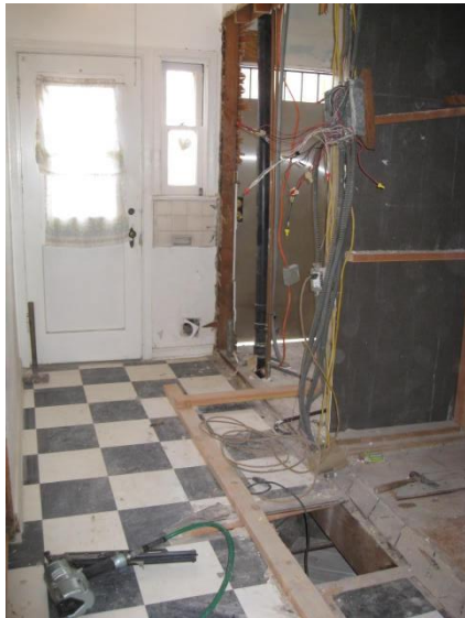
Figure 9. Converting closet and laundry area into new bathroom in lower front unit, 2010.
