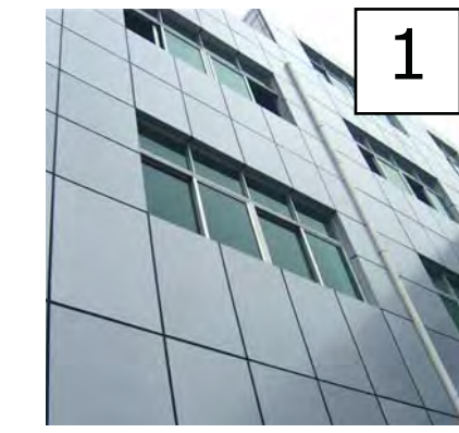
1 EXTERIOR METAL CLADDING
