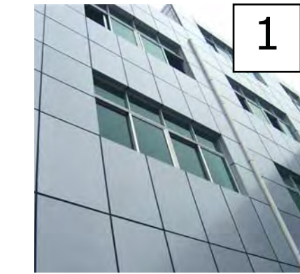
1 EXTERIOR METAL CLADDING
