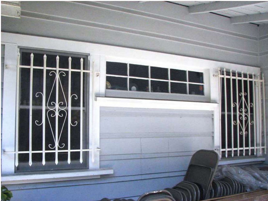
Burchel Duplex, living room windows, 1130-32 N. Beachwood Drive, May 11, 2007 (Charles J. Fisher photo)
