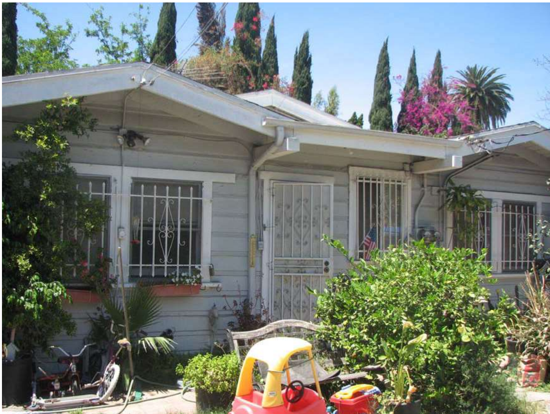
Burchel Duplex, rear facade, 1130-32 N. Beachwood Drive, May 11, 2007 (Charles J. Fisher photo)
