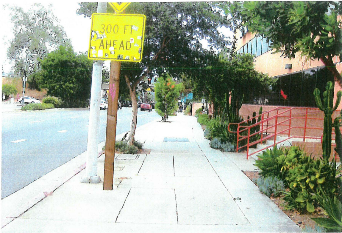
3. South View along 4631 Laurel Cny. Blvd. Sidewalk widths (including curb) along the west side of Laurel Cyn. Blvd. are typically 9'-8" to 12'.
