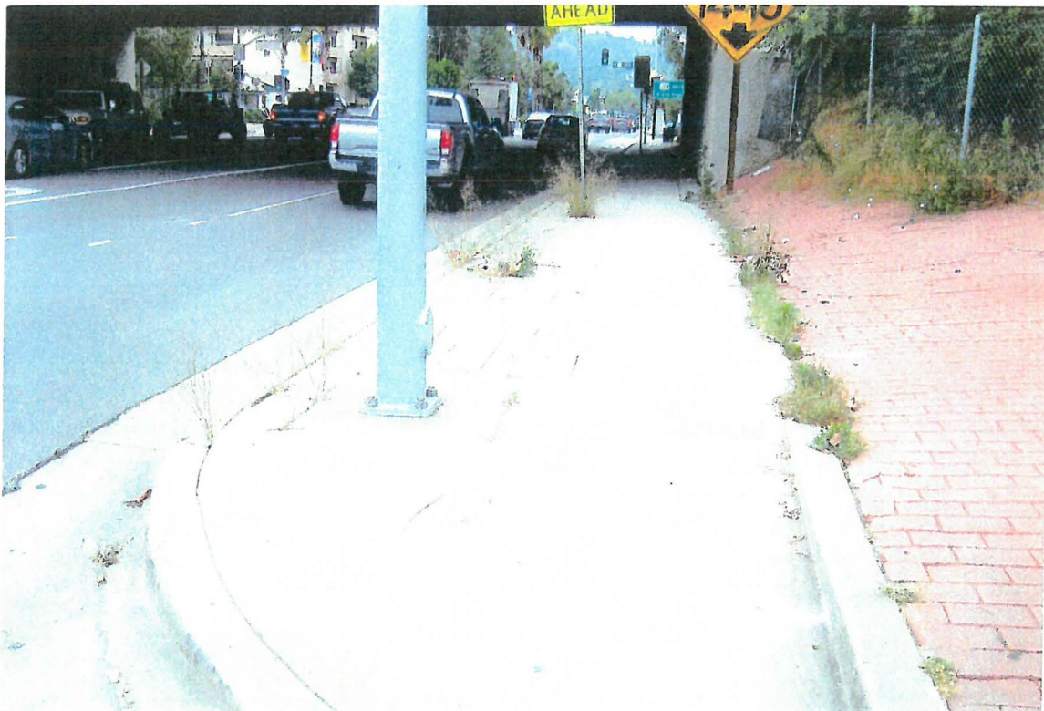
4. View to south from freeway on-ramp. Note sidewalk under freeway is 8'-4".
