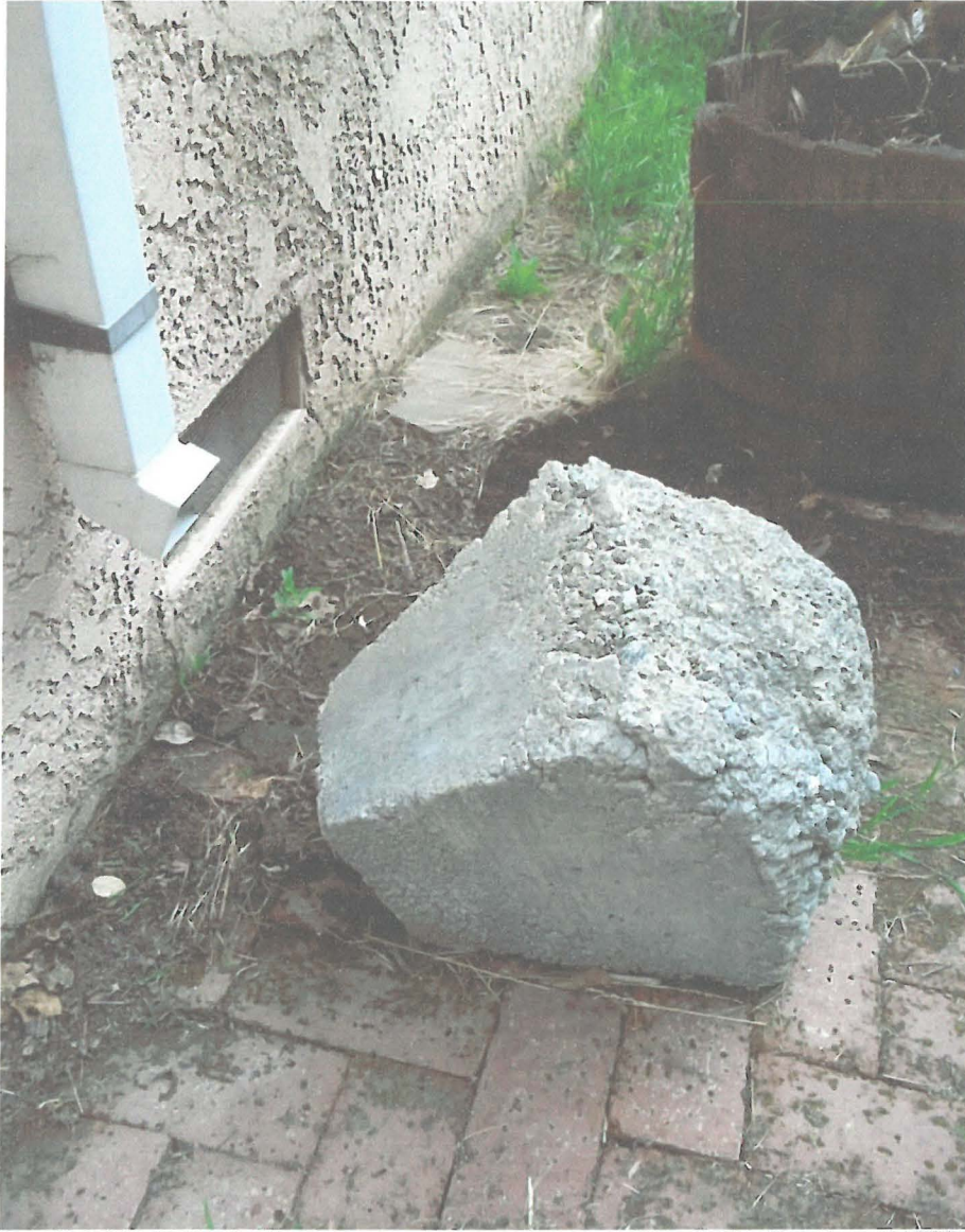
E-2 Landslide of 2001-2002. This landslide began in RHC drainage and wiped out the deck at 4653 San Andreas Avenue. Remains of the deck foundation block are still located to the west of 805 Cynthia Avenue.
