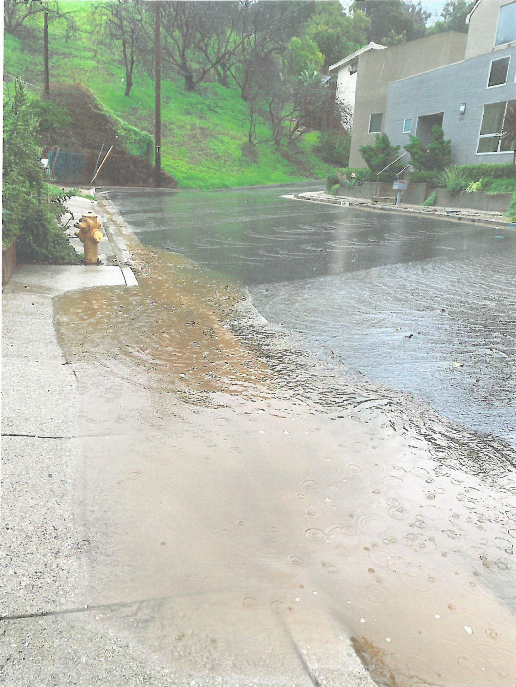
G-1 February 14, 2019. Water runoff from RHC to 830 Cynthia Avenue, consisting of silt up to mid sidewalk.
