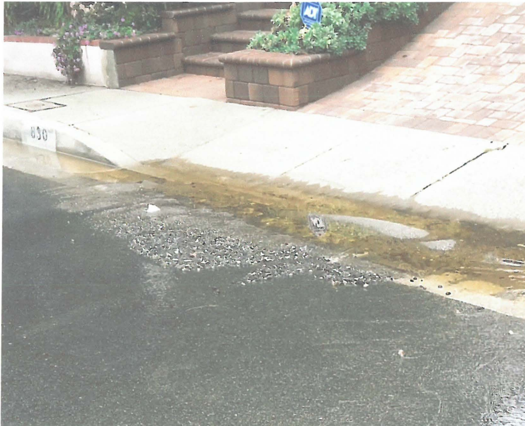
G-2 February 3, 2019. Gravel and silt runoff from RHC to 830 Cynthia Avenue.
