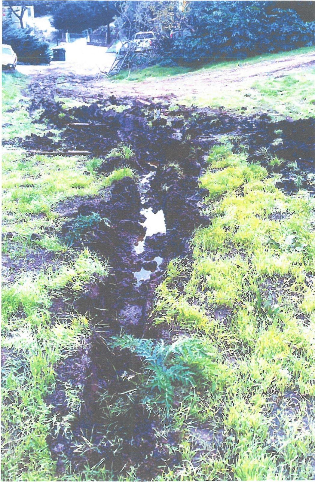
H-2 Attempts to drain the seasonal stream, causing debris flow onto Cynthia Avenue.
