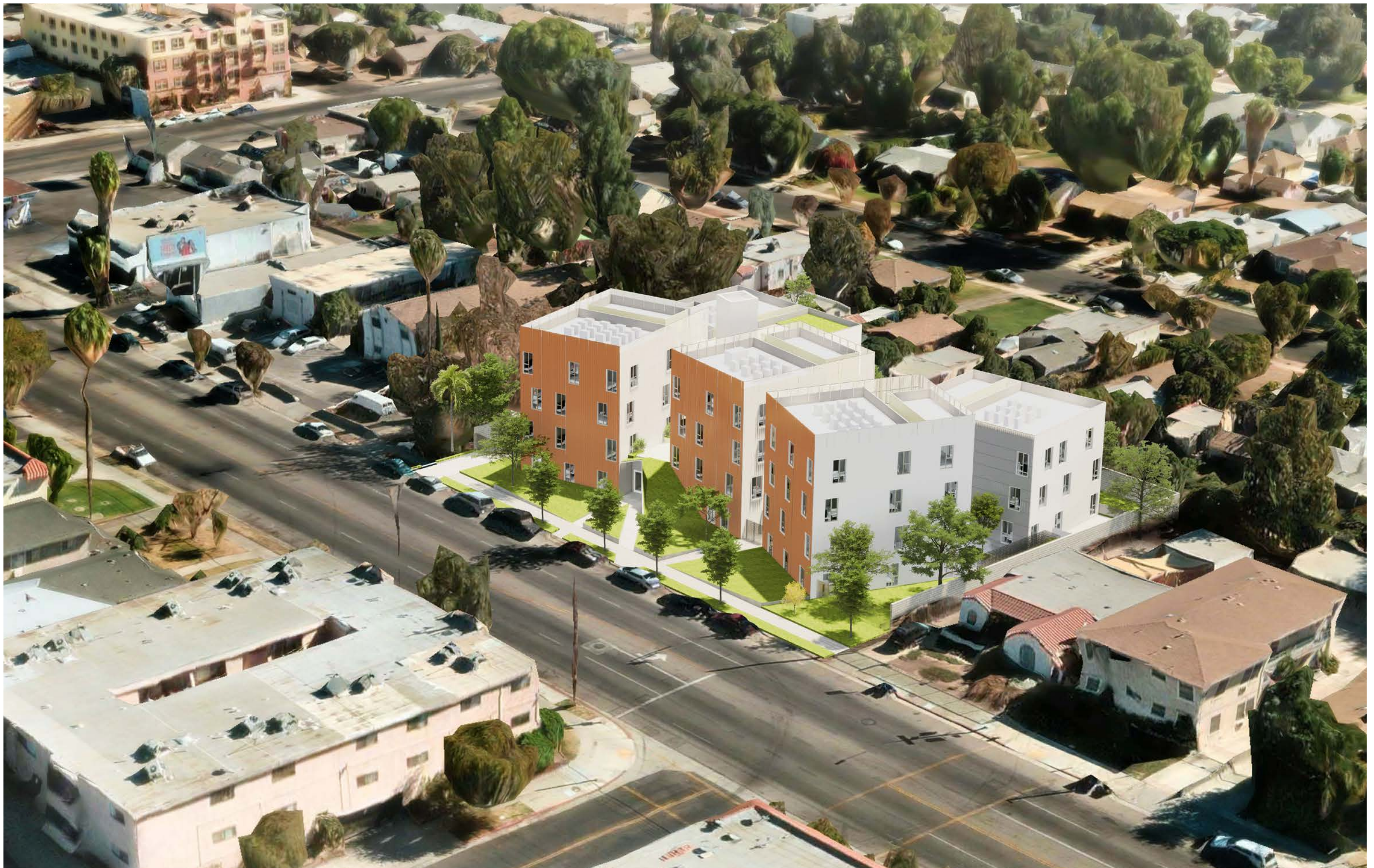
AERIAL VIEW FROM NORTHWEST
