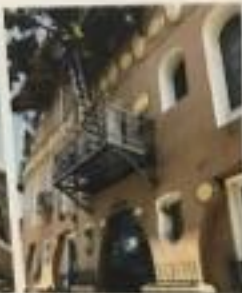
③ METAL RAILING BUSHES GREENING
