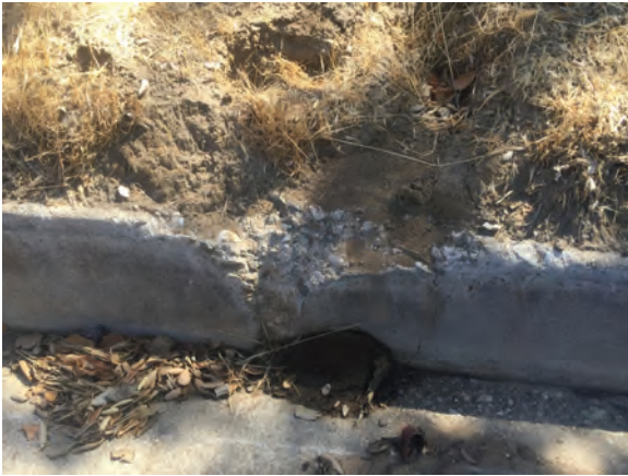
Impact damage from unreported collisions with curb and retaining wall at site of proposed new street entrance.
