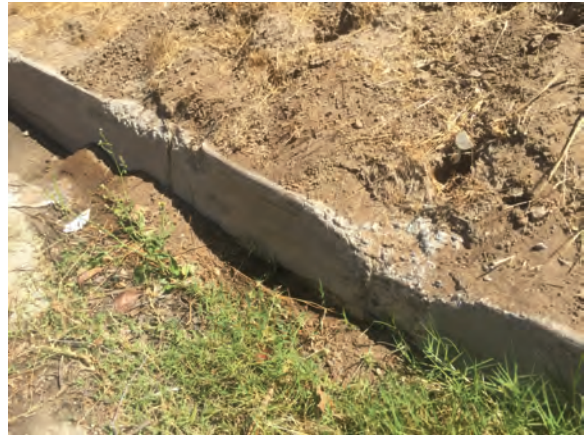
Impact damage from unreported collisions with curb and retaining wall at site of proposed new street entrance.
