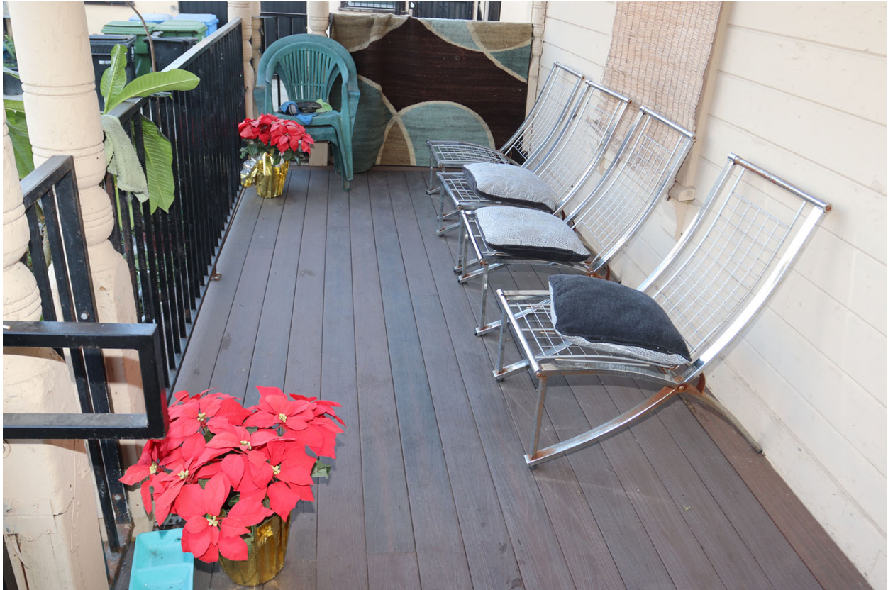
Changed of Wood in Porch area
