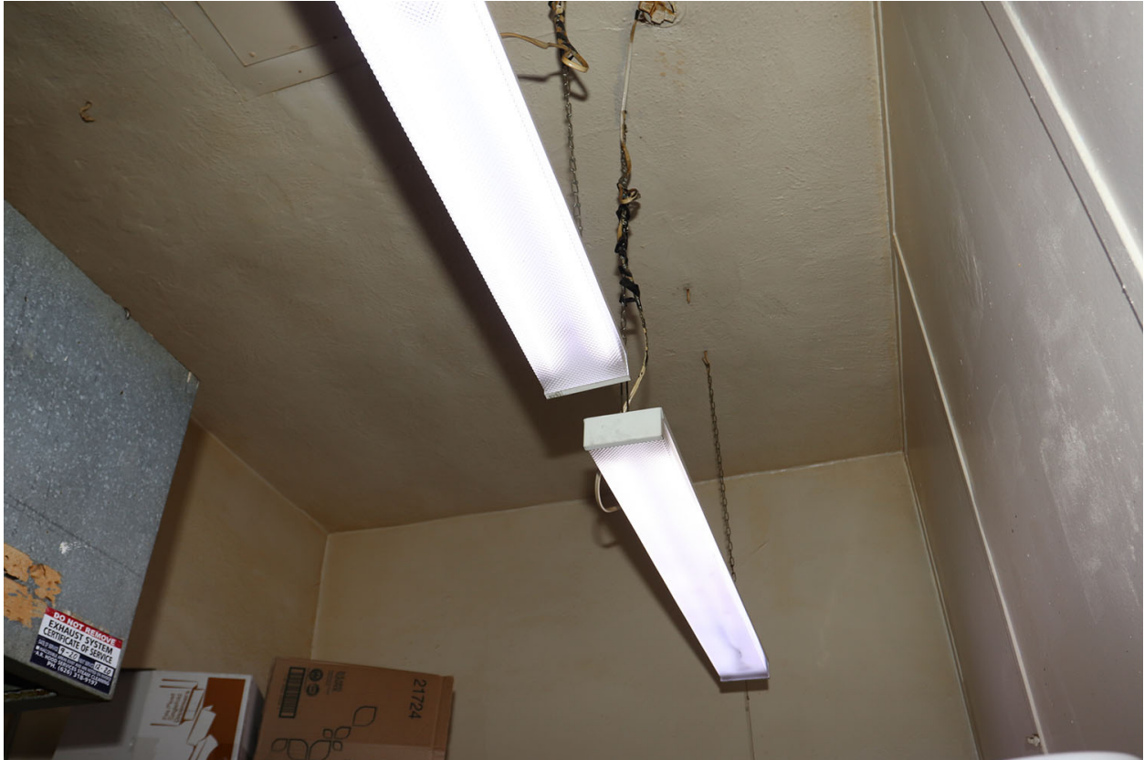
Changed Light fixtures in the kitchen
