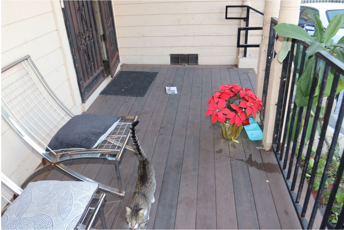
Added Metal door to main entrance
