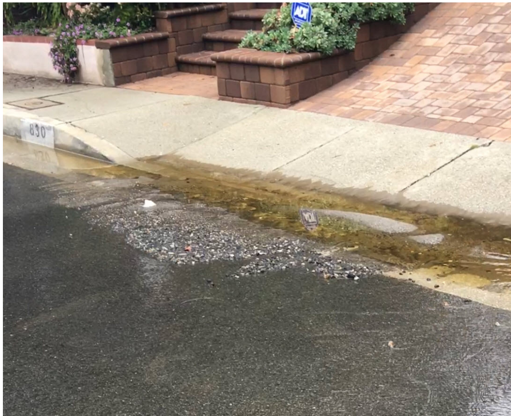
Photo 8: Debris Flow in front of 830 Cynthia Ave. north and downstream from RHC
