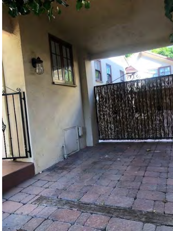
Figure 10A. Eastern Façade (view facing northwest), 14535 Killion Street SOURCE: Sapphos Environmental, Inc., 2019
