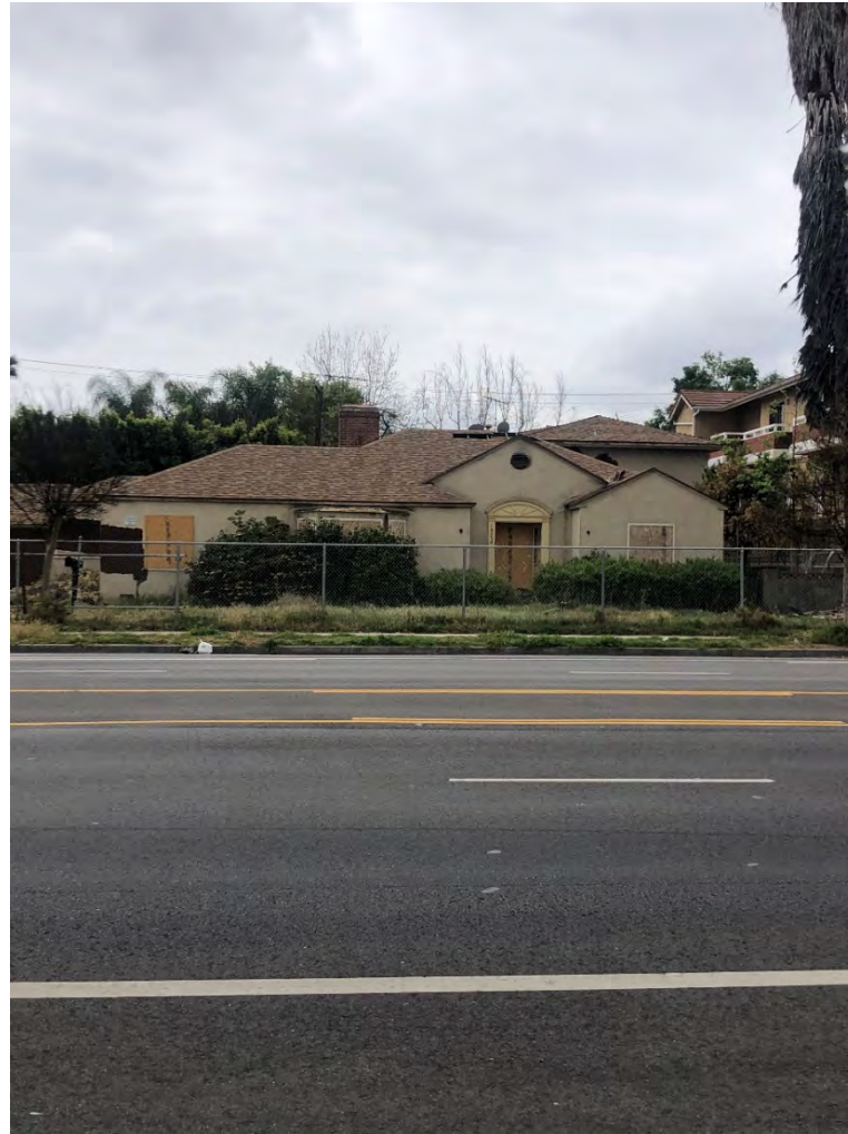
Figure 13. South Side of Burbank Boulevard (view south) SOURCE: Sapphos Environmental, Inc., 2021
