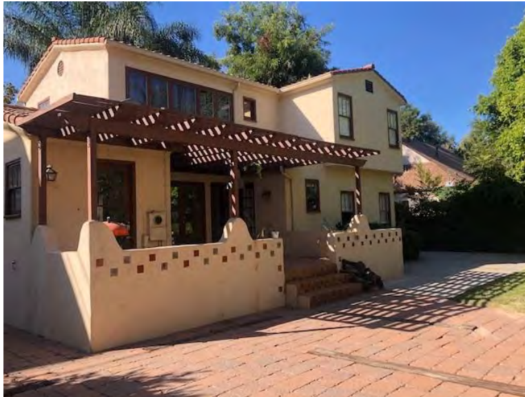
Northern Façade (view facing southwest)
