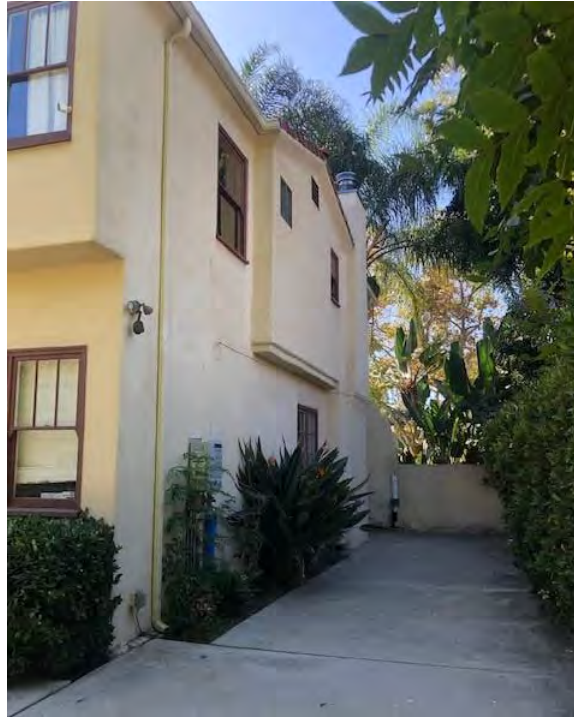
Western Façade (view facing southeast)
