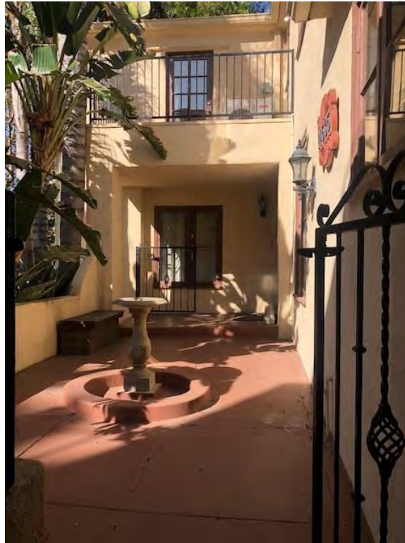
Figure 9. Entrance Detail (view facing east), 14535 Killion Street
