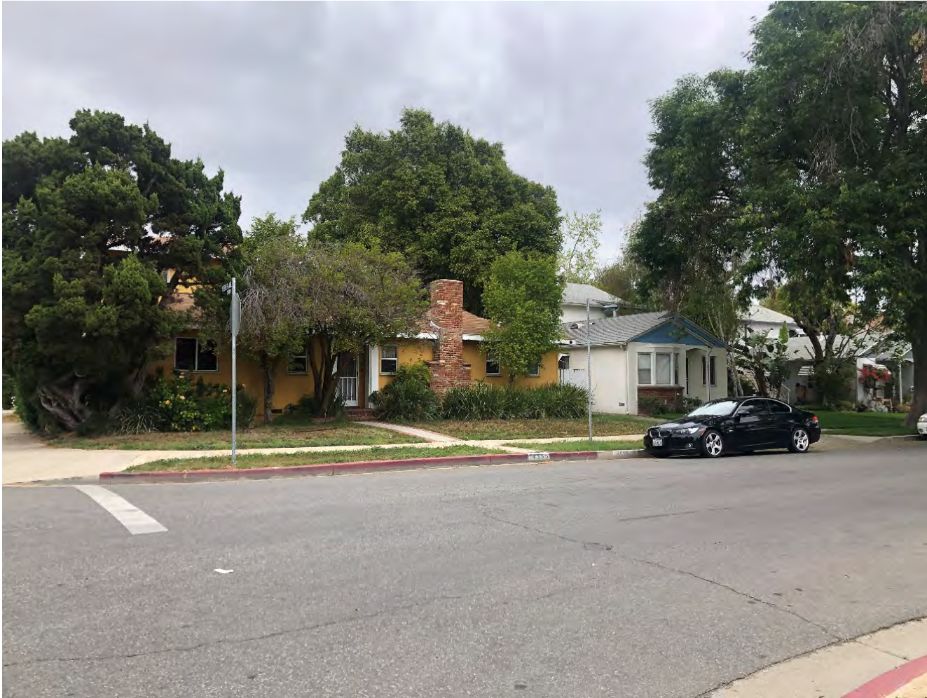
Figure 5. North Side of Killion Street (view northeast) SOURCE: Sapphos Environmental, Inc. , 2021
