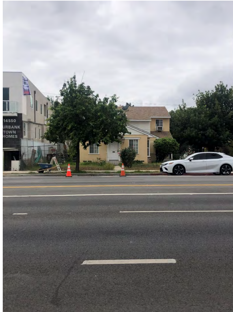
Figure 16. South Side of Burbank Boulevard (view south) SOURCE: Sapphos Environmental, Inc., 2021
