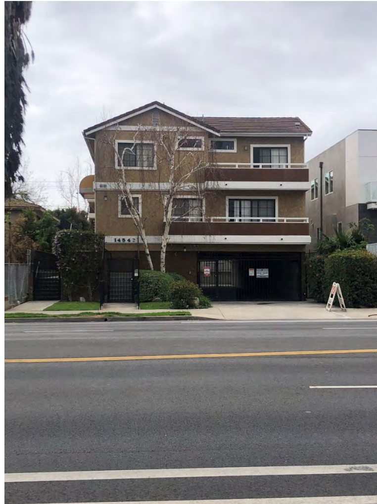
Figure 14. South Side of Burbank Boulevard (view south) SOURCE: Sapphos Environmental, Inc. , 2021
