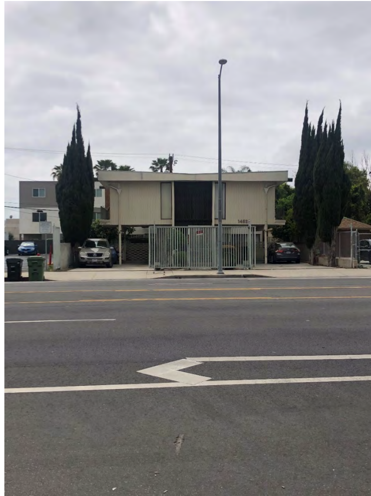
Figure 12. South Side of Burbank Boulevard (view south) SOURCE: Sapphos Environmental, Inc., 2021
