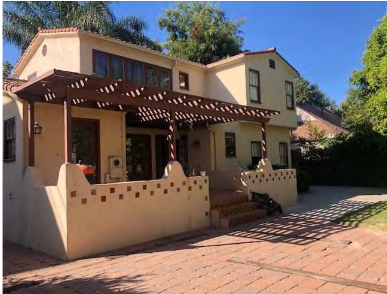
Figure 11. Northern Façade (view facing southwest), 14535 Killion Street SOURCE: Sapphos Environmental, Inc., 2019
