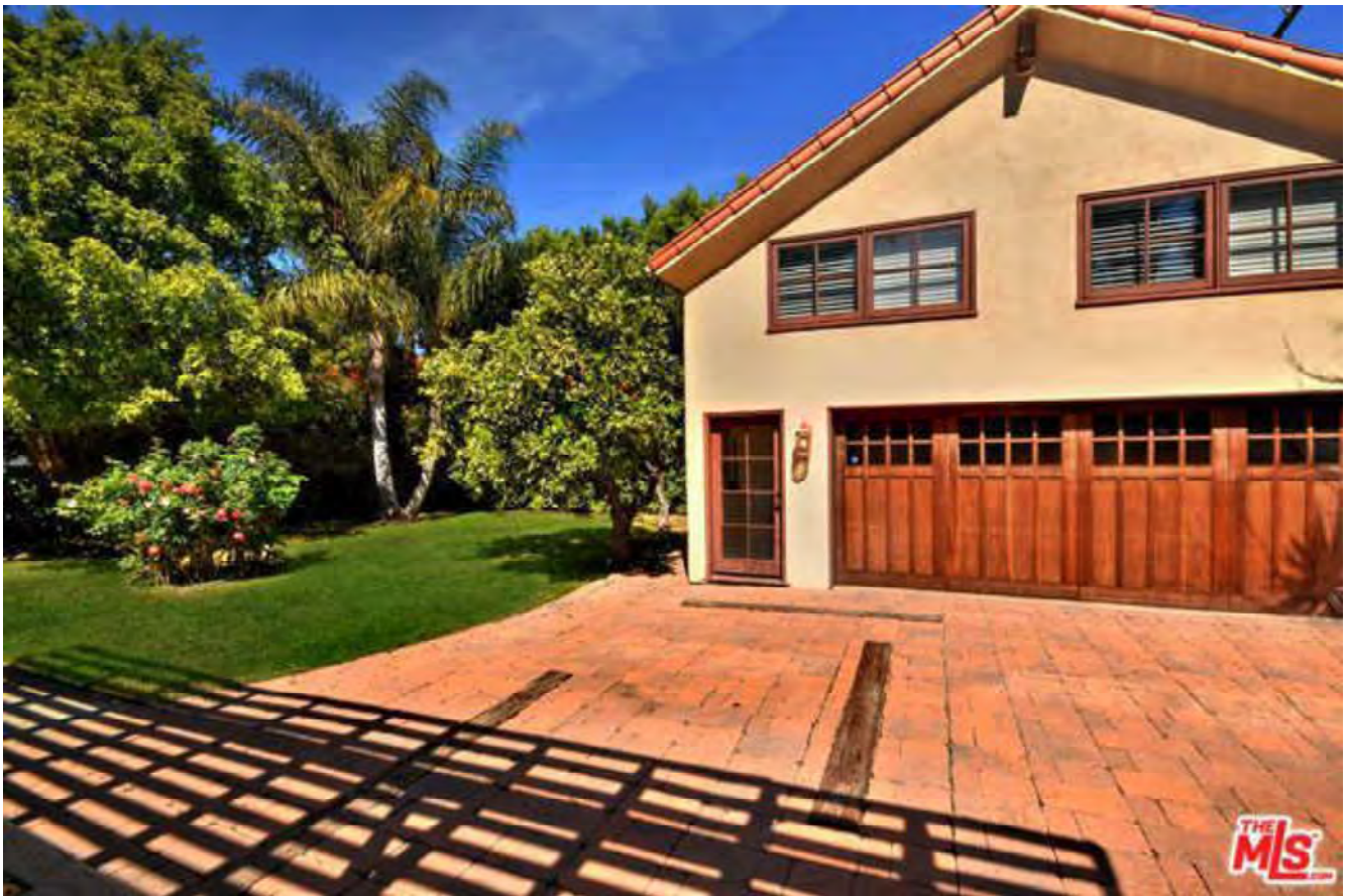
Hatterscheid Residence, new garage, 14535 Killian Street, April 5, 2018 (Multiple Listing Service Photograph)
