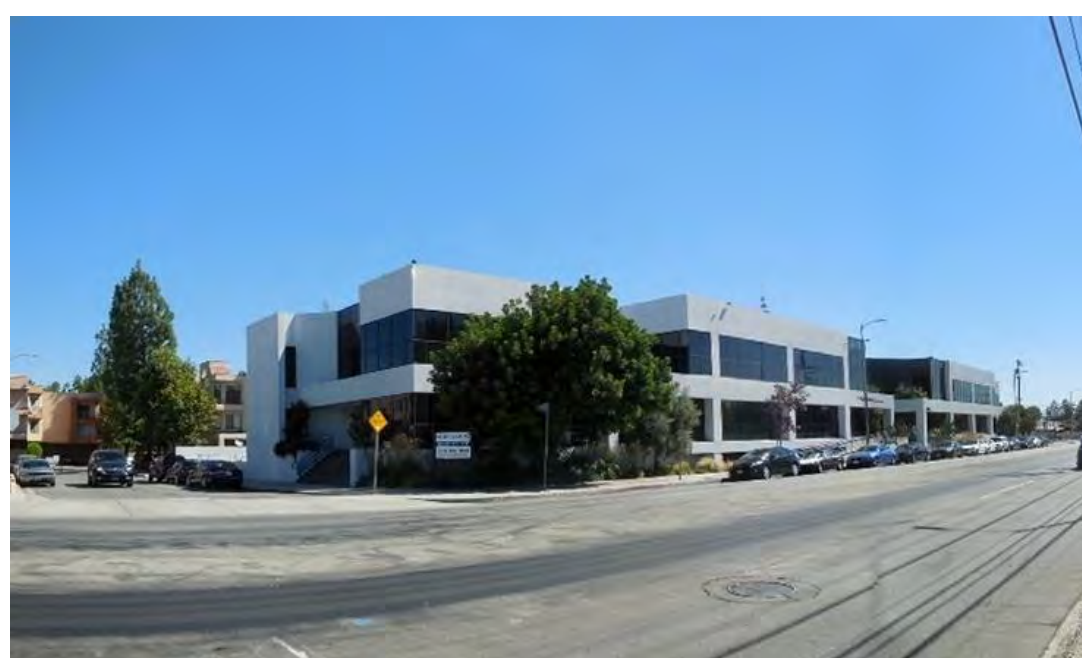
Looking northeast across Vanowen Street toward the west and south (front) sides of the subject property
