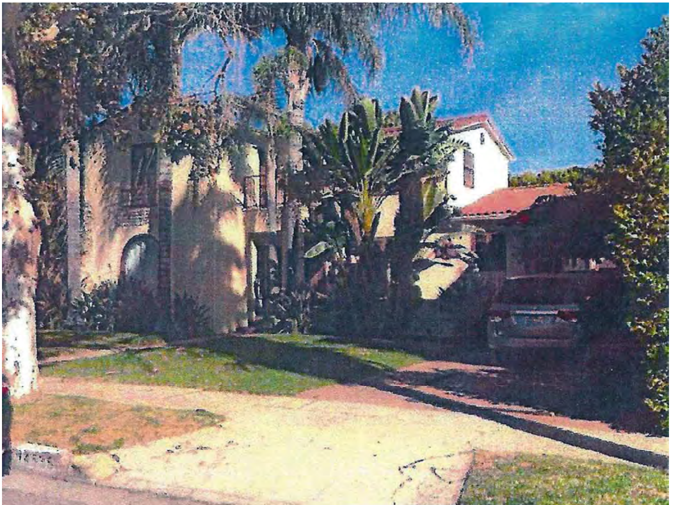
Hatterscheid Residence, Southeast corner, 14535 Killian Street, October 1, 2019 (Photograph by Sappros Environmental)
