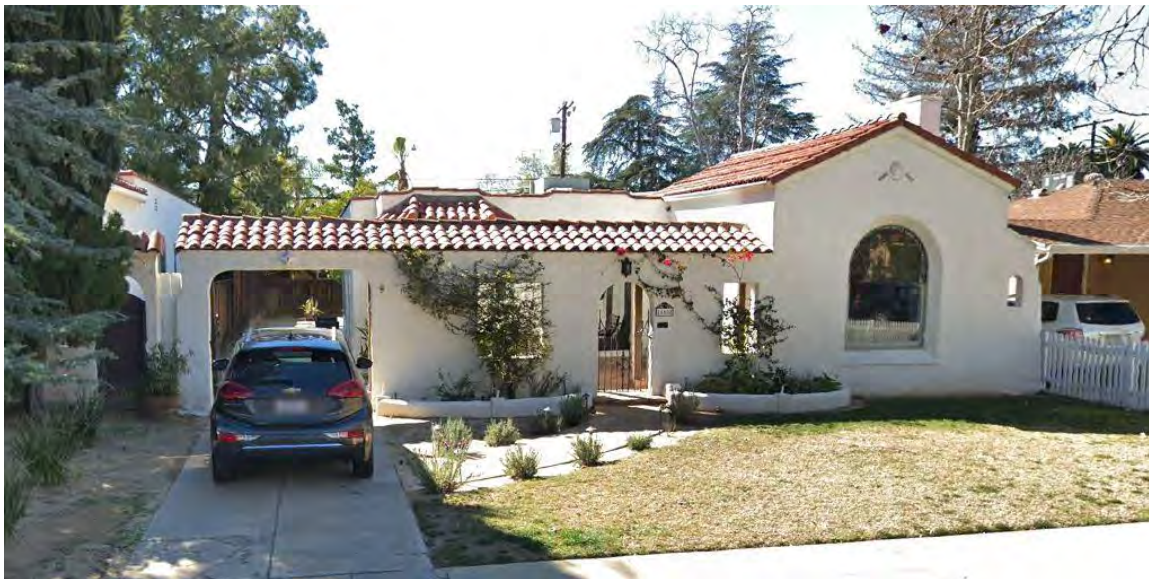
Figure 15. 14608 Killion Street SOURCE: Google Earth, 2019
