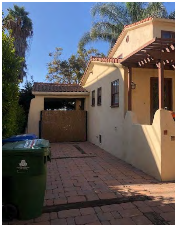
Eastern Façade (view facing southwest)
