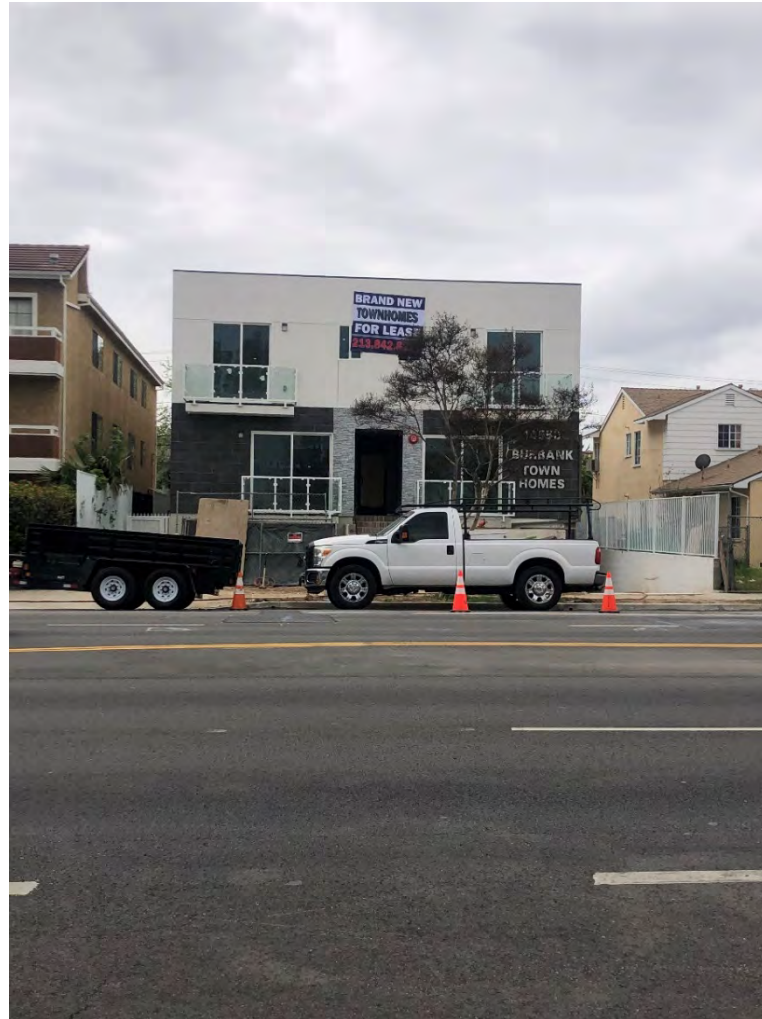
Figure 15. South Side of Burbank Boulevard (view south) SOURCE: Sapphos Environmental, Inc. , 2021
