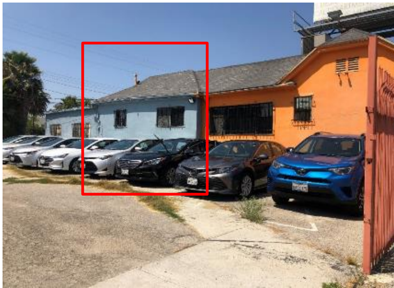
Figure 3. Southwest Façade Showing Rear Addition SOURCE: Sapphos Environmental, Inc., 2020
