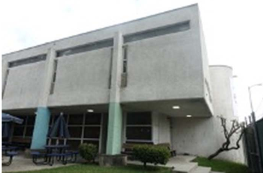
Figure 3. The symbolic vertical windows. The vertical sash was removed, and the bottom portion filled, which is an indication of adaptation over time.
