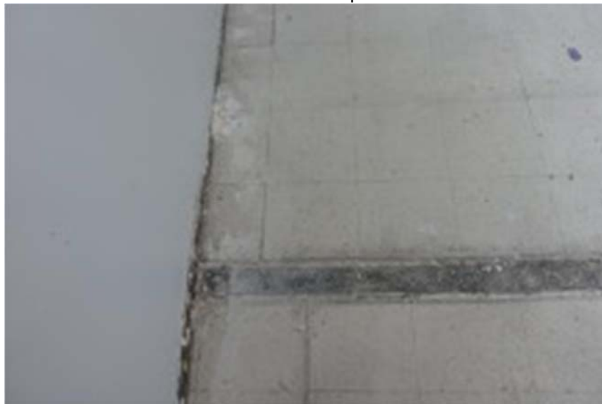
Figure 4. The exposed dark trace in the floor indicates that a partition was removed and the floor plan was changed. It is a non-reversible alteration and an indication of adaptation over time.
