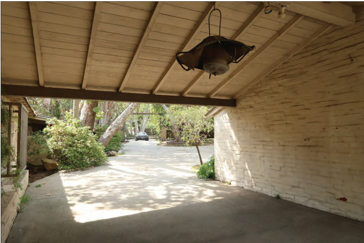
Image 6: Original entry breezeway, view northwest (Chattel, 2021)
