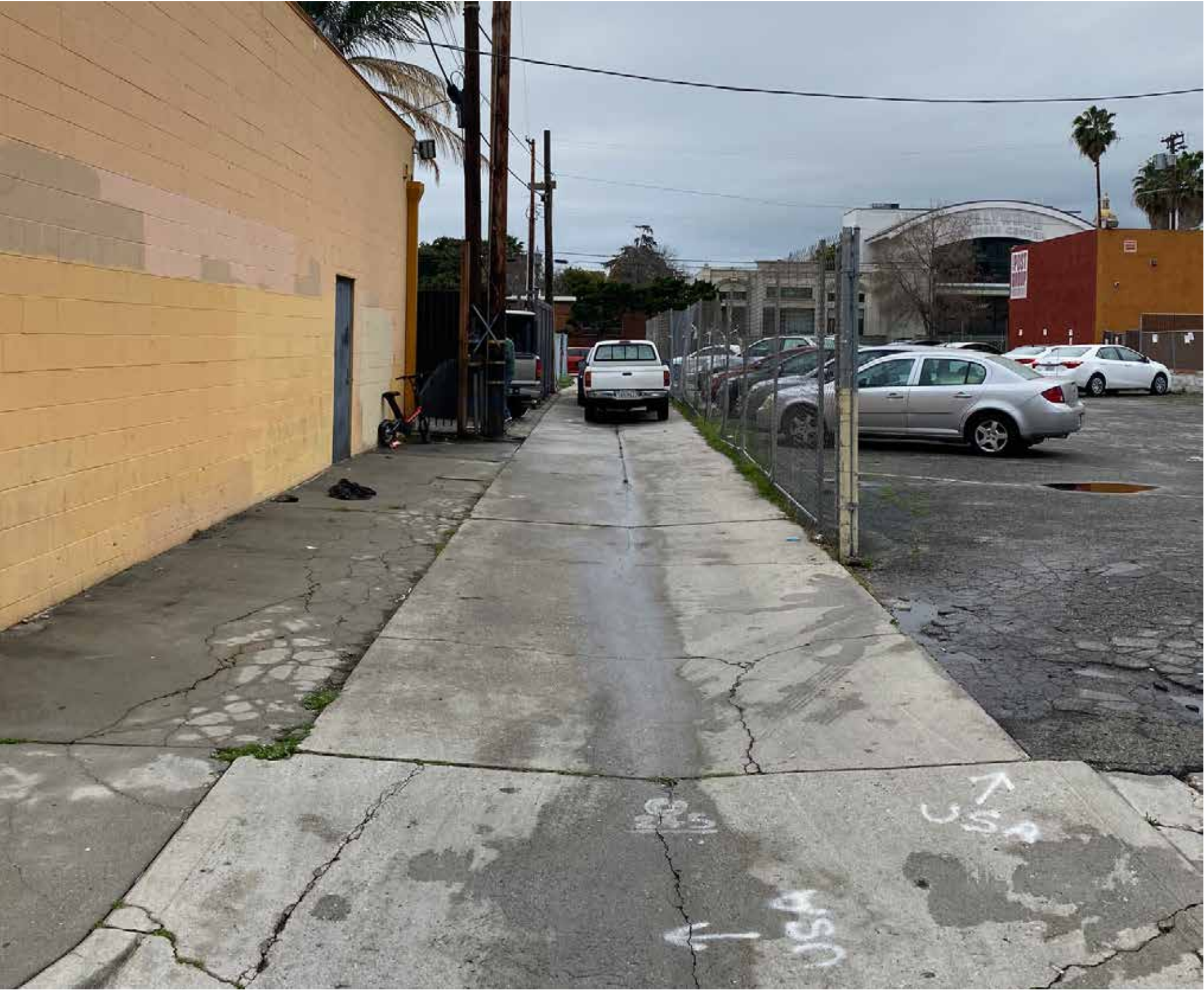
3 VIEW WEST ON WILCOX AT ALLEY
