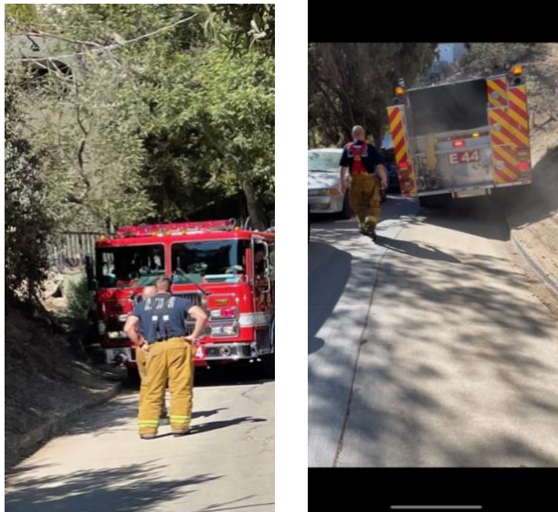
Photos of Fire Trucks attempting to reach gas leak caused by construction.
