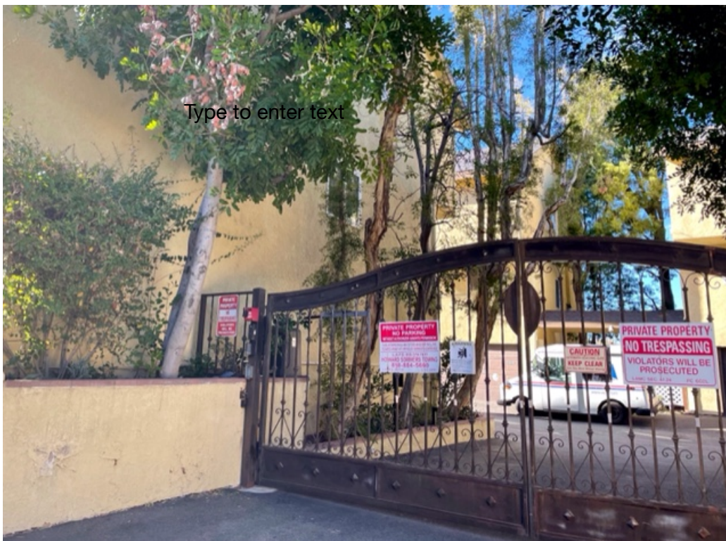
Via Del Valle Townhouses Entrance Gate. (11-25-2022)
