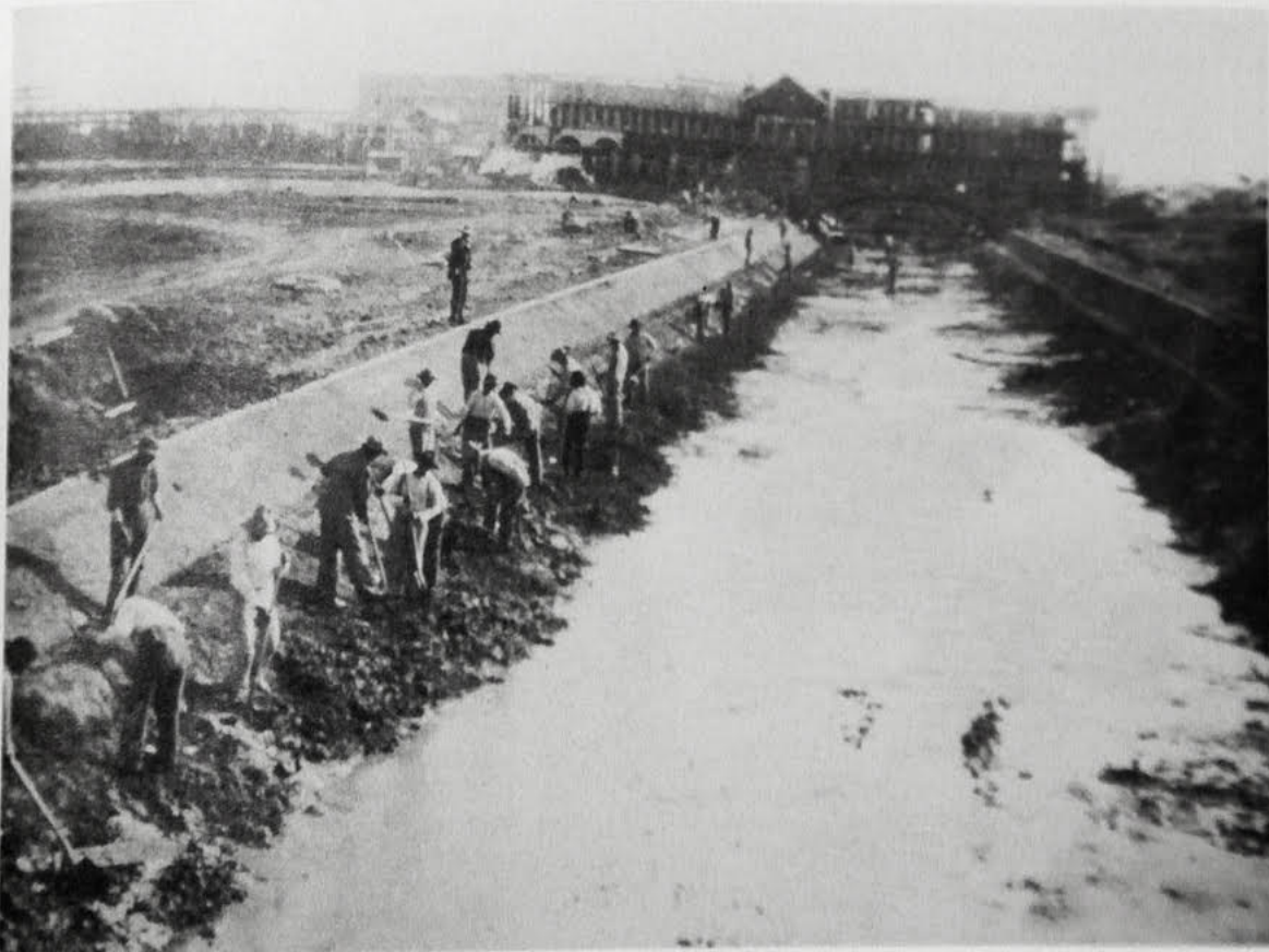
Constructing the canal's sloping sides, circa 1905.
