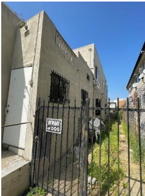
Figure 14. 318 N. Oxford Avenue Northern Façade (view southwest) SOURCE: Sapphos Environmental, Inc., 2023
