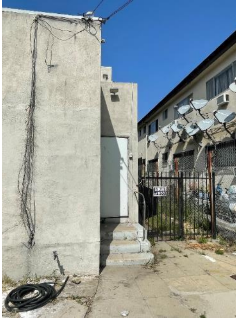
Figure 13B. 318 N. Oxford Avenue Eastern Façade (view west) SOURCE: Sapphos Environmental, Inc., 2023
