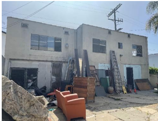
Figure 15. 318/320 N. Oxford Avenue Additional Building Northern Façade (view east) SOURCE: Sapphos Environmental, Inc., 2023
