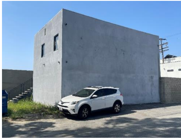
Figure 17A. 311 N. Serrano Avenue SOURCE: Sapphos Environmental, Inc., 2023
