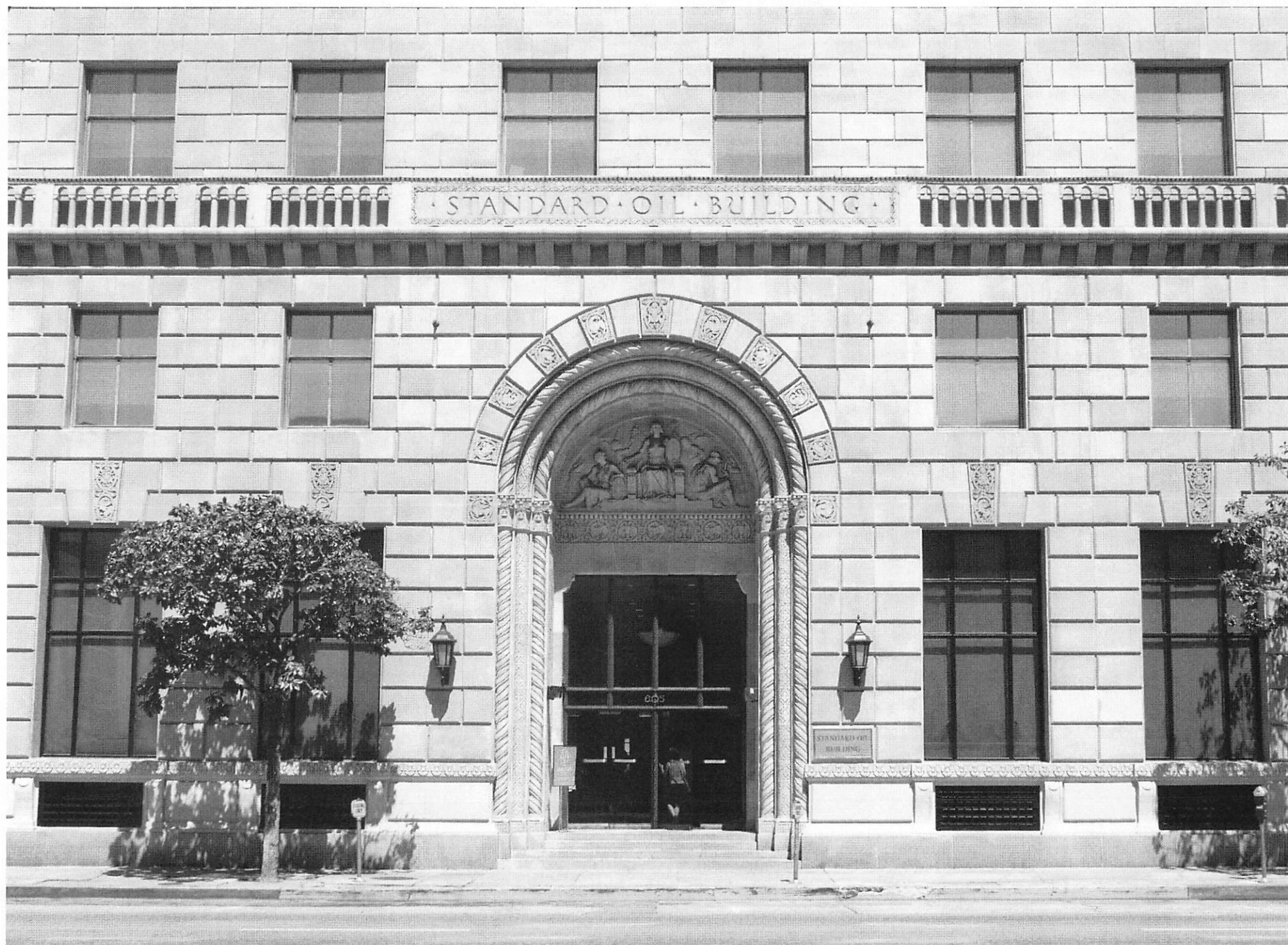
Standard Oil Company Building
