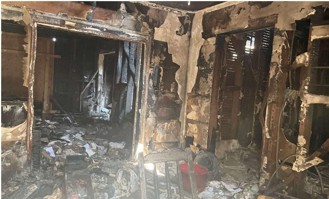
Image 15: Interior, view northwest
