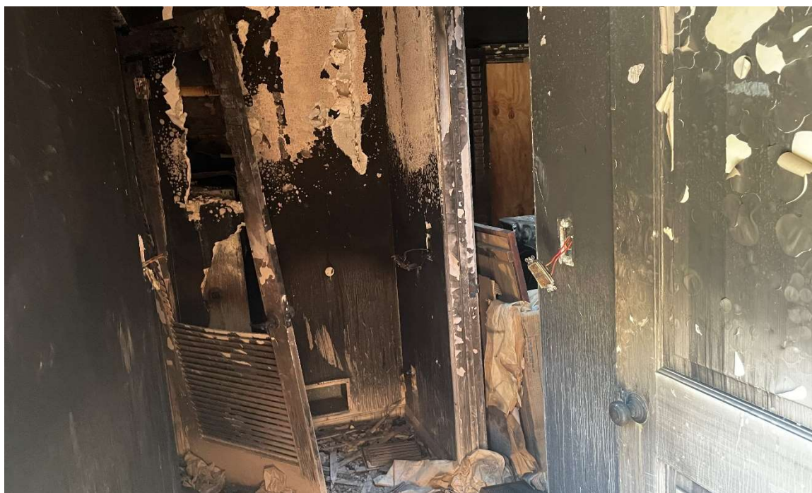
Image 14: Interior, view northwest
