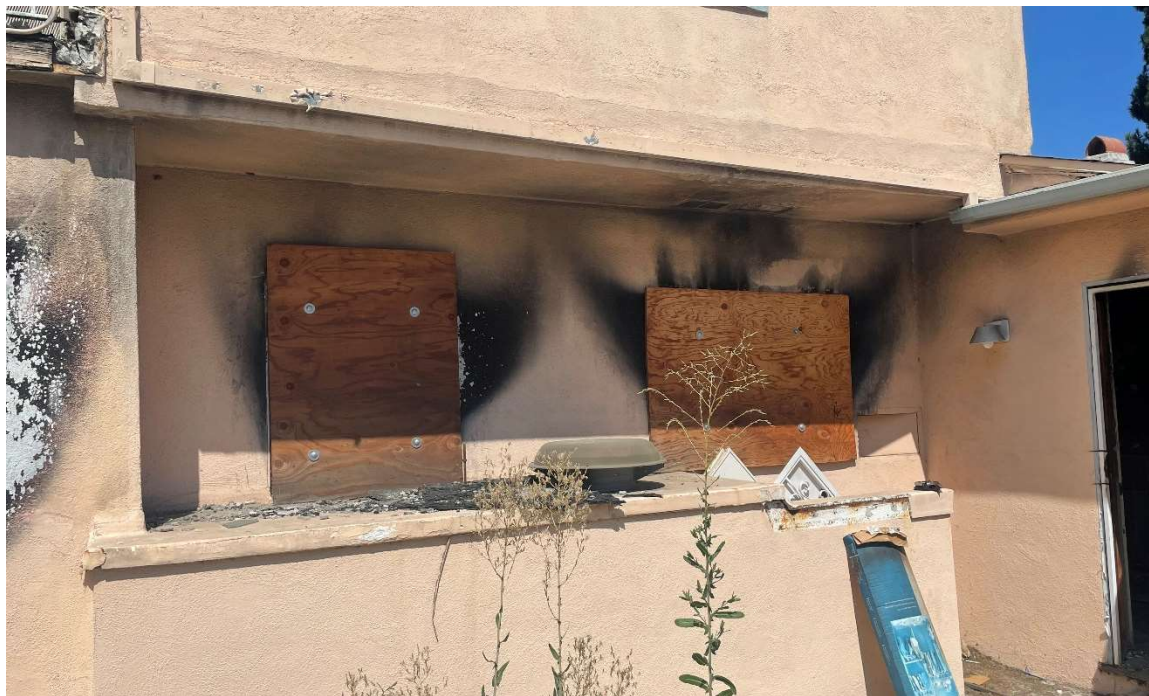
Image 13: Rear (east) façade, missing windows and smoke-damaged walls
