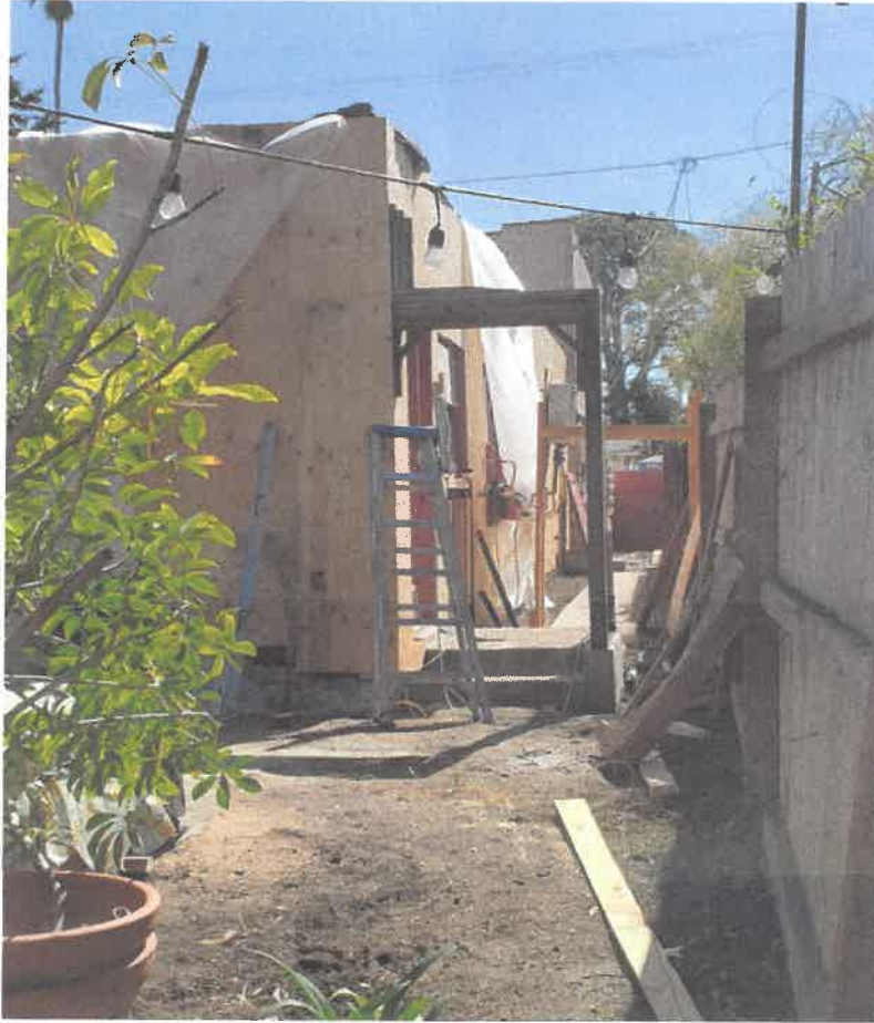
West building, 3/18/25; Note that original arched buttress was removed, but appears to be reconstructed here; similar original arched buttress on east building remains
