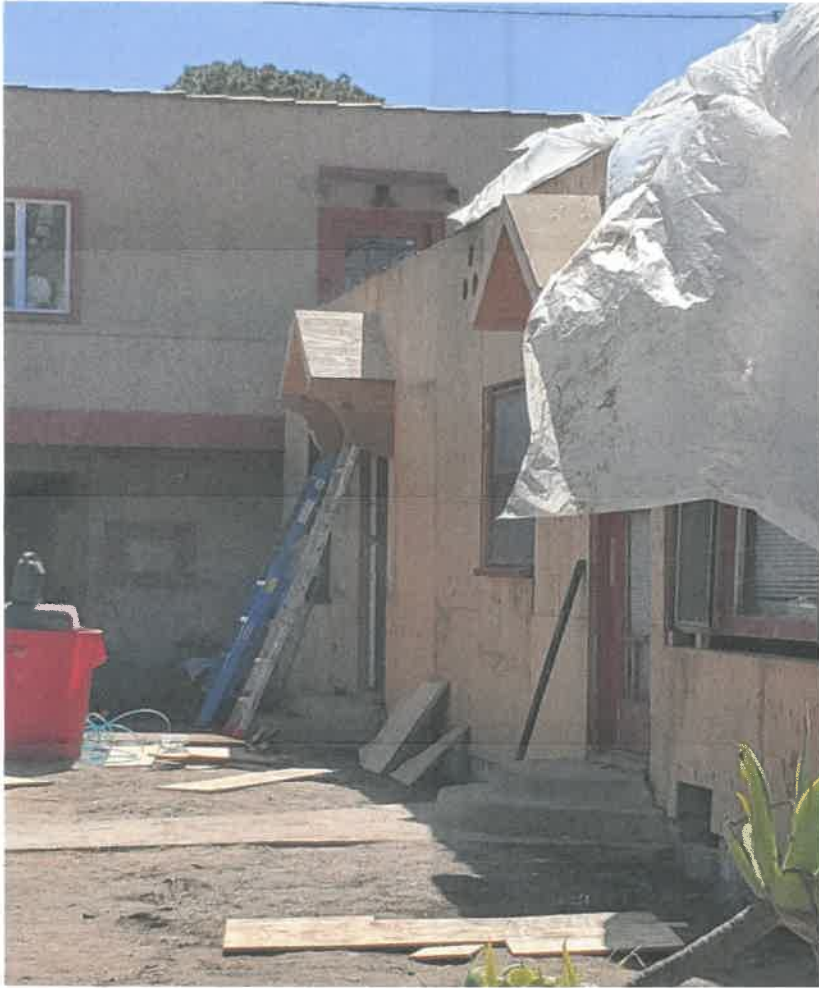
West building, 3/18/25; building being prepared for new stucco; note that new over-door awnings have been added; note that circular vents and original wooden multi-lite doors and windows remain
