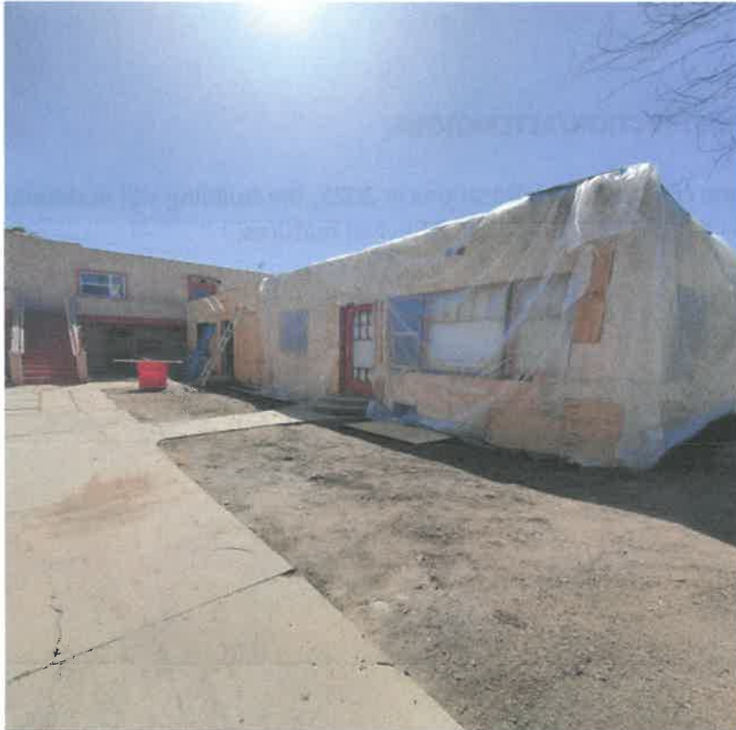
West building, 3/18/25; building is being prepared for re-stucco; note that original wooden multi-lite doors and windows, as well as circular vents, remain
