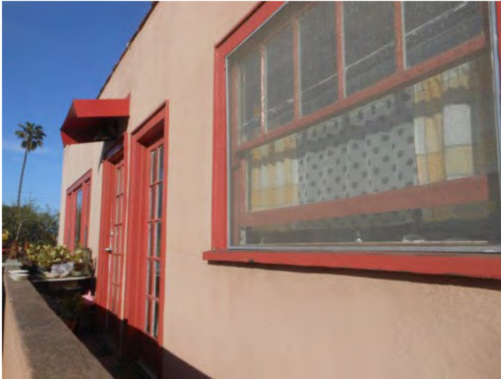
27. 926 ½ Marco Place, north elevation
