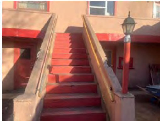
Stairway up to 926 and 926 1/2 Marco Place
