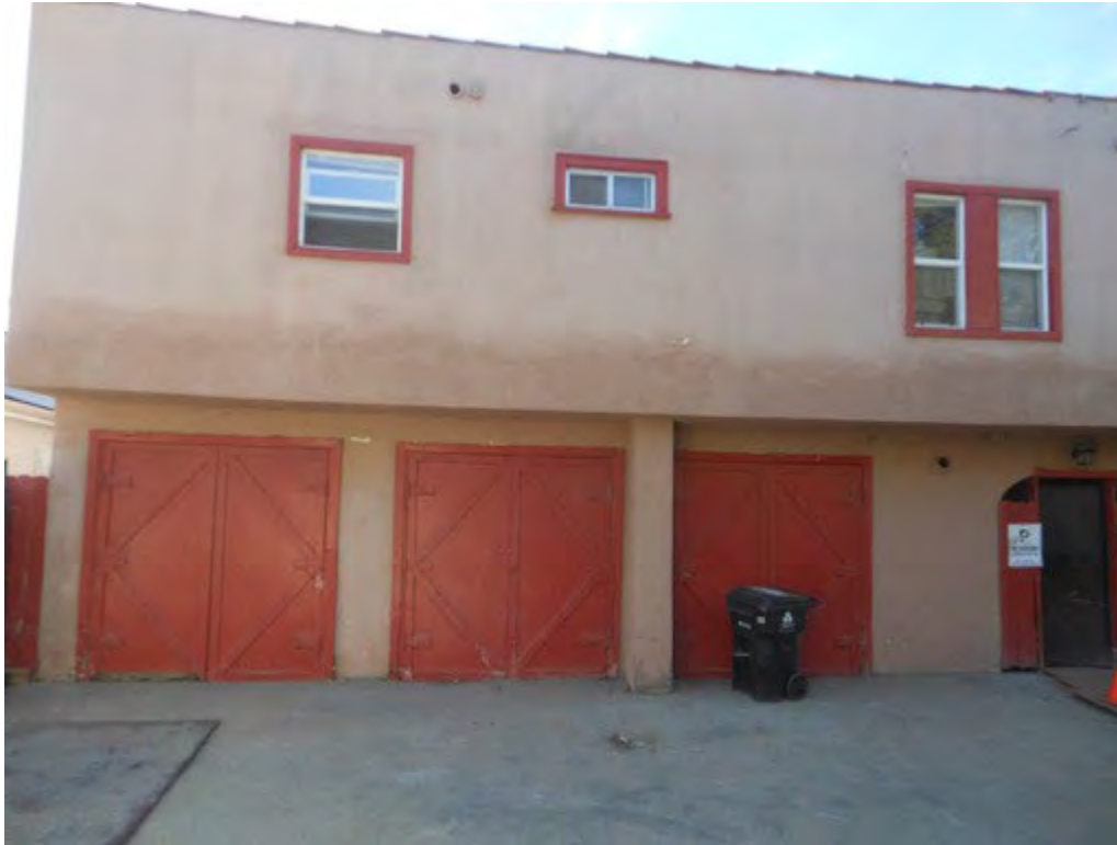
35. 926 Marco Place, rear (south) elevation
