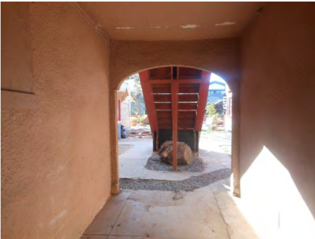
32. Area under stairway and corridor to alley, looking north
