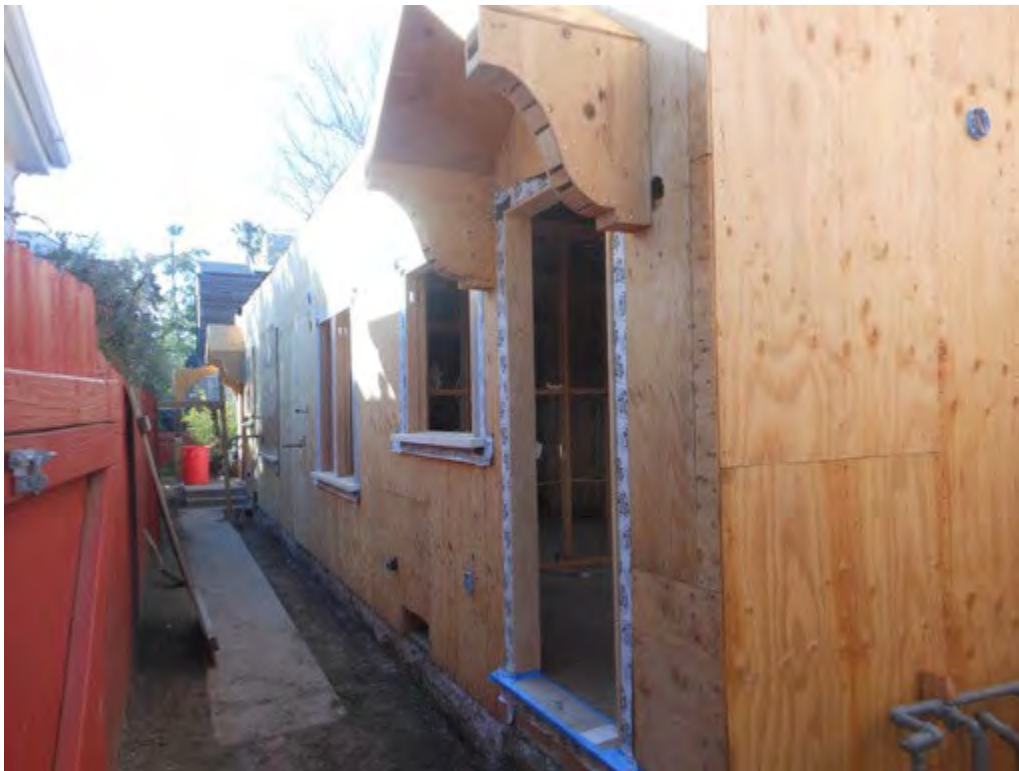
22. 924-924 ½ Marco Place, rear (east) elevation
