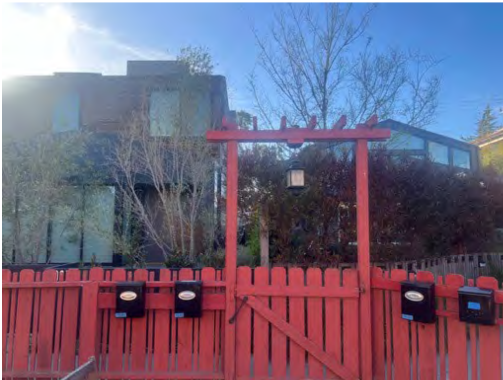
6. Gate and fence of 924-928 Marco Place
