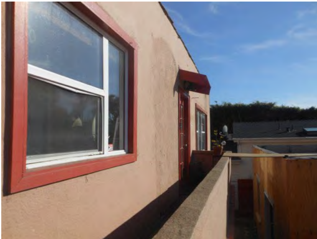
26. 926 Marco Place, north elevation
