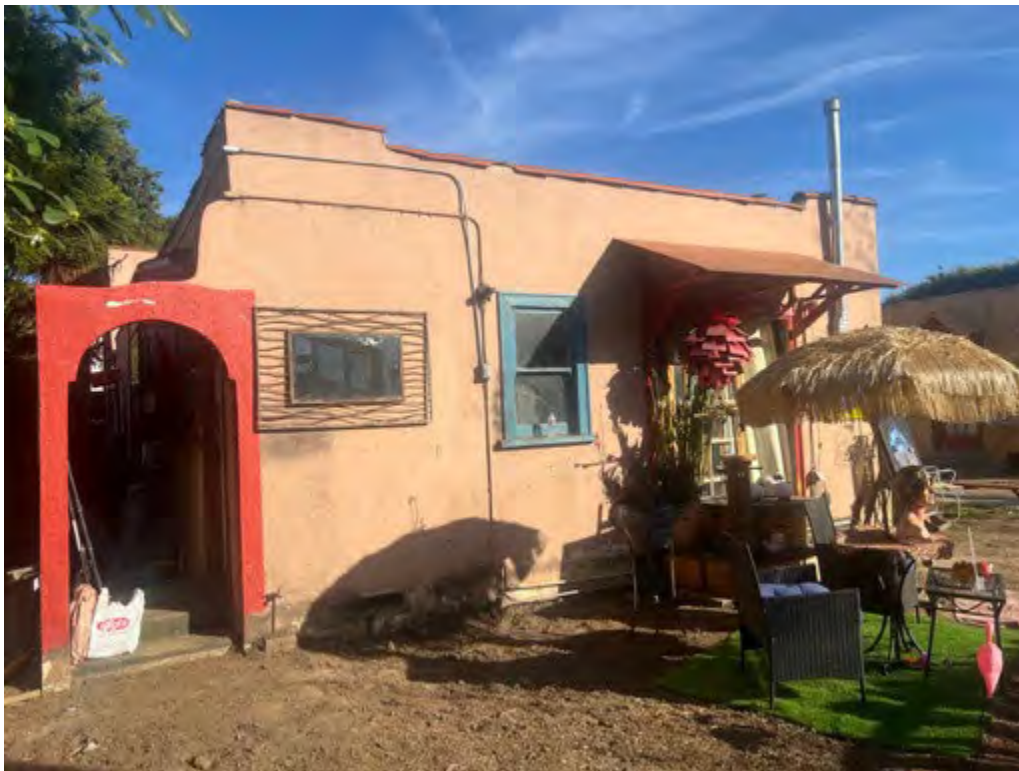
12. 928 ½ Marco Place, north elevation
