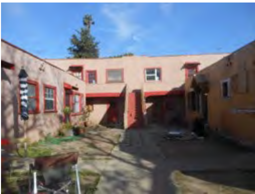
926 -926 1/2 Marco Place, north elevation
