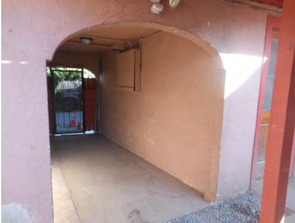
33. Area under stairway and corridor to alley, looking south
