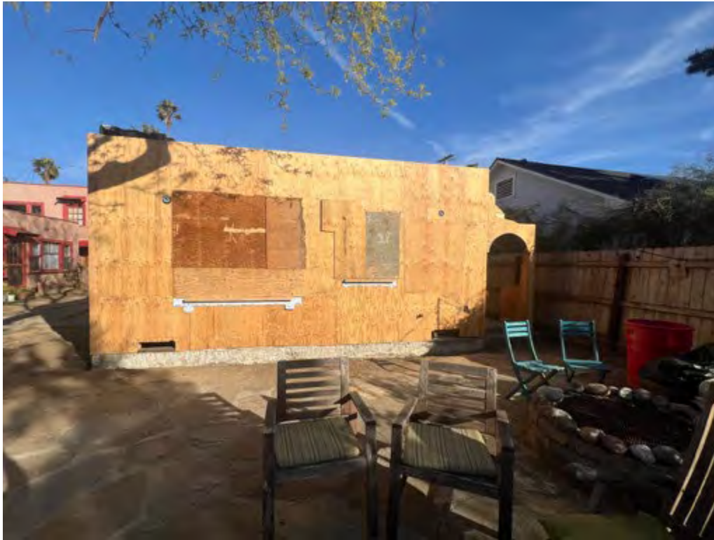
19. 924 Marco Place, north elevation
