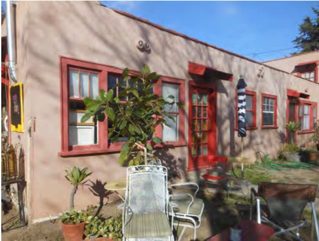
15. 928 ½ and 928 Marco Place, east elevation
