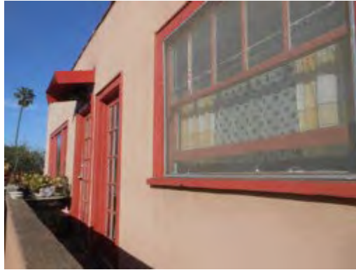
926 1/2 Marco Place, north elevation
