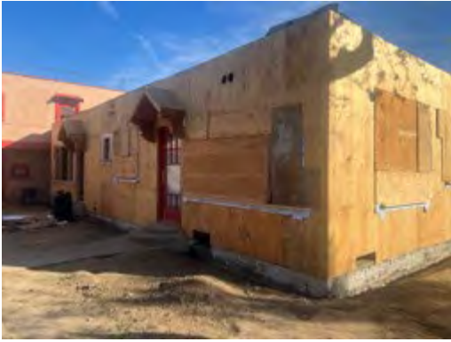
924 Marco Place, north and east elevations
