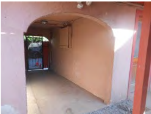
Area under stairway and corridor to alley, Looking south
