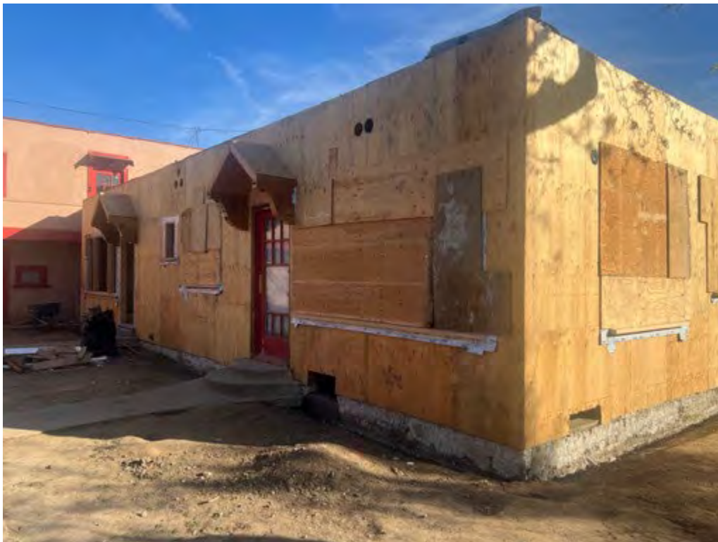
20. 924 Marco Place, north and east elevations
