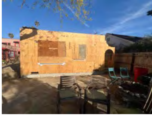
924 Marco Place, north elevation
