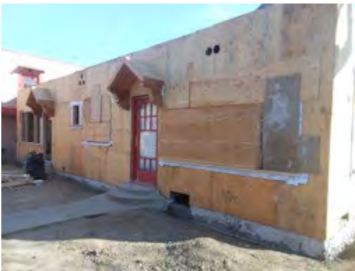
924 and 924 1/2 Marco Place, east elevation
