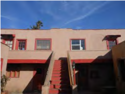
926 -926 1/2 Marco Place, north elevation, stairs and windows
