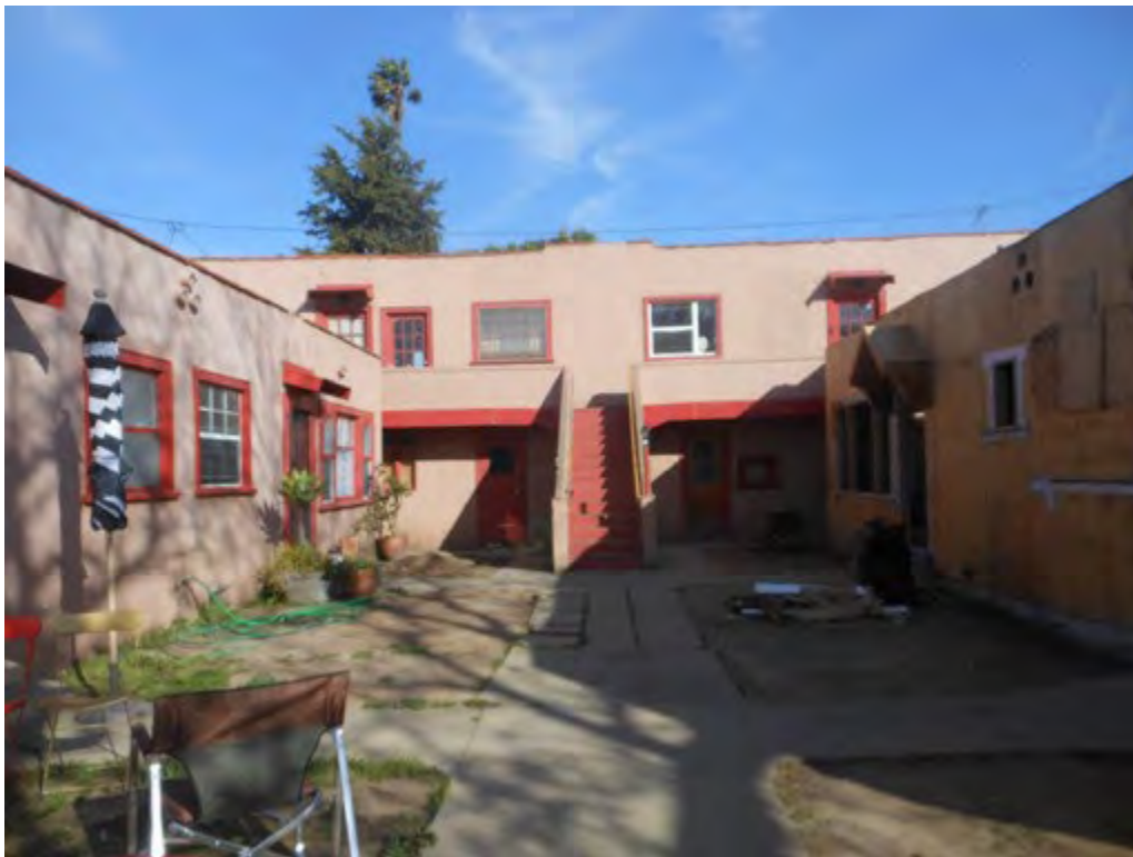
8. 924-928 Marco Place, looking south
