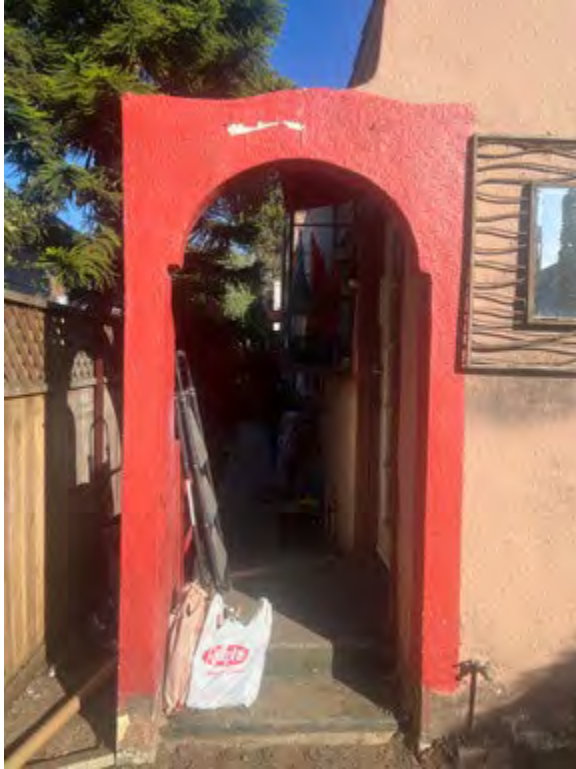
13. 928 ½ Marco Place, east end of north elevation
