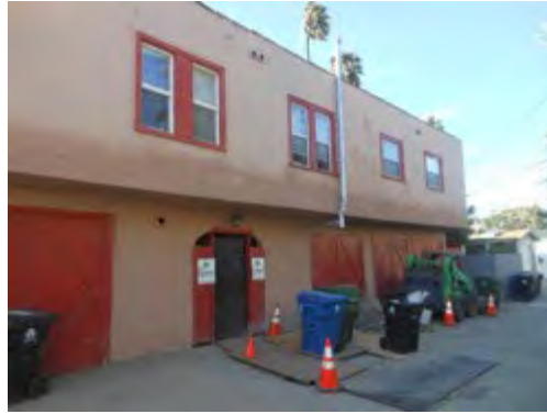
926 and 926 ½ Marco Place, south elevation
