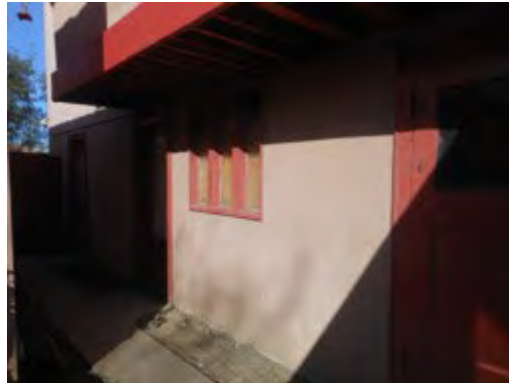
Lower level of 926 1/2 Marco Place, north elevation
