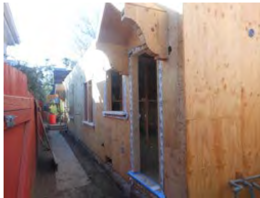
924-924 1/2 Marco Place, rear (east) elevation
