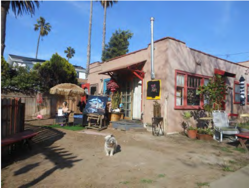
11. 928 ½ Marco Place, north and west elevations
