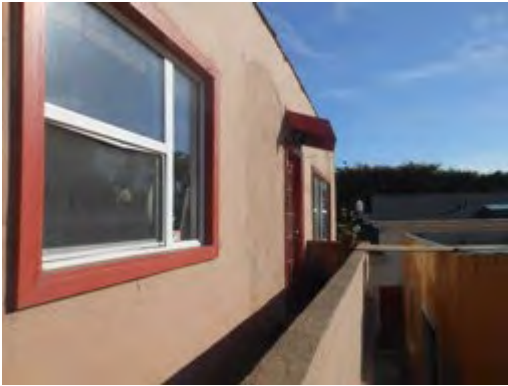
926 Marco Place, north elevation
