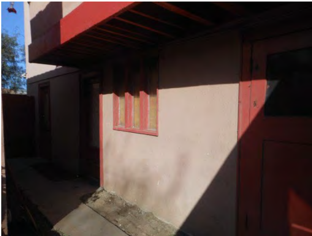
30. Lower level of 926 ½ Marco Place, north elevation
