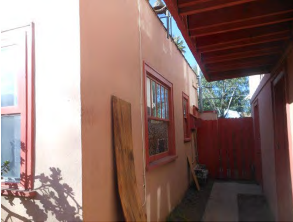
29. South elevation of 928 Marco Place and north elevation of lower level of 926 ½ Marco Place
