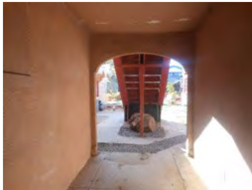
Area under stairway and corridor to alley, looking north
