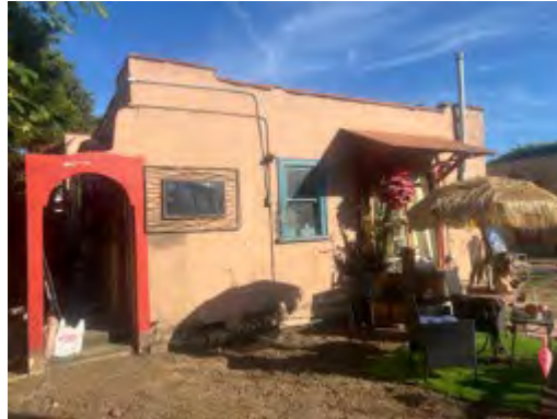
928 ½ Marco Place, north elevation
