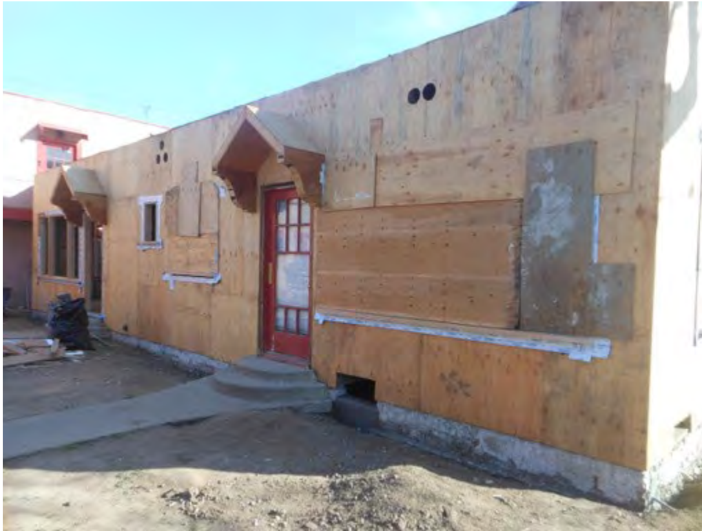
21. 924 and 924 ½ Marco Place, east elevation
