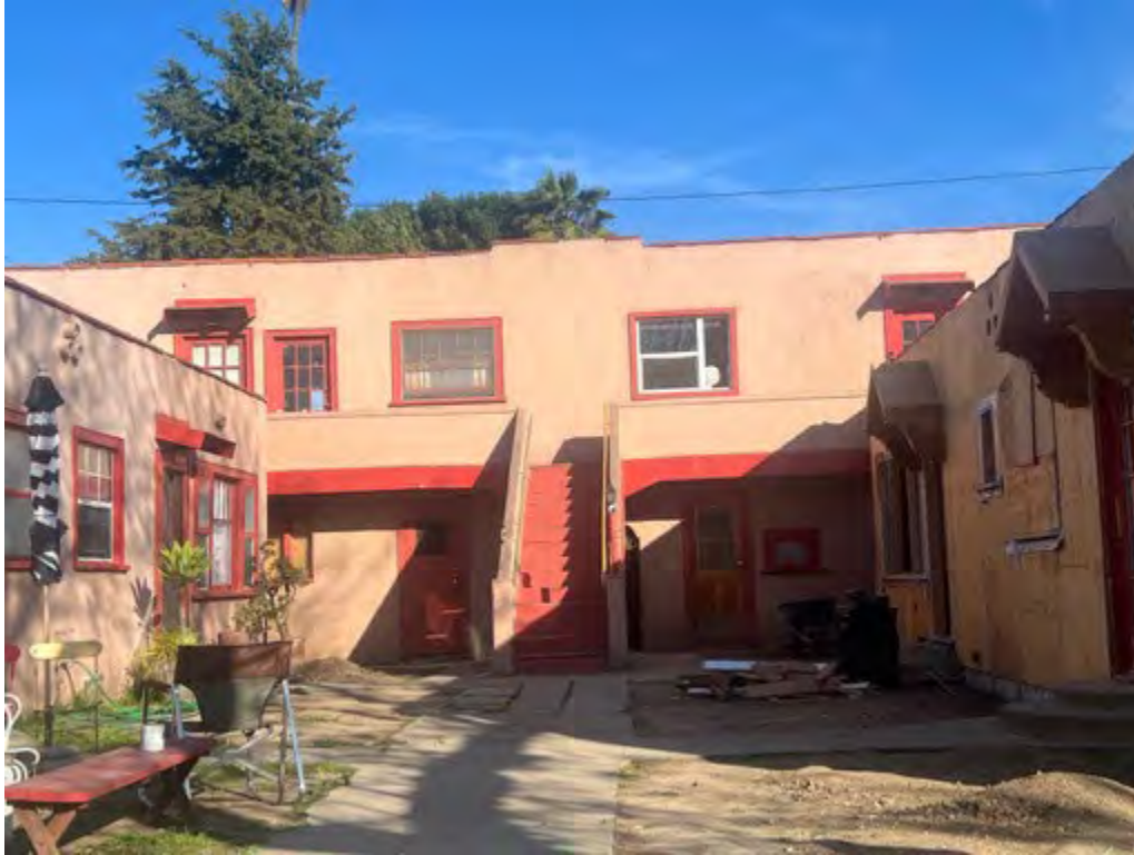
23. 926 -926 ½ Marco Place, north elevation
