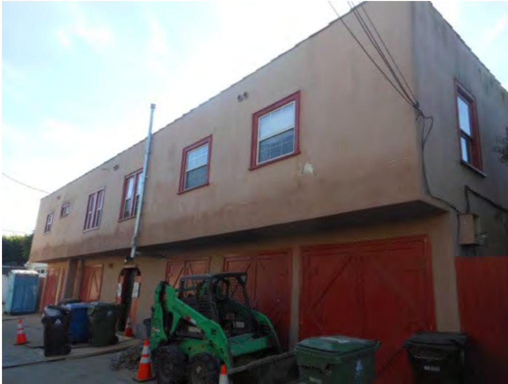
37. Rear (south) elevation of 926 and 926 ½ Marco Place with residences above and garages below
