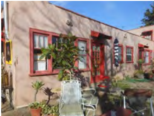
928 ½ and 928 Marco Place, east elevation
