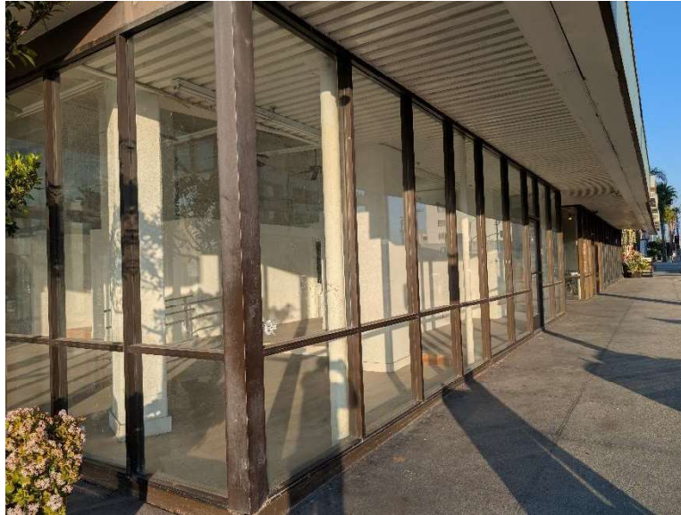
Detailed View of Contemporary Storefronts
