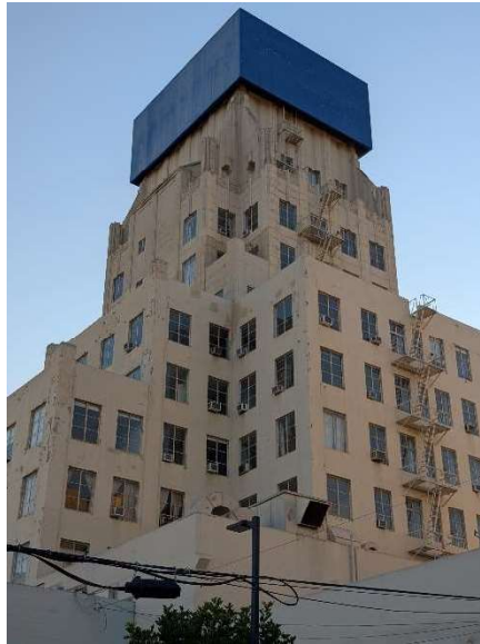
View of Upper Floors and Capital. Note removed finials.
