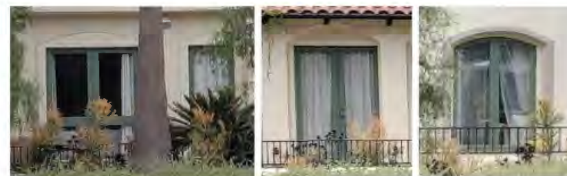
MATCHING WINDOWS OF 3 ADJACENT PROPERTIES
