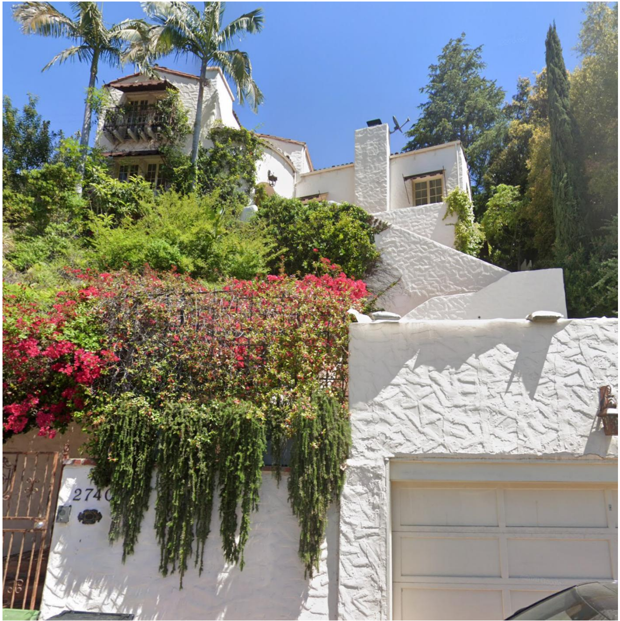
1920'S SPANISH REVIVAL HOUSE ON WOODHAVEN DRIVE
