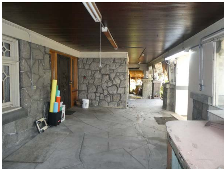
Figure 3: Tokio Florist/Sakai-Kozawa Residence, first-story porch, view looking south (GPA, 2019)
