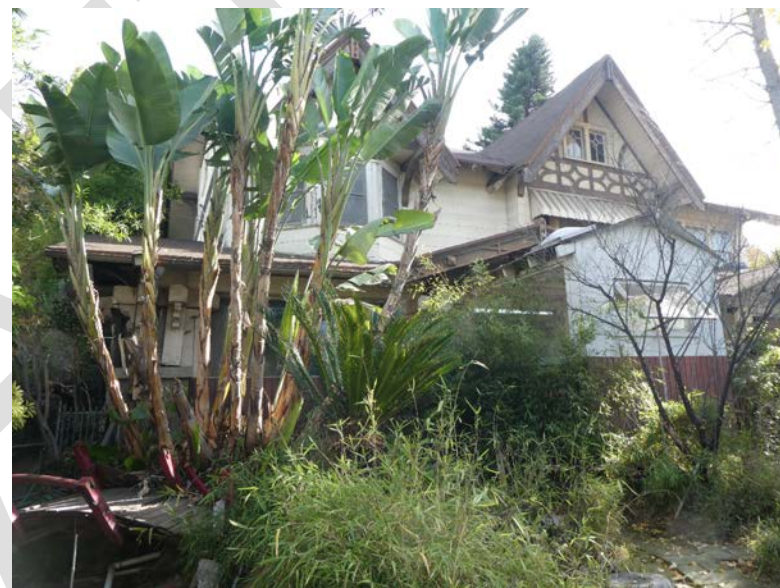
Figure 2: Tokio Florist/Sakai-Kozawa Residence, circa 1911 residential building, view looking southeast (GPA, 2019)
