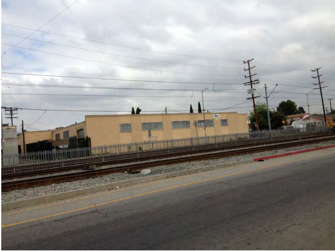
Photo 16 - A railroad right-of-way and commercial/industrial sites, across Long Beach Avenue to the west
