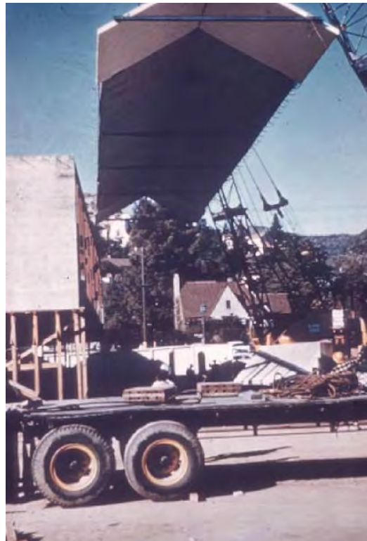
Figure 47 Placement of Folded Panels on Bank Under Construction, 1959 (Kurt Meyer Archives)
