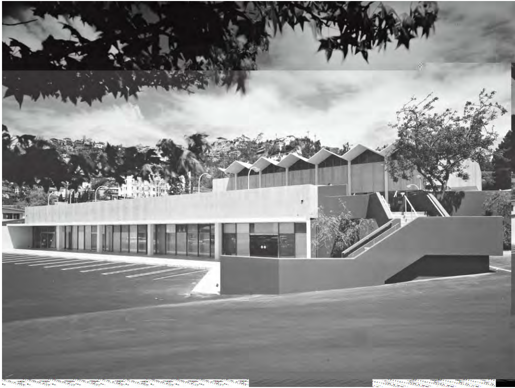
Figure 51 Lytton Center, Primary (South) Elevation, Photographed by Julius Shulman 1962 (Julius Shulman photography archive, 1936-1997. Series IV. Job numbers, 1934-2009( http://hdl.handle.net/10020/cat657475 ) GRI Special Collections)
