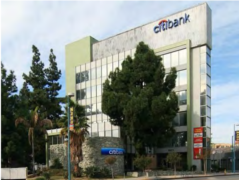
Figure 19 Commonwealth S & L, 5077 Lankershim Boulevard, North Hollywood, Architect Gerald H. Bense, Constructed 1961 ( http://www.you-are-here.com/modern/commonwealth.html )
