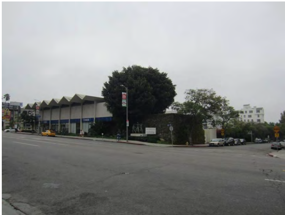
Figure 88 Bank, Primary (North) and West Elevations, View Southeast (PCR 2013)
