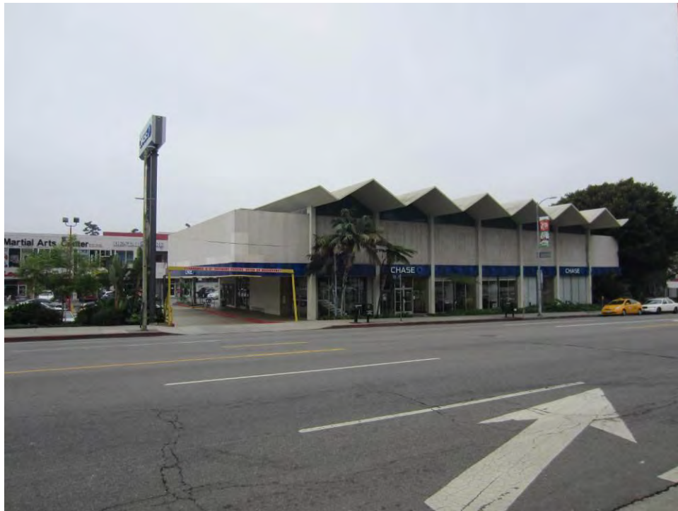
Figure 83 Home Branch, Primary (North) Elevation, View Southwest (PCR 2013)
