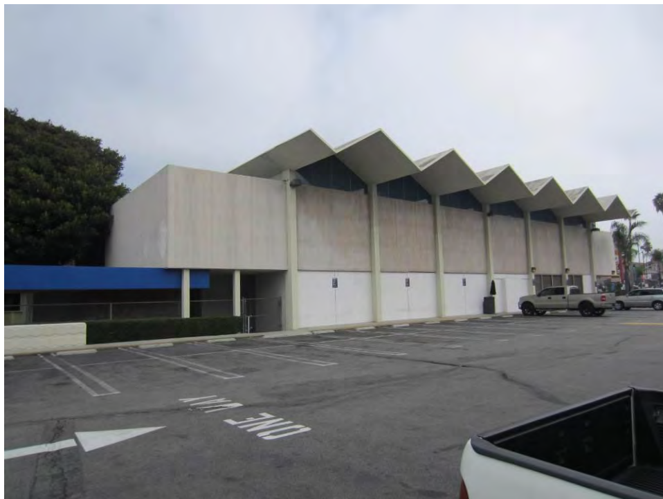
Figure 93 Bank, Rear (South) Elevation, View Northeast (PCR 2013)
