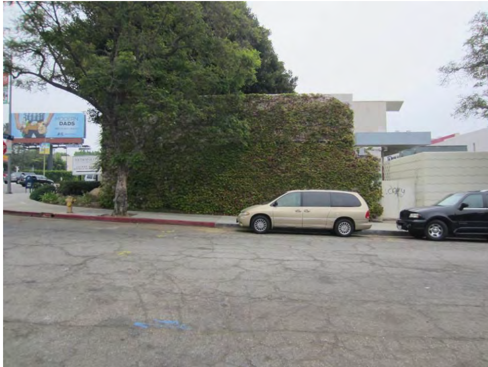
Figure 95 Bank, Side (West) Elevation, View East (PCR 2013)
