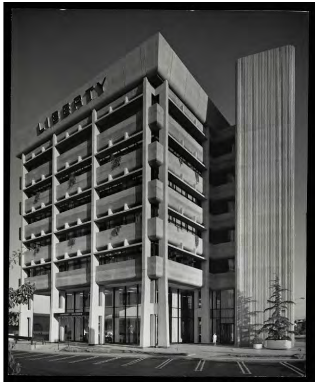
Figure 69 Liberty S & L, 1180 S. Beverly Drive, West Los Angeles, Constructed 1966, Photographed by Julius Shulman 1966-1967 (Julius Shulman photography archive, 1936-1997. Series IV. Job numbers, 1934-2009( http://hdl.handle.net/10020/cat657475 ) GRI Special Collections)
