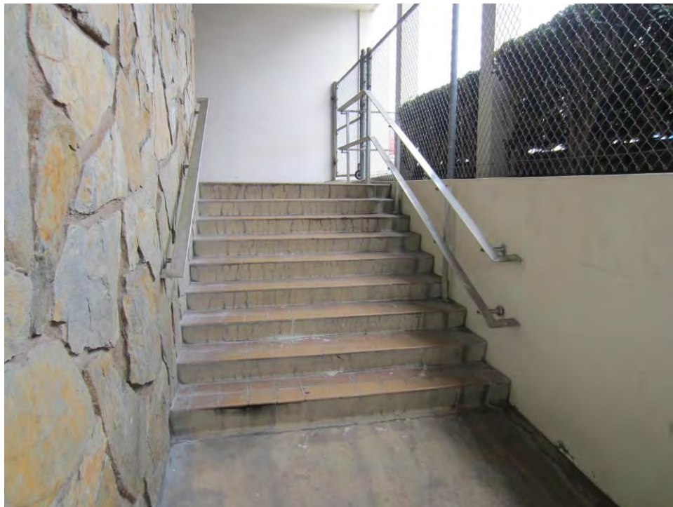
Figure 96 Bank, Set of Stairs Leading to Secondary Entrance, Side (West) Elevation, View East (PCR 2013)
