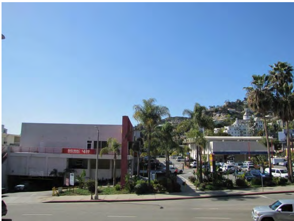
Figure 82 Project Site, Strip Mall to Left, Lytton Bank to Right, View West (PCR 2013)
