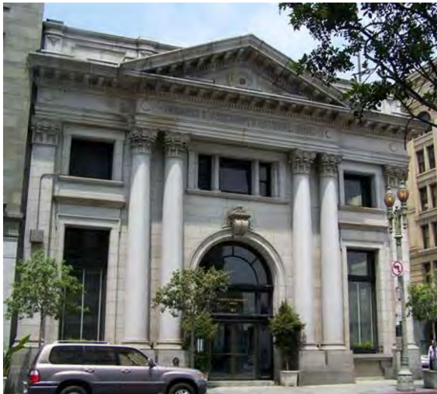
Figure 12 Farmers and Merchants National Bank, 4th and Main Street, Downtown Los Angeles, Constructed 1923 (Google Street View)
