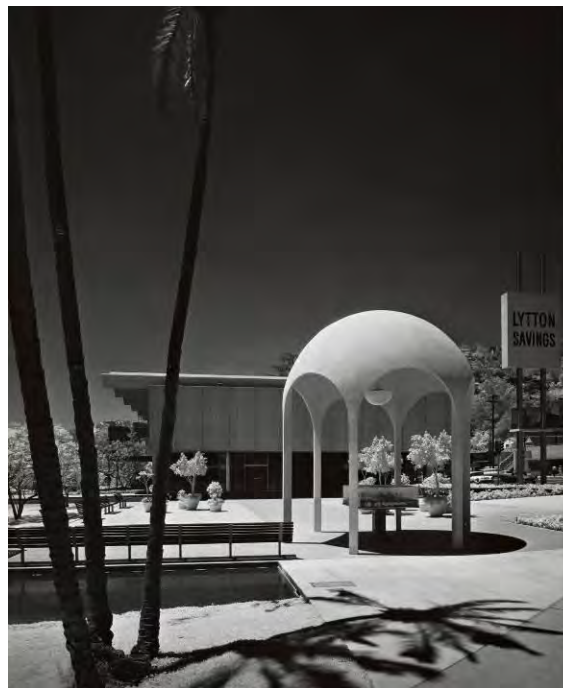
Figure 40 Plaza, Pavilion, and Reflecting Pool of Lytton Savings Home Branch, Public Relations Photographs of New Home Office, June 22, 1960, View to West (Julius Shulman Photography Archive, 1935-2009, Box 524, Getty Research Institute)
