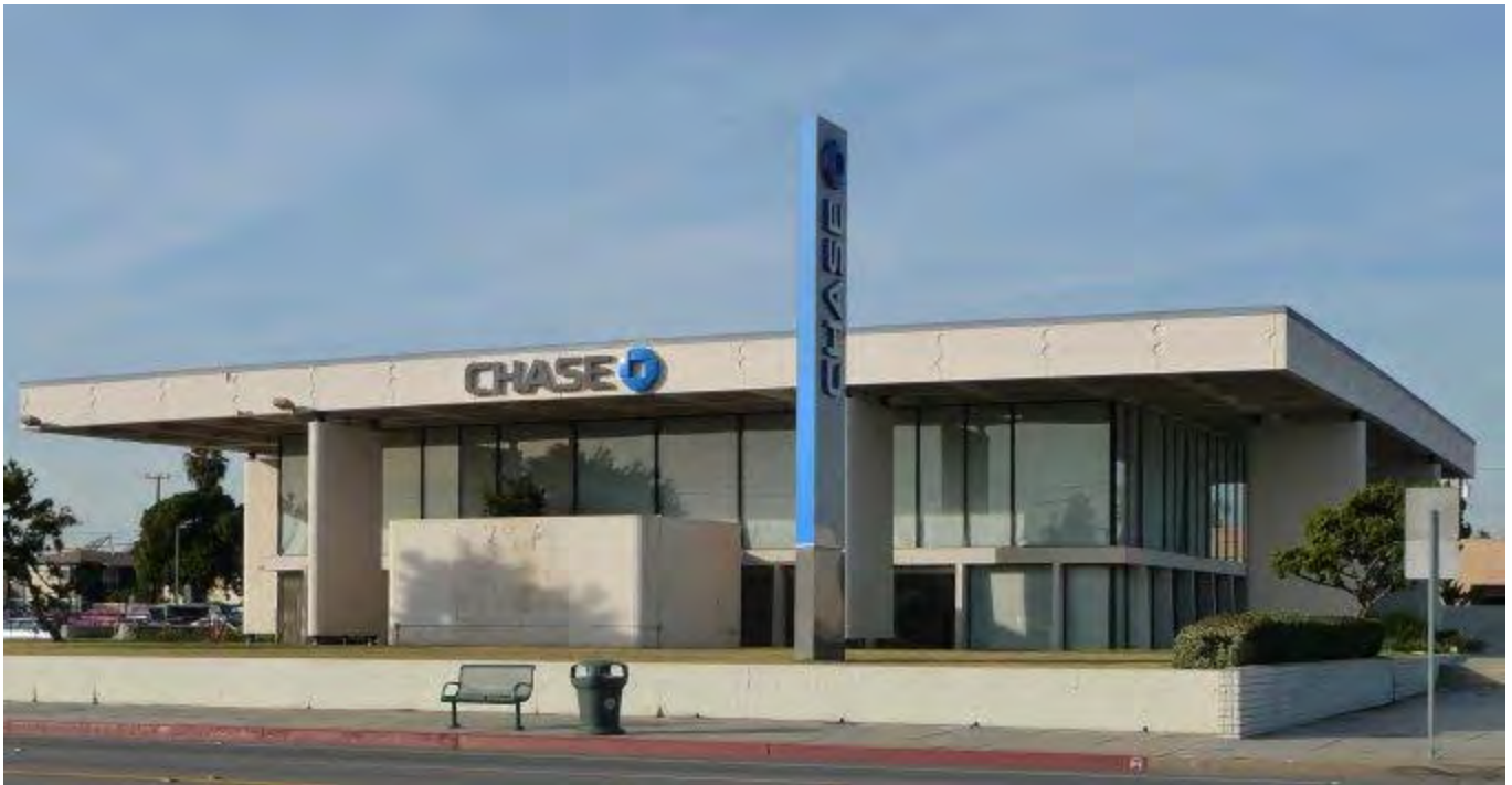
Figure 21 Great Western Savings and Loan, 2501 W. Rosecrans Avenue, Gardena, Designed by Paffard Keatinge-Clay of Skidmore, Owings & Merrill, Constructed 1961 ( https://www.laconservancy.org/locations/chase-bank-gardena )
