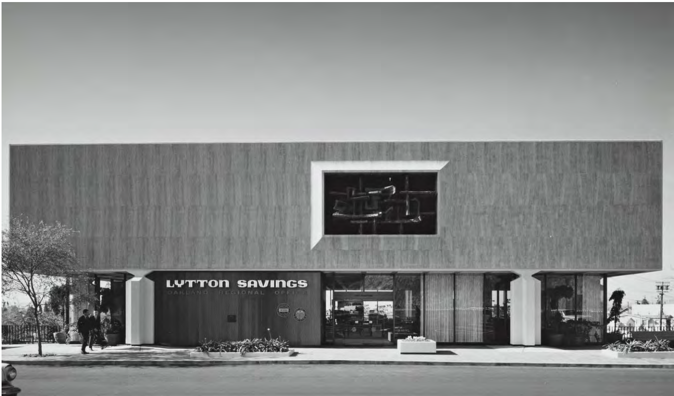
Figure 67 Lytton Savings Oakland Branch, Kurt Meyer Architect, Photographed by Julius Shulman 1966 (Julius Shulman photography archive, 1936-1997. Series IV. Job numbers, 1934-2009( http://hdl.handle.net/10020/cat657475 ) GRI Special Collections)
