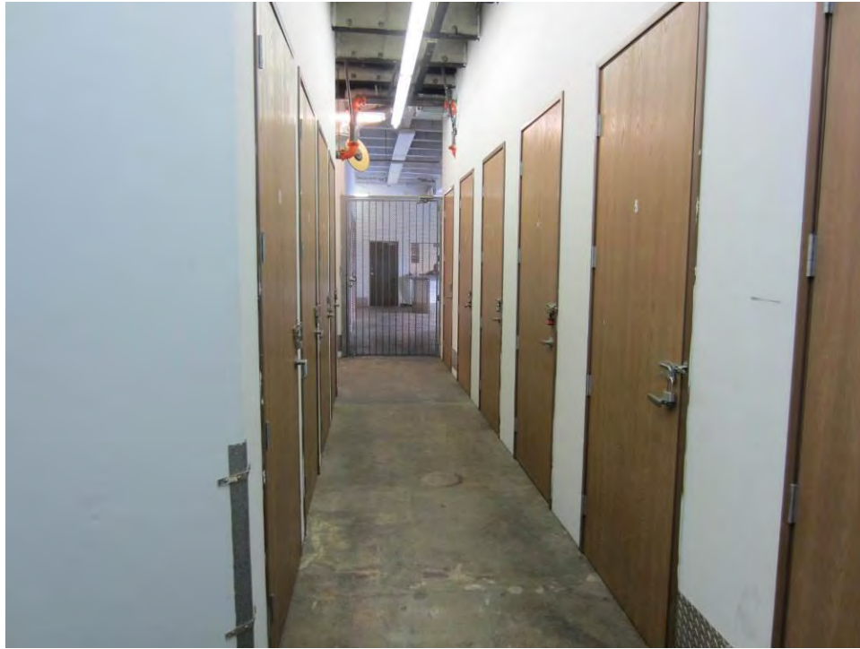
Figure 107 Former Lytton Center now Art Storage (PCR 2013)
