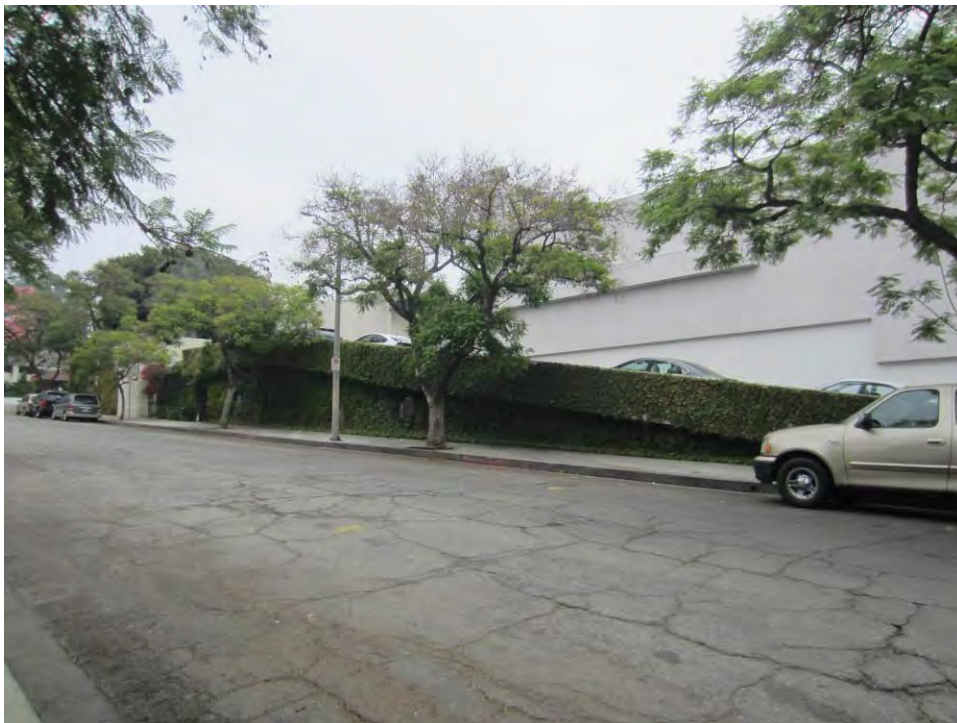
Figure 86 Ramp to Lytton Center Parking Lot and West Elevation of Addition, View North (PCR 2013)
