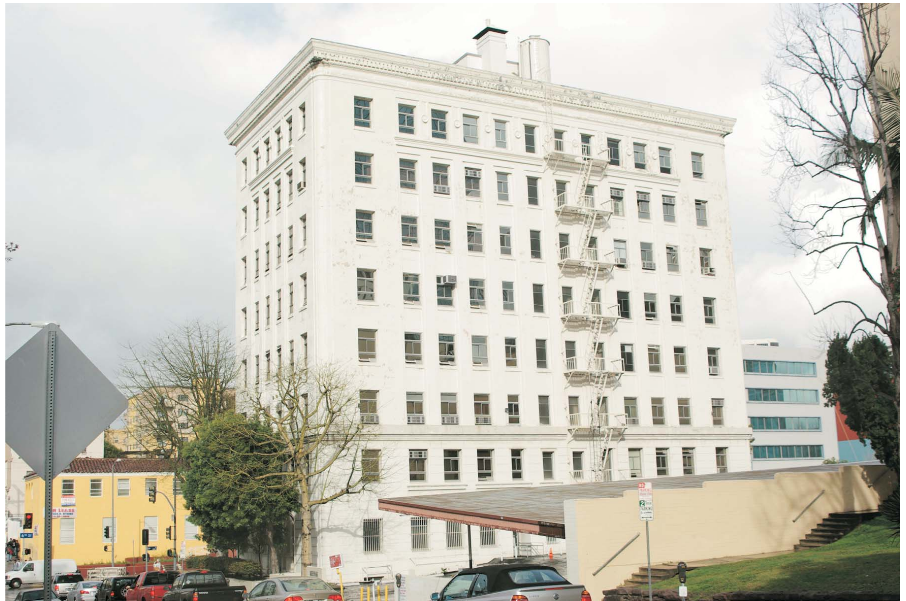
Figure 6 Medical Office Building, 1136 W. Sixth Street South and West Elevations, View to Northeast
