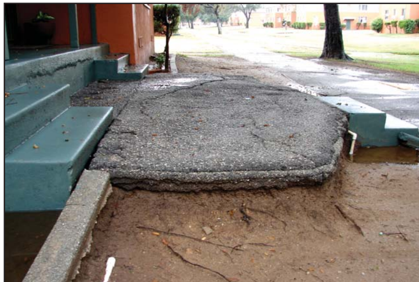
View 2: Erosion and exposed pipes
