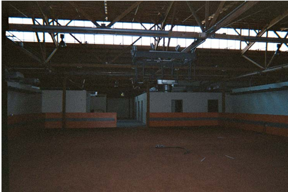
Photograph 10: Inside building at 1933 S. Bundy Drive.
