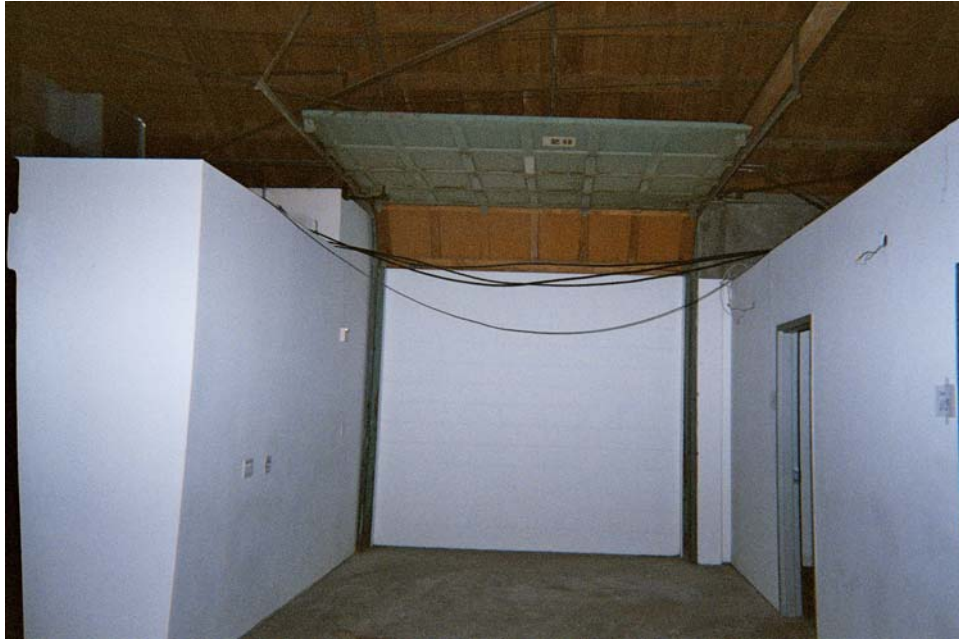
Photograph 11: A former roll-up bay door that has been re-bricked.
