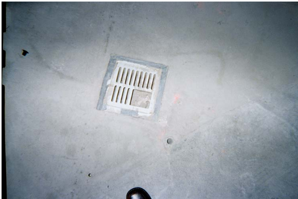
Photograph 12: Floor drain inside building at 1901 S. Bundy Drive.
