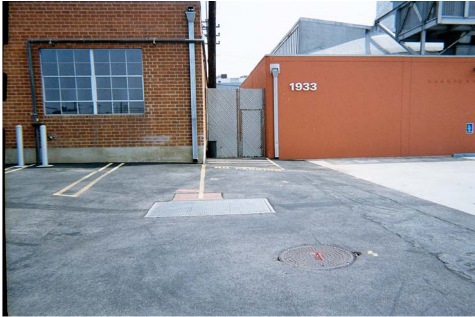
Photograph 9: Utility vaults and manhole covers between 1925 and 1933 S. Bundy Drive buildings.
