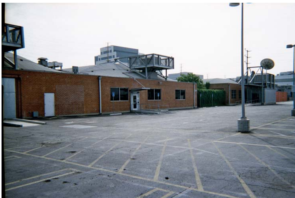
Photograph 2: Buildings at 1925 and 1933 S. Bundy Drive.
