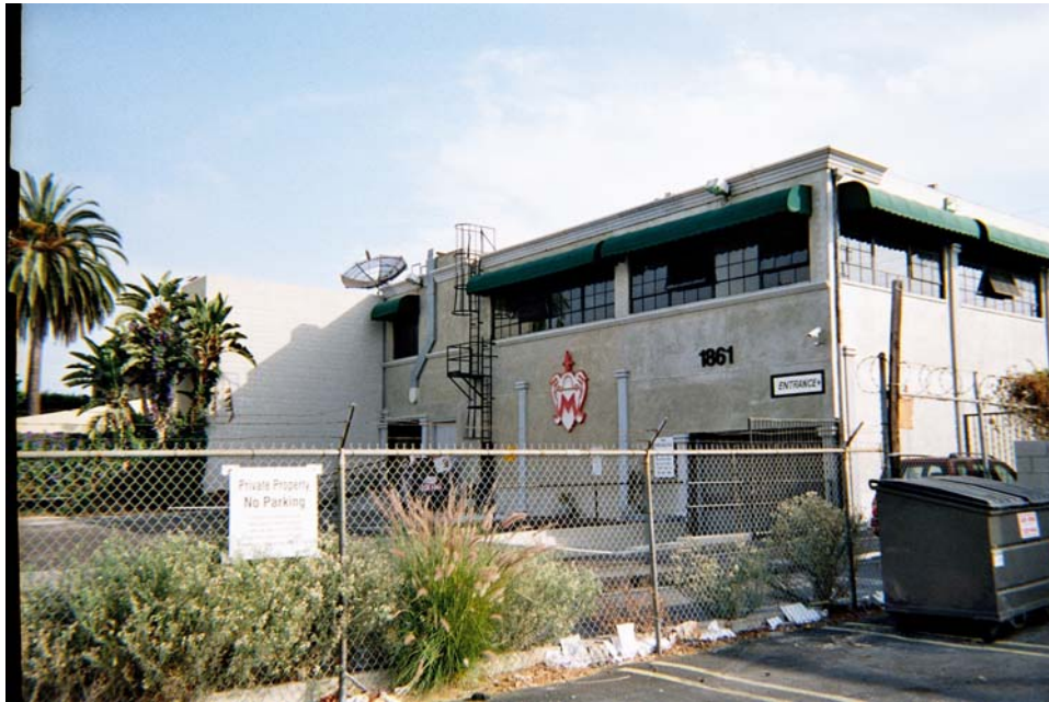
Photograph 5: Adjacent multi-tenant building at 1861 S. Bundy Drive.
