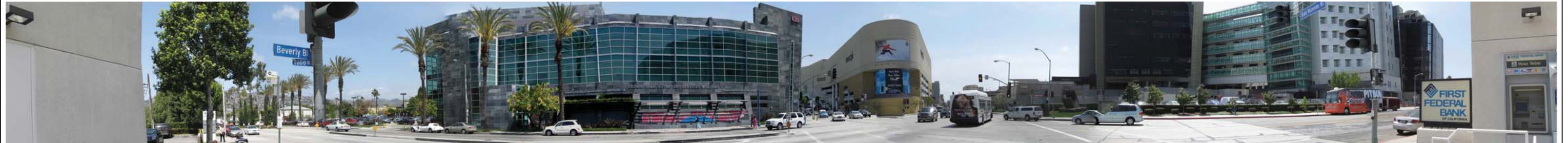
LOOKING SOUTHWEST TOWARD CSMC CAMPUS
