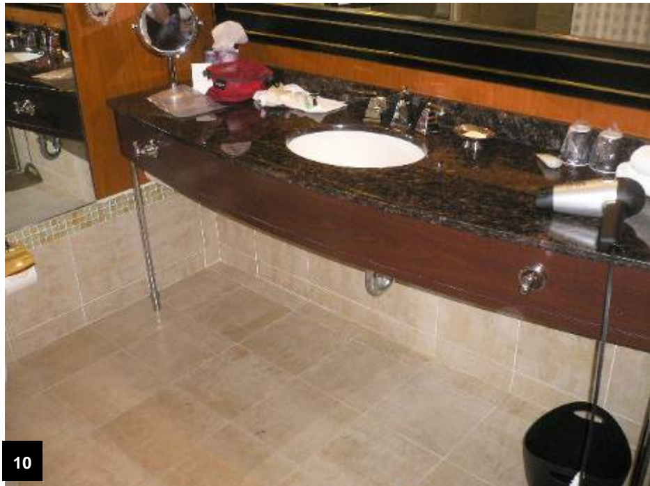
Typical unit bathroom
