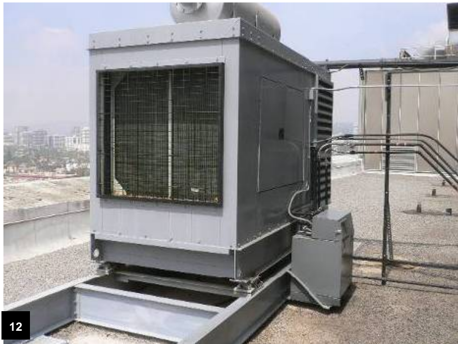
Emergency generator on roof
