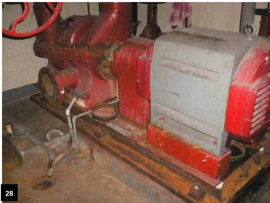
Old fire pump (electric)
