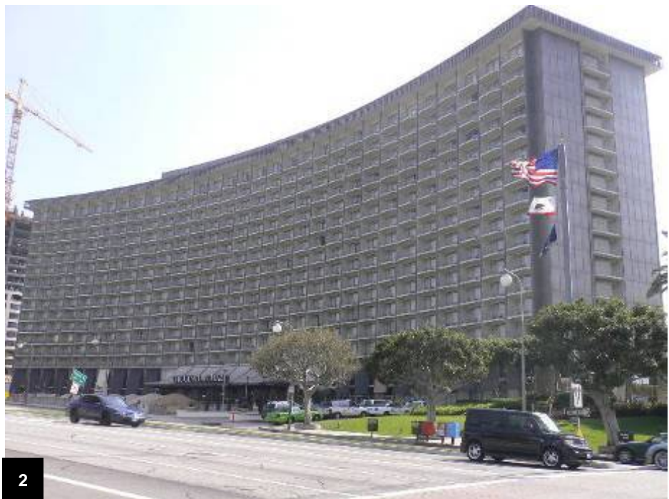
Subject building from the north
