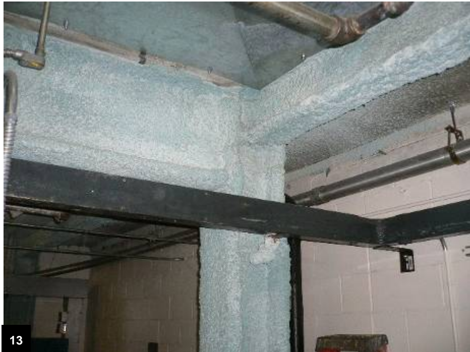
New spray-on fire proofing
