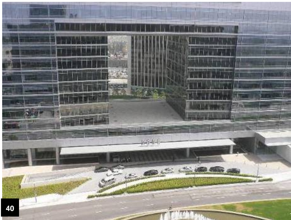
Surrounding property to the northeast
