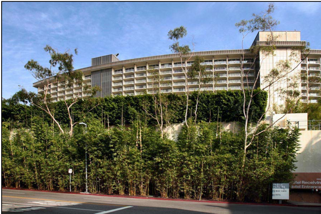
Photograph 4: Eastern view of Project Site from Garden Lane showing rear of existing hotel.
