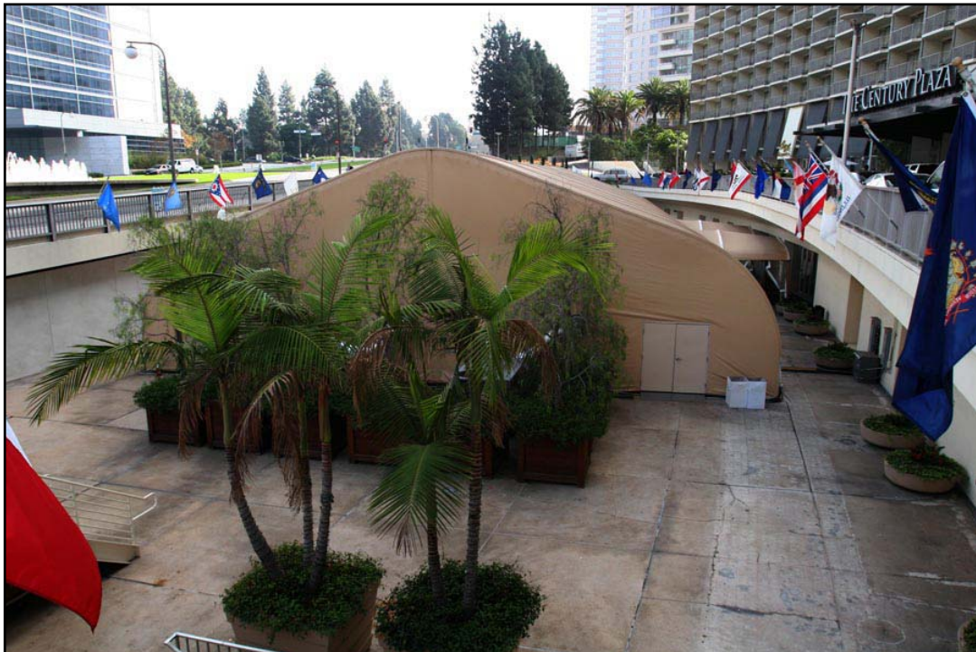
Photograph 6: Southern (onsite) view of sunken area fronting Avenue of the Stars.
