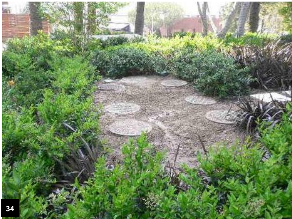
Grease interceptors for X Bar restaurant
