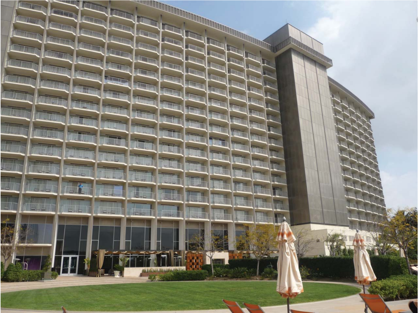
West facade, view looking southeast
