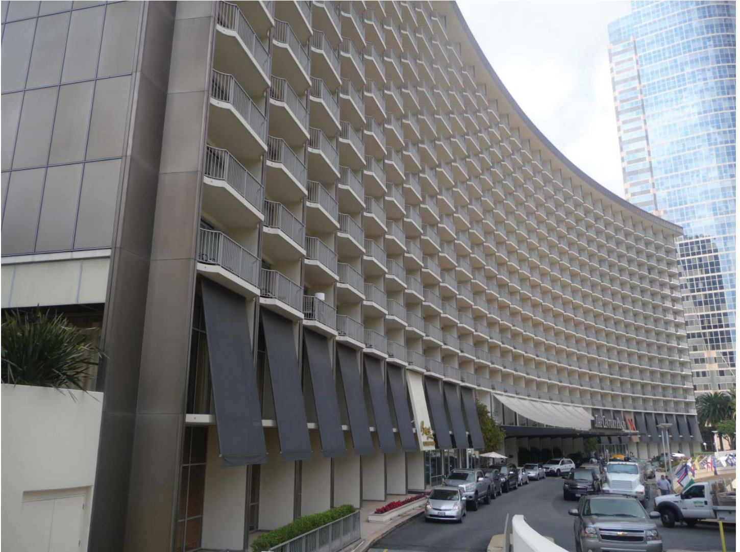
Main (east) facade, view looking northwest
