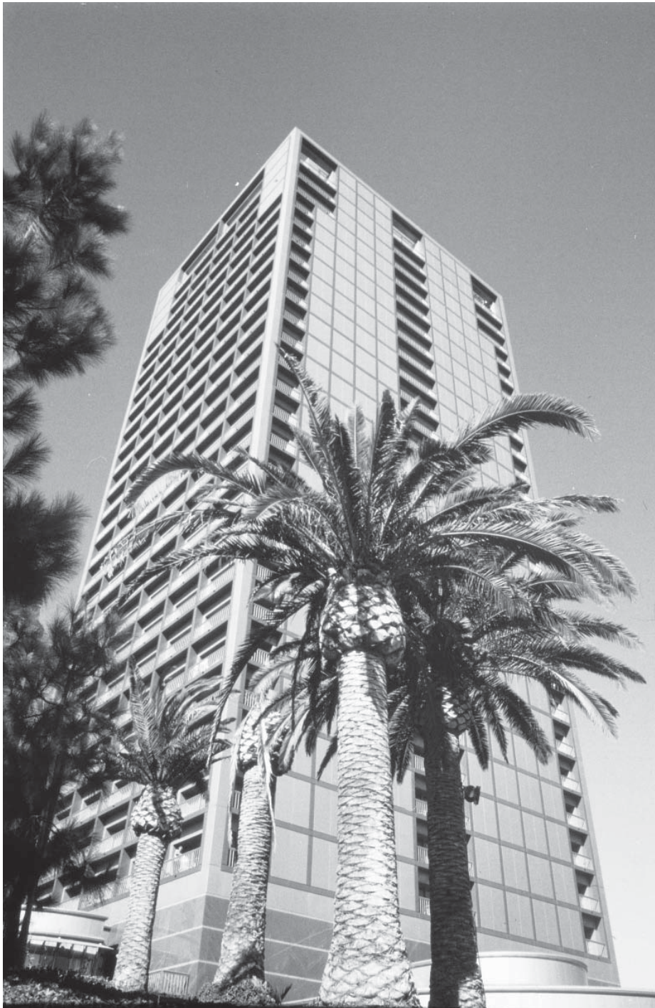
View of tower addition from ground, c. 1980s. (Source: Courtesy Westin Hotels & Resorts, Image No. 656b280f39_2.1.)
