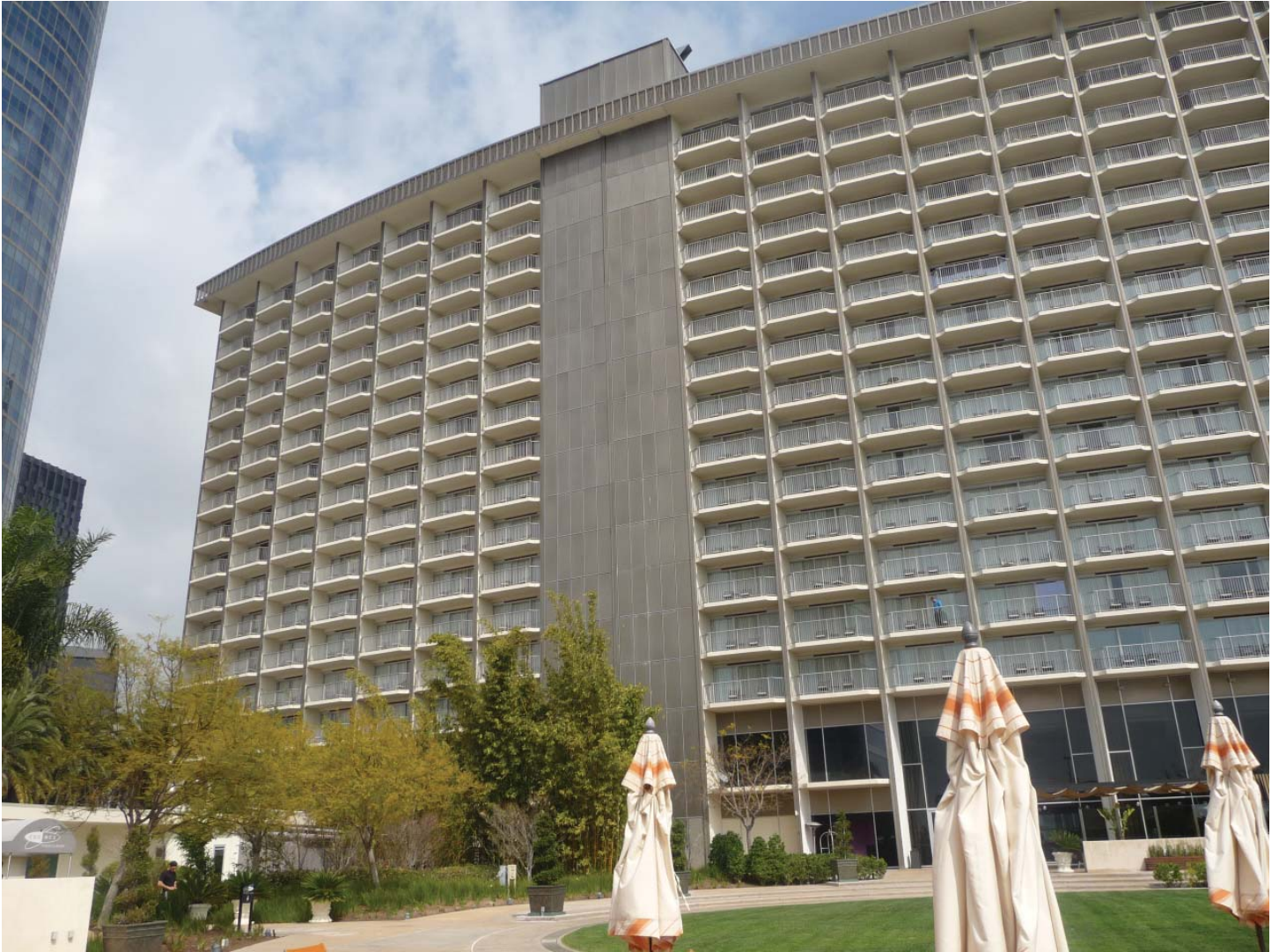
West facade, view looking northeast
