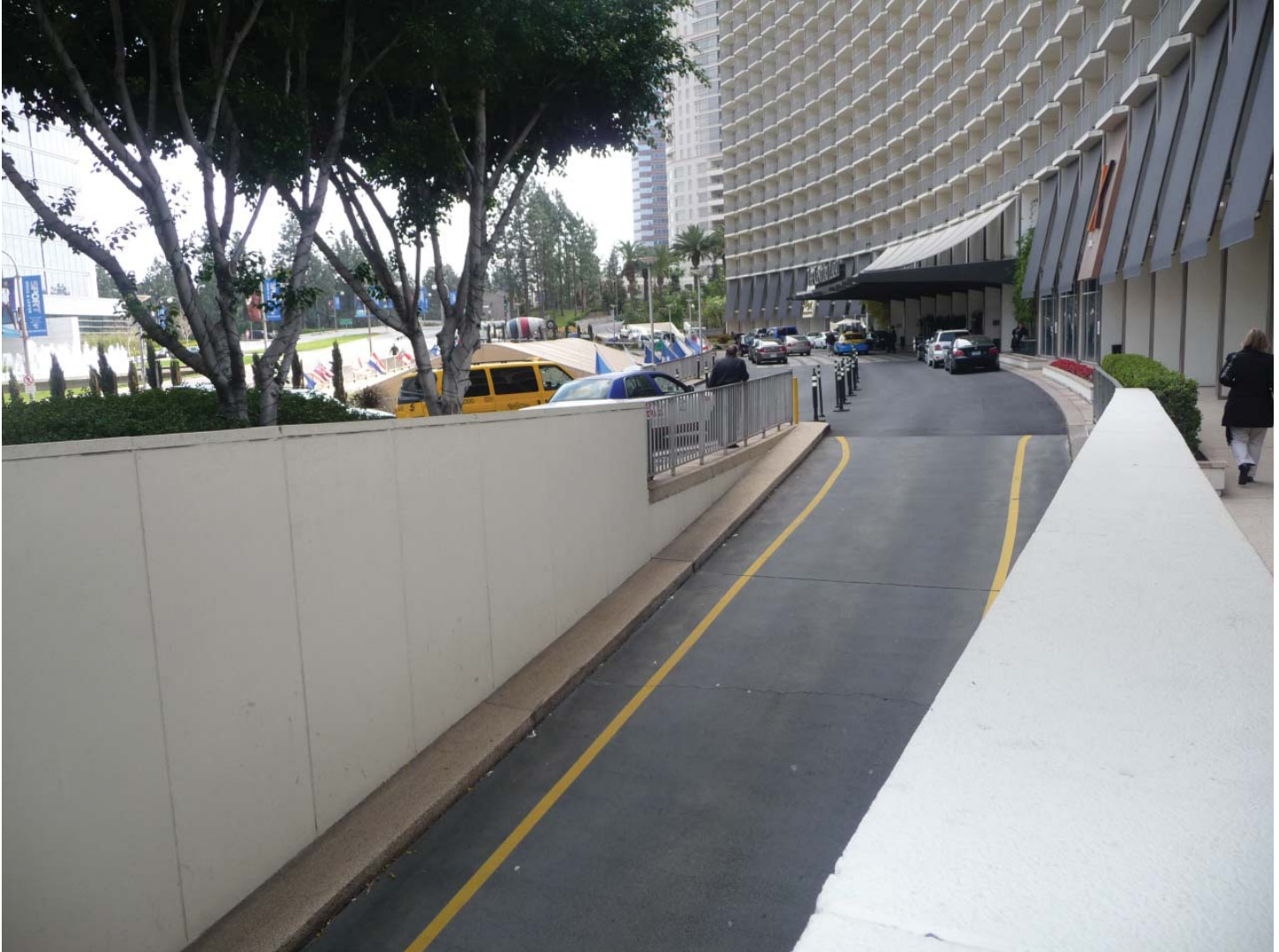
Driveway, main facade. View looking south
