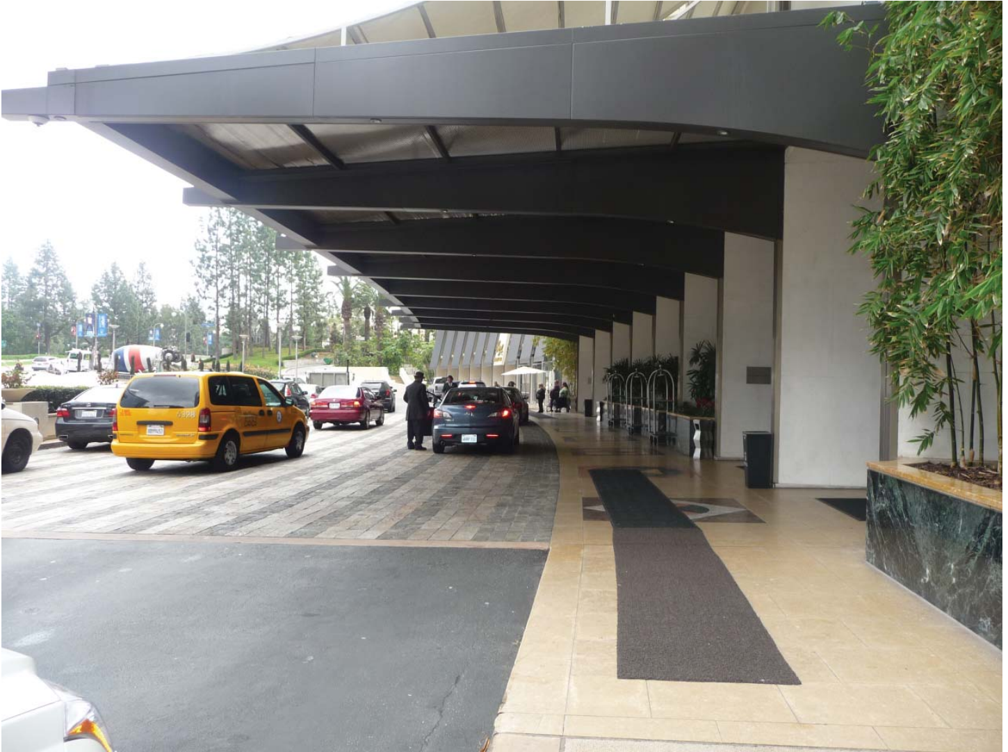
Detail canopy, main facade. View looking south
