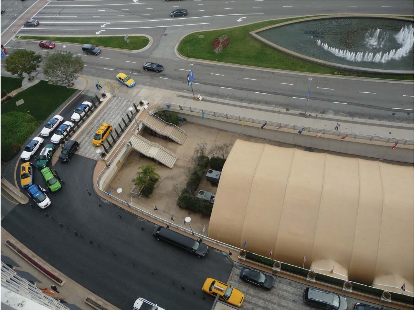
Driveway and sunken plaza, from upper balcony
