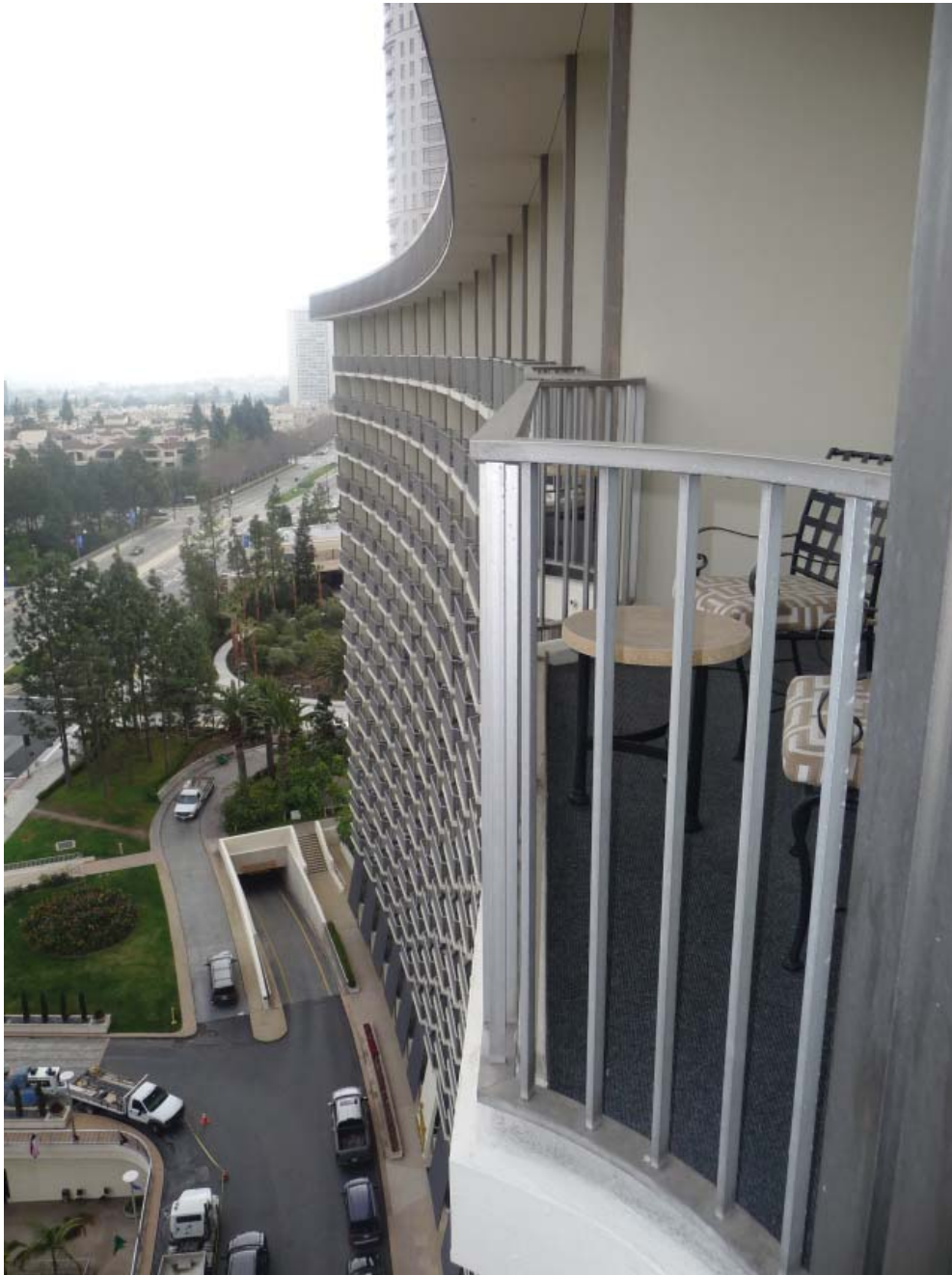
Facade detail from 19th floor balcony. View looking south.
