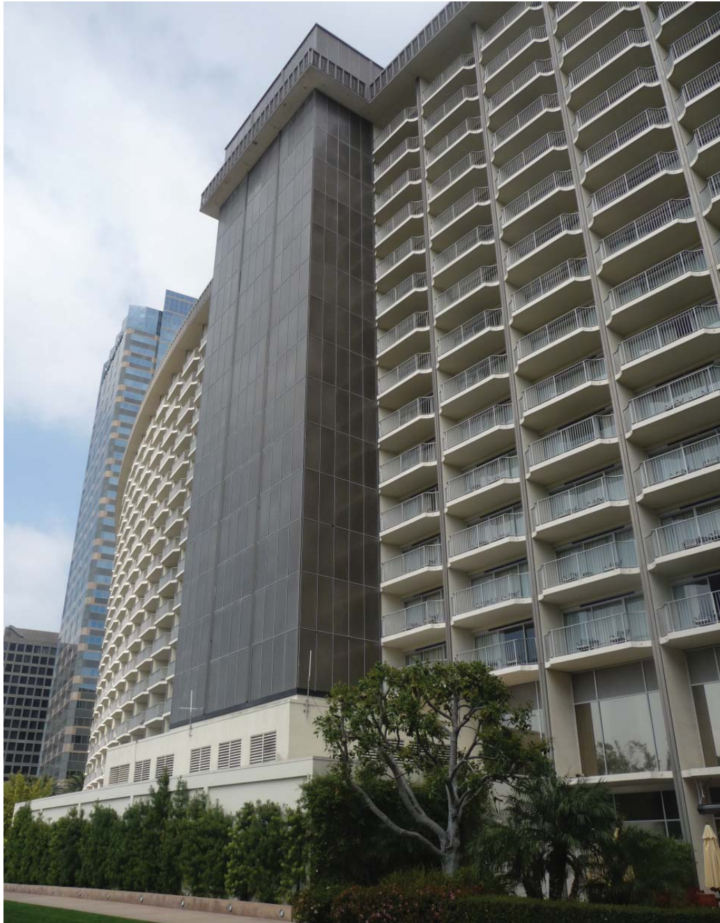
West facade detail, view looking northeast
