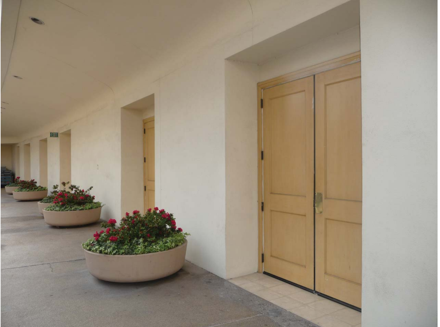
Sunken plaza, east-facing elevation detail
