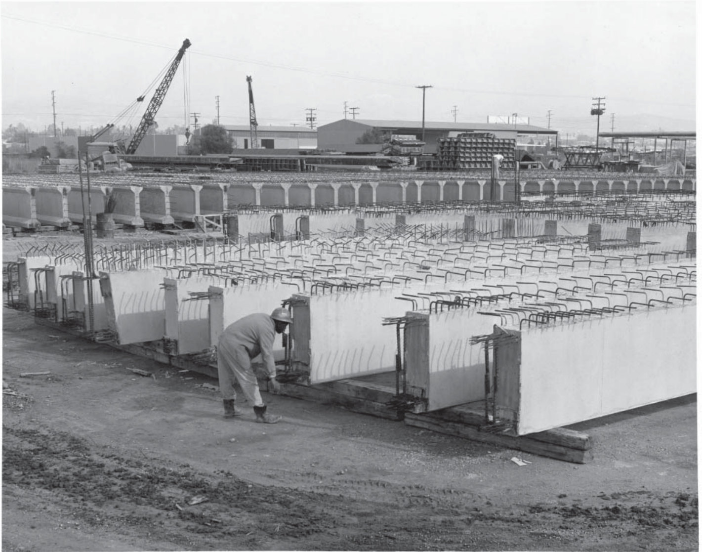
View of precast concrete building elements, c. 1965. (Source: Courtesy Westin Hotels & Resorts, Image No. 656b291f69_22.)
