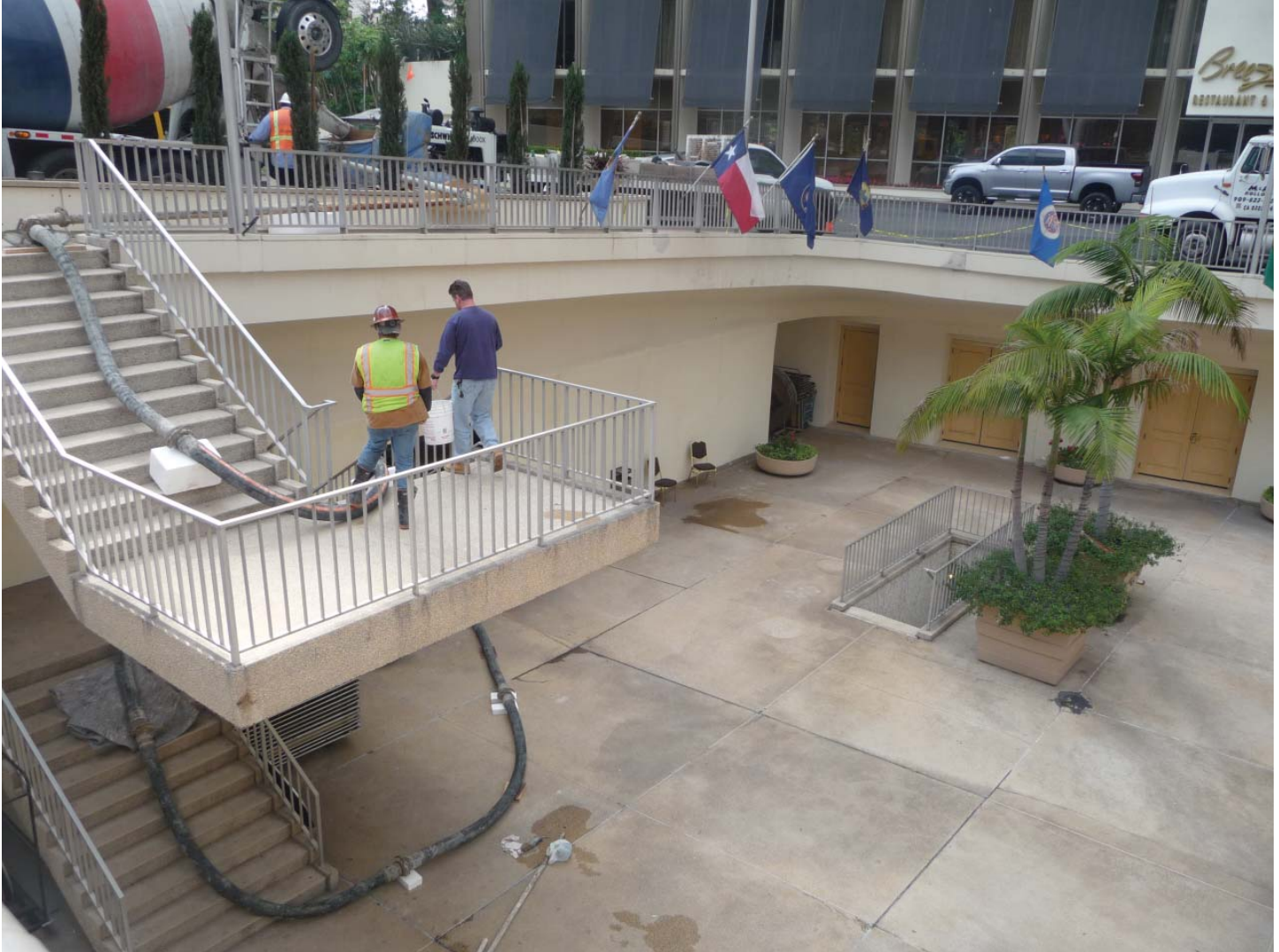
Sunken plaza, north- and east-facing elevations
