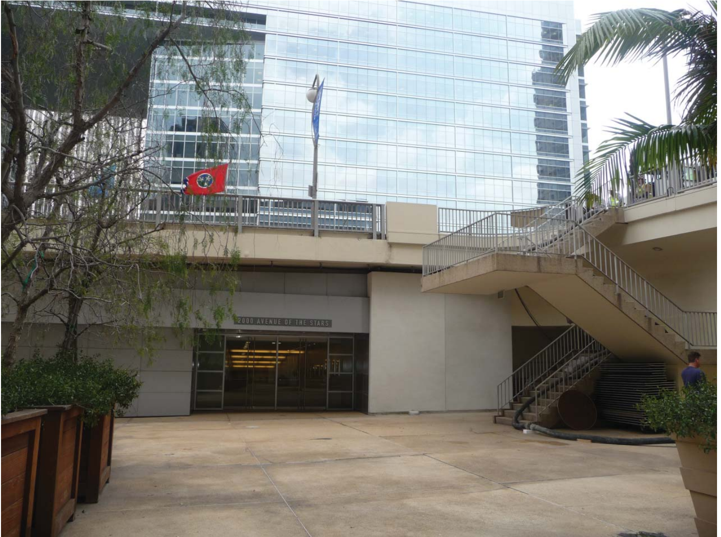
Sunken plaza, entrance to subterranean tunnel. West-facing elevation, view looking east
