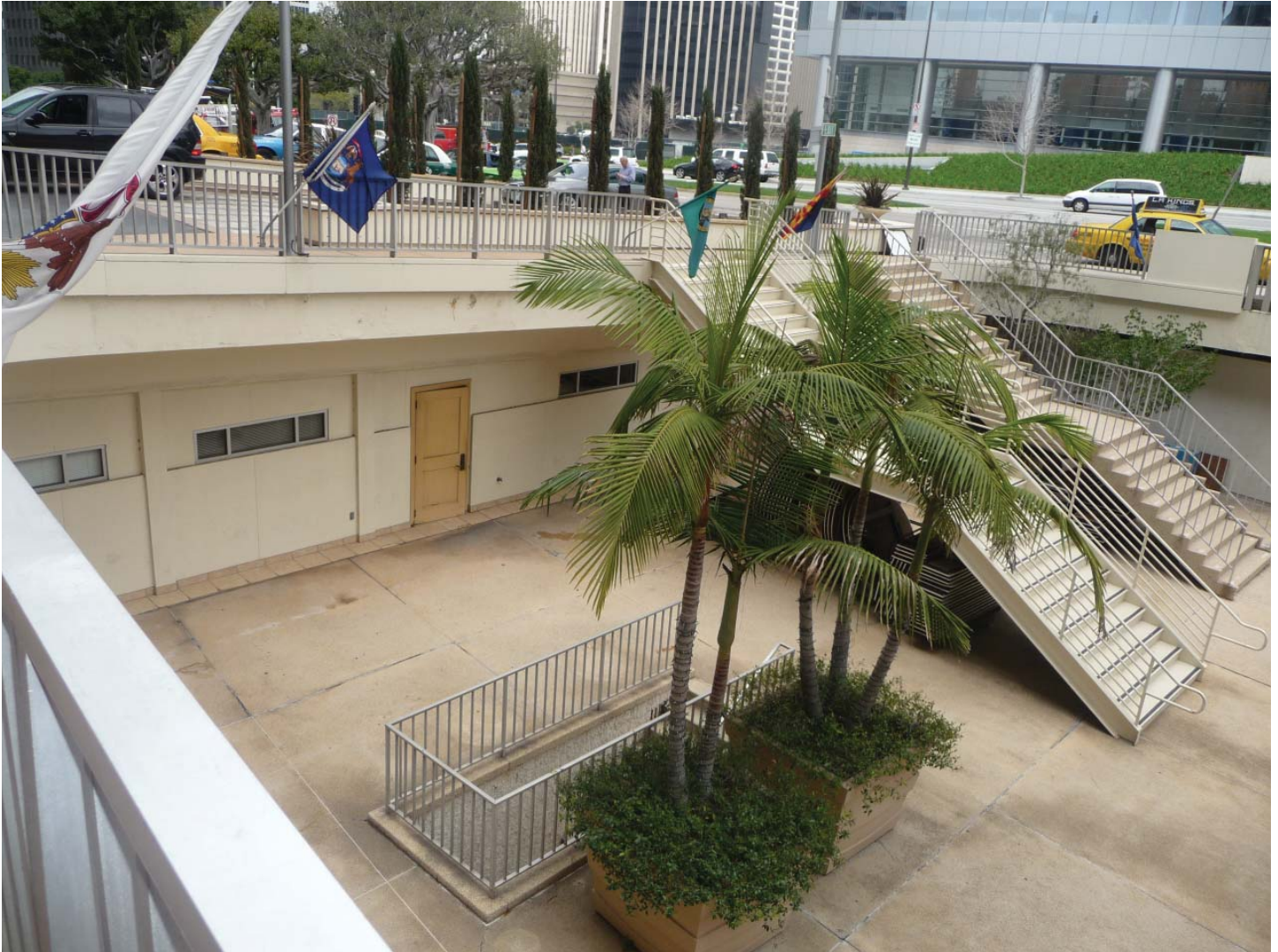
Sunken plaza, south-facing elevation
