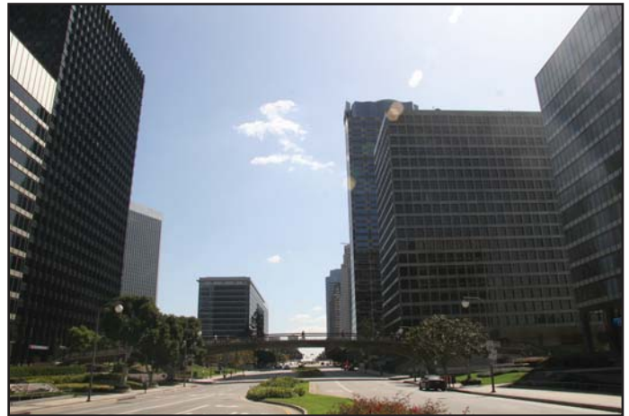
Photograph 16: Southeastern view along Avenue of the Stars toward the pedestrian bridge that crosses Avenue of the Stars and the 2000 Avenue of the Stars building.
