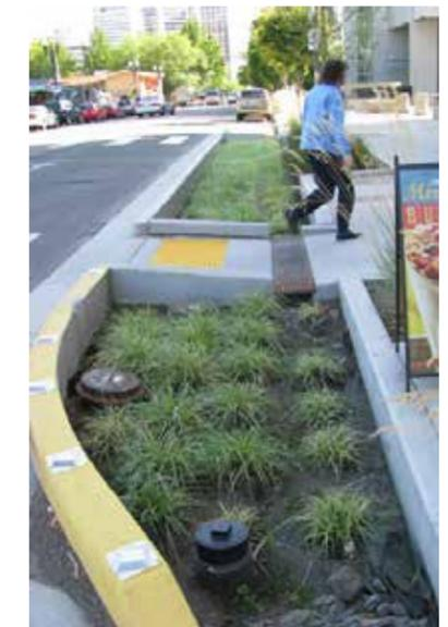
These curb extensions at street level with curbs collect and infiltrate street runoff. The excess runoff in the above right example flows into the storm drain system through a raised drain.
