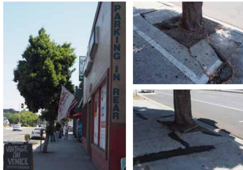
As these photos show, some already small tree wells have been filled with asphalt. Because the tree wells are so small, concrete is sometimes uplifted.
