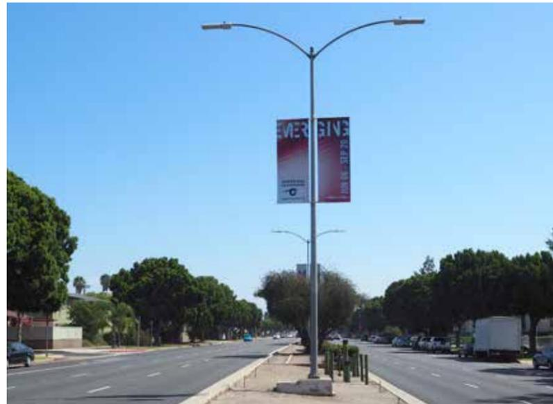
Street lights to illuminate the roadway are located in the median, except at intersections where they are on the sidewalks.
