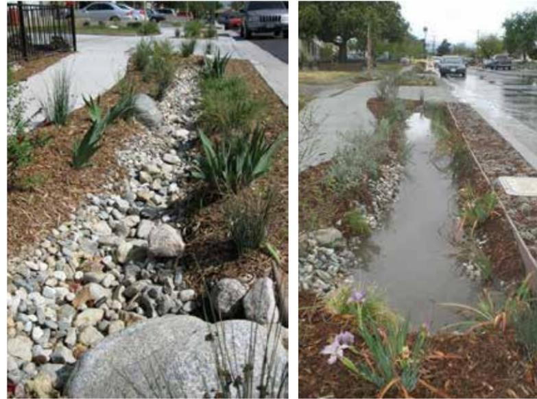
1. Parkway at sidewalk level with a swale or depression to collect and infiltrate sidewalk runoff. This example on Elmer Avenue in Sun Valley also infiltrates street runoff. (photo source: Council for Watershed Health)
