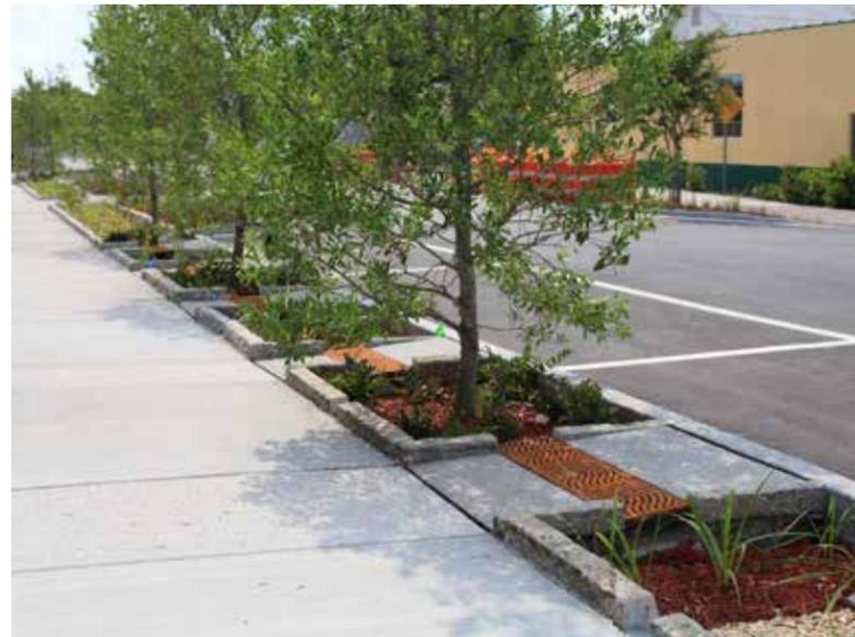
2. Tree wells at sidewalk with depressed soil level and curb breaks to collect street runoff are connected to function as a continuous infiltration basin. Curbs are often required where the soil level is lower than the sidewalk, as shown here. Overflow is released back into the street at the end of the connected tree wells. (photo source: Blue-Green Building.org)
