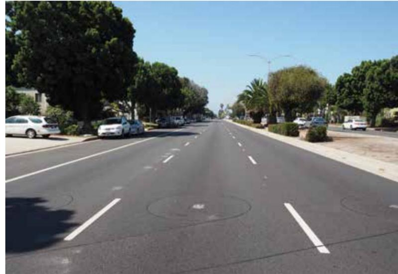
The roadway cross section is consistent from Beethoven Street to Inglewood Boulevard: three lanes, a bike lane and on-street parking in each direction. This photo of the eastbound half of the street is looking west.
