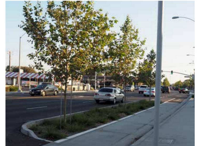
This street level parkway with a curb along the roadway on Rosemead Boulevard in Temple City separates the bike lane from traffic lanes. Street runoff flows from the street into the parkway through openings in the curb. Runoff that is not infiltrated flows across the bike lane into the gutter.
