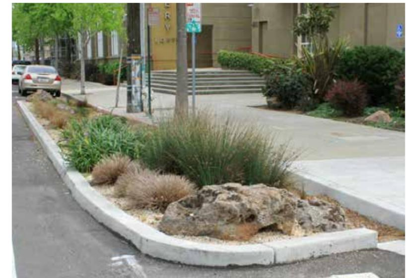
4. Curb extensions at street level with curbs. In this example runoff flowing along the gutter is directed into the curb extension swale where it can be absorbed into an "infiltration gallery" beneath the surface; in a heavy rain, excess runoff flows back into the gutter and into the existing storm drain system. (photo source: land8.com)
