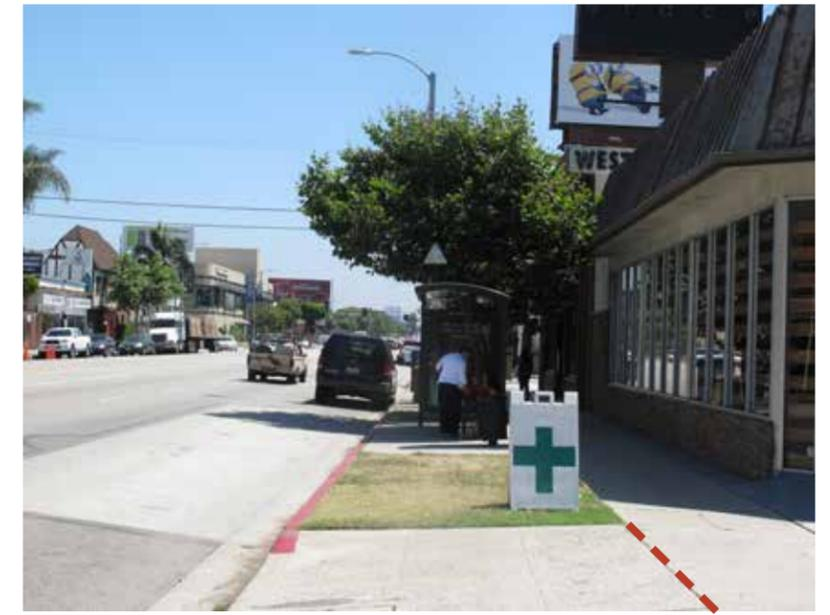
Where the sidewalk is at least 11' wide and the parkway is at least 5.5' wide, the sloped area of the driveway can align with the parkway. In this portion of Pico Blvd., the sidewalk is 15' wide and the parkway is wider than 5.5', so the slope of the driveway can be less than 10%.
