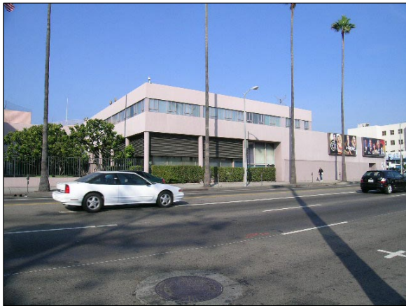
Television Building, South Façade
