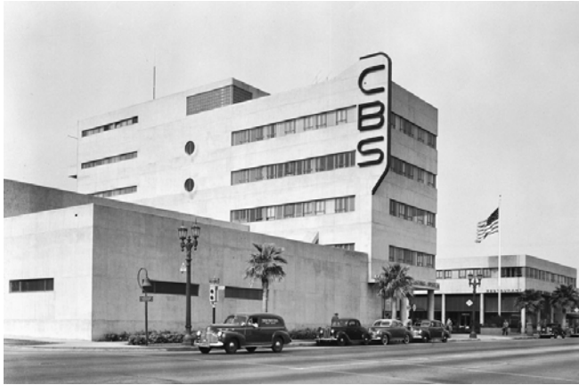
Figure 1: CBS Columbia Square looking NE
