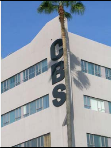
Detail of Sign, South Façade Radio Building
