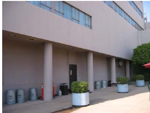
Figure 42: Detail of Radio Building, 2006
