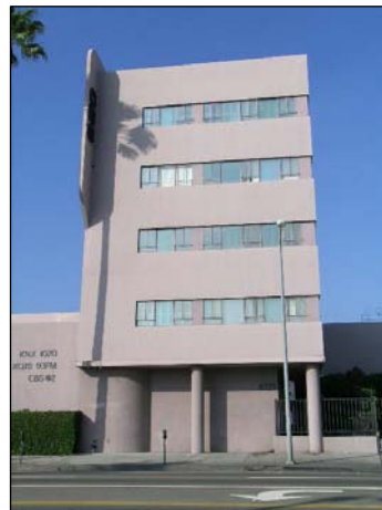
Radio Building, South Façade
