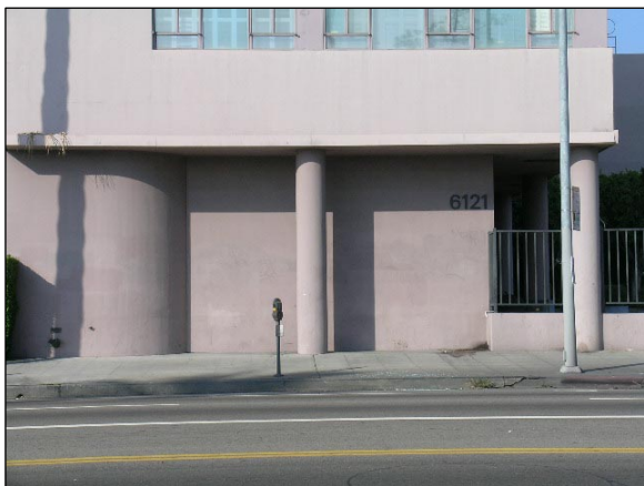
Detail, Radio Building South Façade
