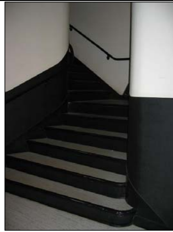
Radio Building Stair
