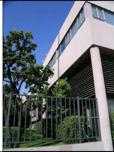
Detail, Television Building West Façade
