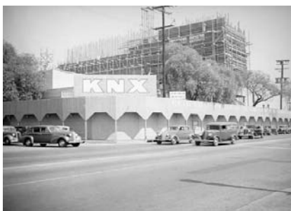
Figure 8: CBS Columbia Square during construction, c. 1937
