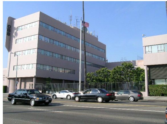
Figure 34: Columbia Square Complex, 2006
