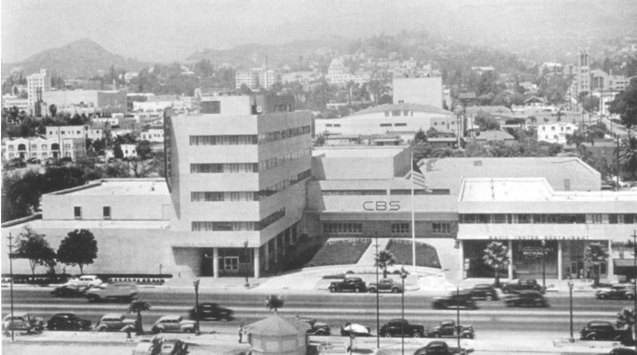
Figure 24: CBS Columbia Square Complex c. 1940 showing the Lescaze and Parkinson & Parkinson components
