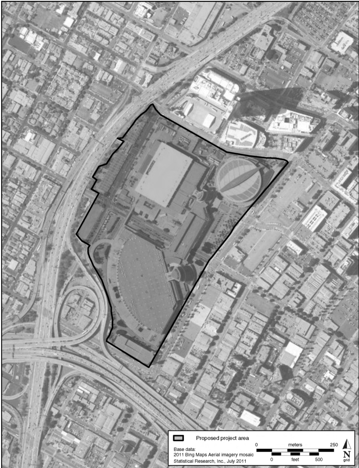
Figure 1.3. Aerial photograph of the existing Proposed Project site.
