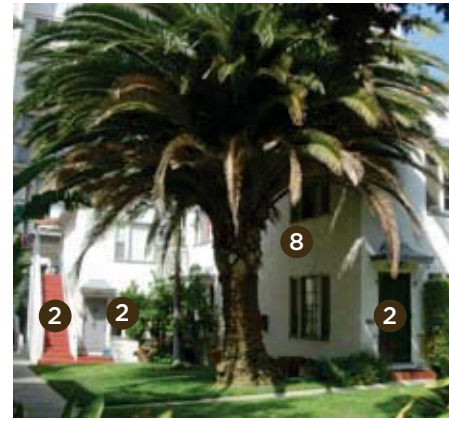
Figure 3-51 Materials and Colors in the Franklin Avenue Design District
