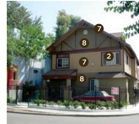
Figure 3-52 Materials and Colors in the Franklin Avenue Design District
