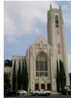
Figure 3-15 10. Hollywood Methodist Church
