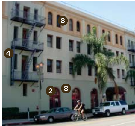
Figure 3-50 Materials and Colors in the Franklin Avenue Design District
