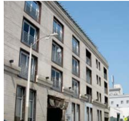
Figure 3-54 Balconies Within the Hollywood Boulevard District
