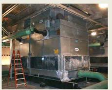
Evaporative Condenser (note scale buildup on front right)
