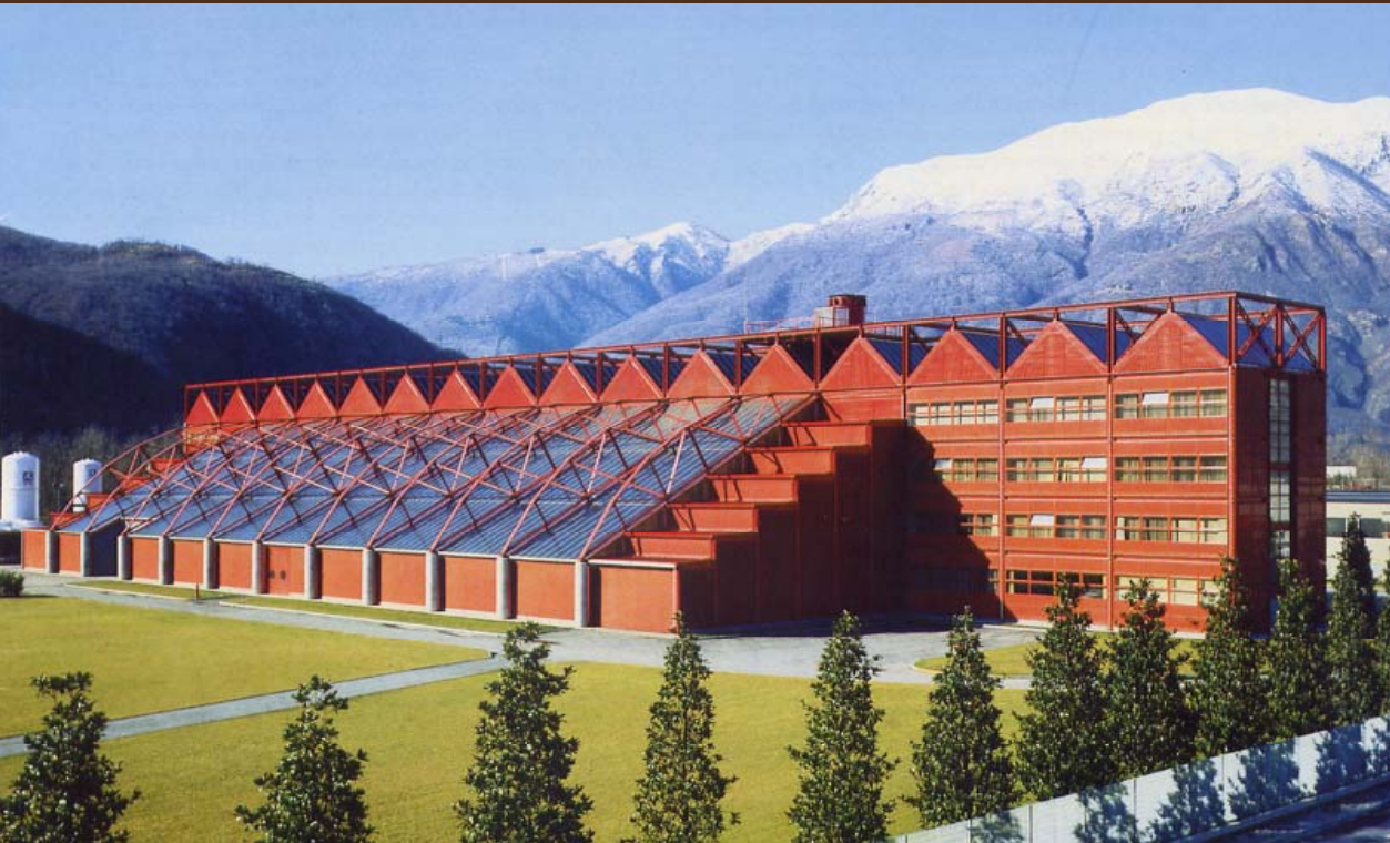
Gasification Plants (Germany)
