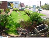
through infiltration and evapotranspiration. Swales are most effective where longitudinal slopes are small (two to six percent), increasing the residence time for treatment, and where water depths are less than the vegetation height.
