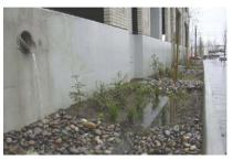
infiltrate through the planter soil matrix and into the ground. Flow-through planters include the use of a waterproof lining and underdrain. Both types of planter boxes require an overflow to an approved stormwater conveyance system and may be used to help fulfill site landscaping requirements.
