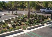
for adequate time for infiltration and pollutant adsorption and uptake. During large storms, a portion of runoff is diverted past the facility to the storm drain system. Depending on location and site constraints, bioretention systems can be designed with and without perforated
