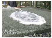
not release harmful chemicals into the environment. It has been in use throughout Europe for about fifty years. A domestic formula known as the Portland Cement Pervious Pavement has been used successfully since the 1970s in the U.S. The pavement is a special blend of Portland cement, sand-free coarse aggregate, and water.
