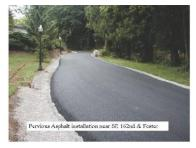
designed to temporarily store the volume of stormwater generated from a design storm and infiltrate it into underlying soils or into an underdrain system. Similar to pervious concrete designs, pervious asphalt mix pavements have been used in parking lots, private streets, driveways, and pedestrian access areas since the 1970s.
