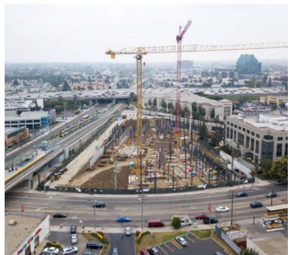
Construction adjacent to the active ROW may require ongoing coordination with Metro.
