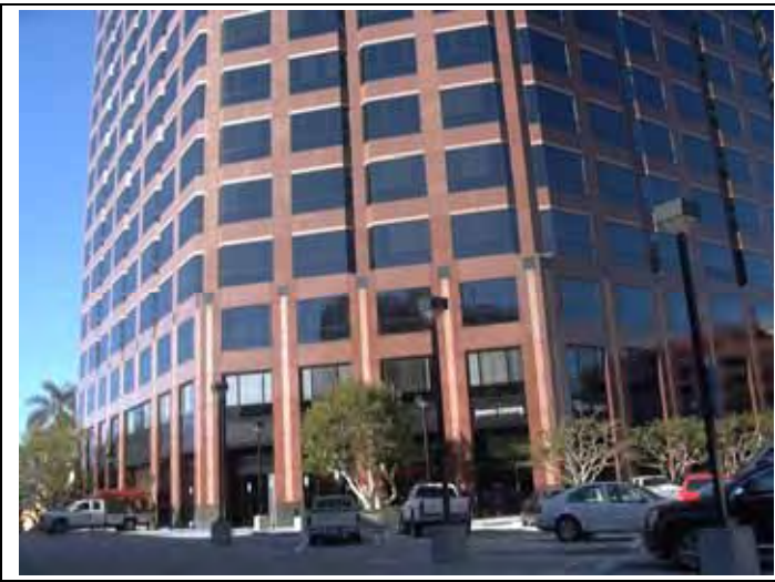
1. View of south side of the subject property office building.
