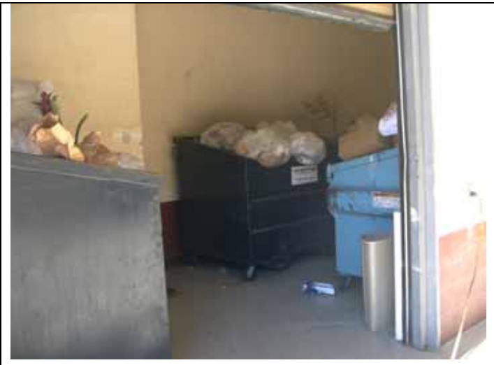
3. View of dumpster area on the ground floor, southwest portion of the office building.
