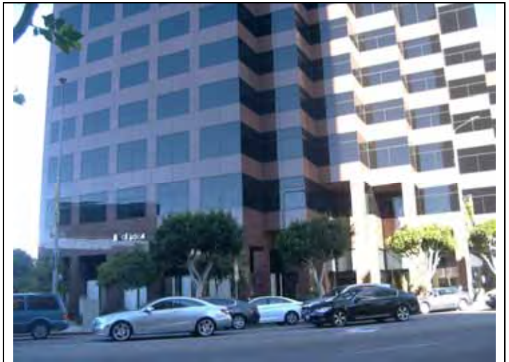
6. View of west side of the office building.
