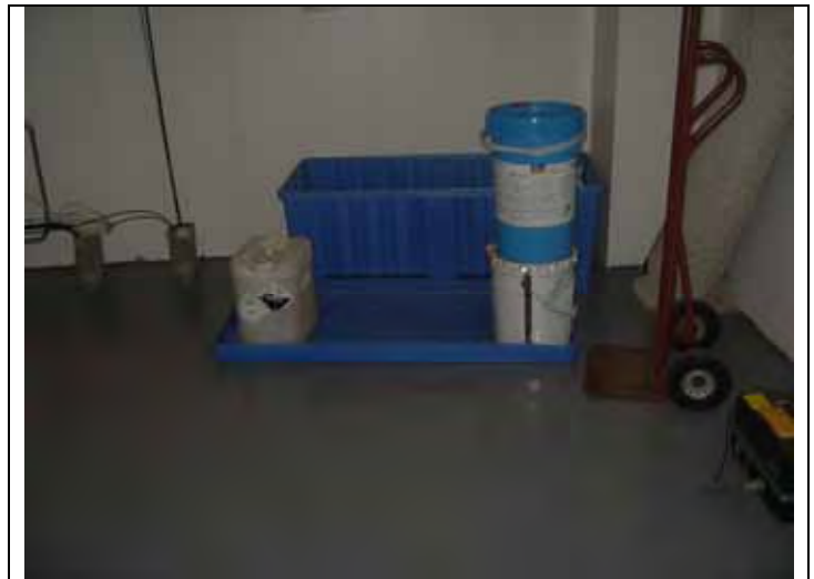
18. View of water treatment chemicals at the subject property.
