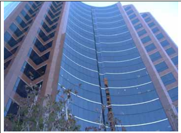
5. View of north side of the office building.
