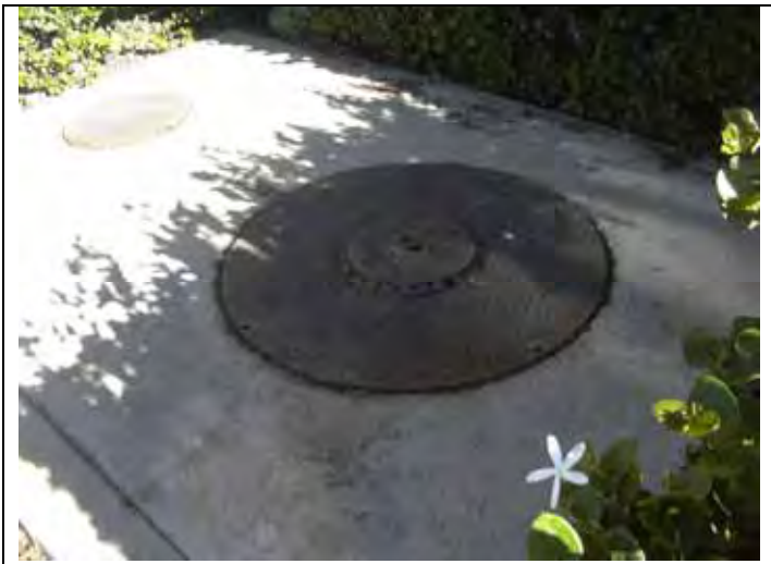
9. View of diesel UST location on the northwest portion of the retail building.
