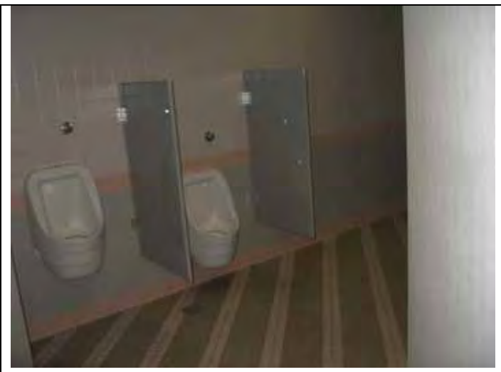
15. View of a restroom inside the office building.
