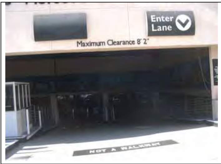
7. View of entrance to the subterranean parking garage.
