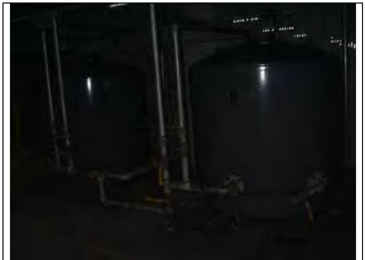
24. View of de-watering filtration system at subterranean parking garage P4.
