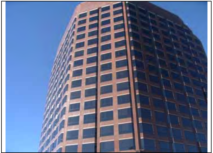
2. View of office building at the subject property.
